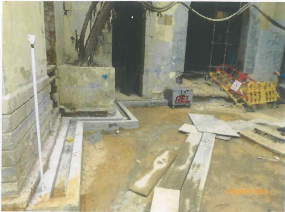
Fig. 8 The site near Tree 11 is under renovation.
