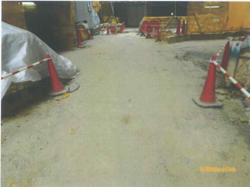
Fig. 11 The site outside the cordon zone appears clean and tidy.
