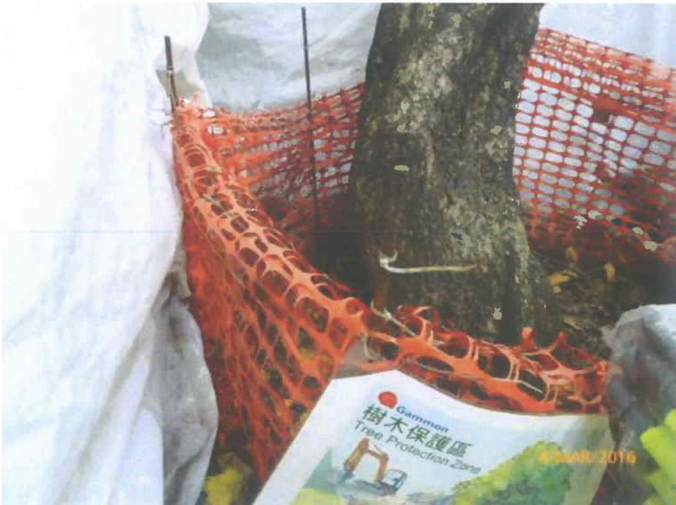
Fig. 7 The small cordon zone is in order.
