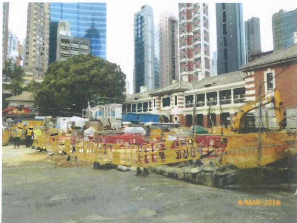
Fig. 13 Construction works are in progress outside the cordon zone.
