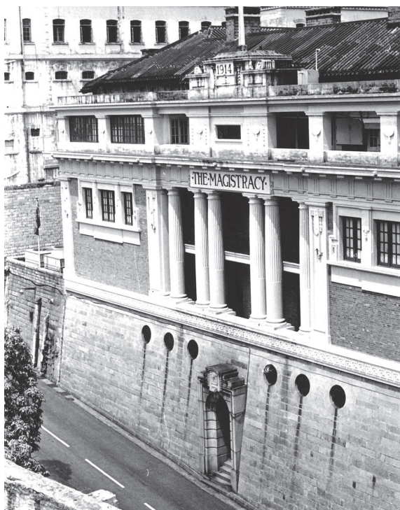
Front (east) elevation of the Magistracy on Arbutnot Road
