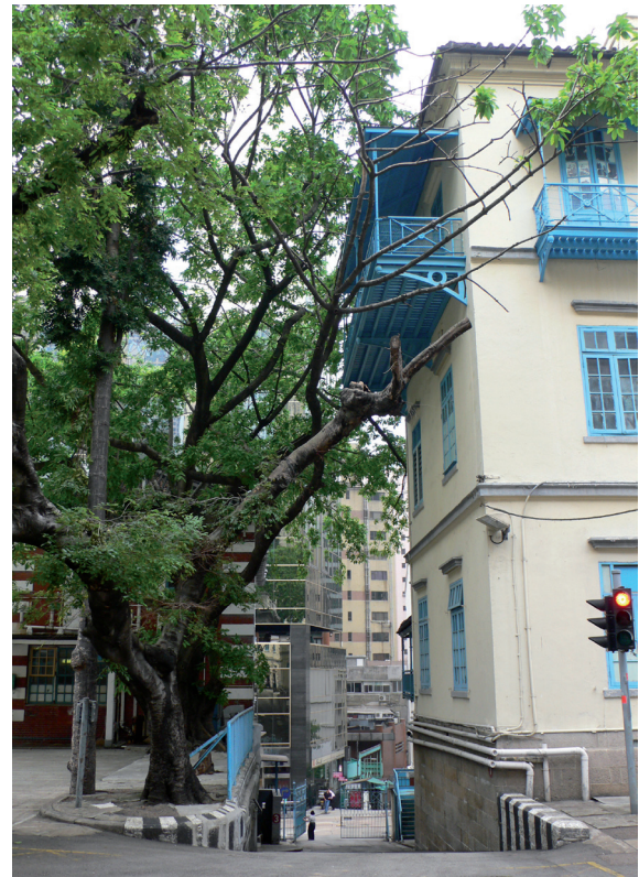
View of the main entrance ramp (Pottinger Street) from inside the site
