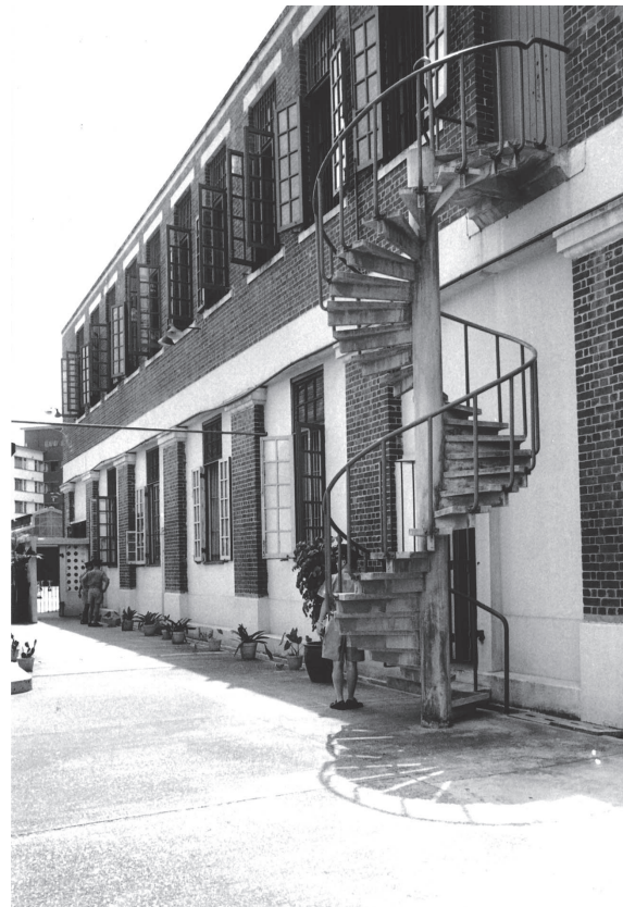
F Hall exterior
