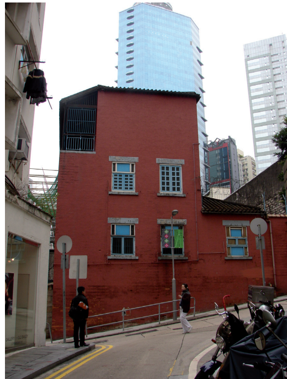
West façade of the Ablutions Block as viewed from Staunton Street
