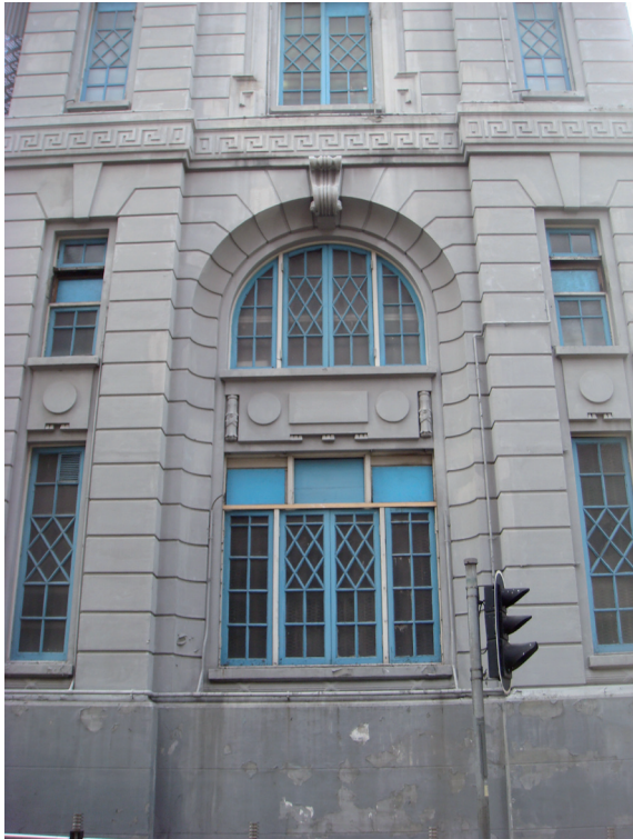
Detail view of the north façade on Hollywood Road
