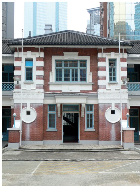
View of the central bay of the Headquarters Block showing brick and render similar to the Fringe Club.
