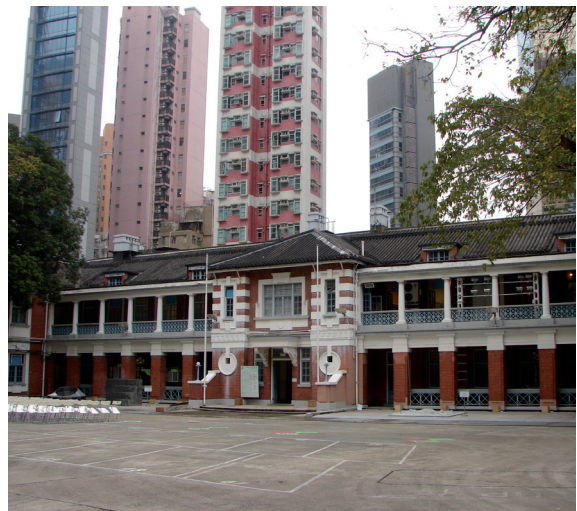
View of the south façade of the Headquarters Block facing the Parade Ground
