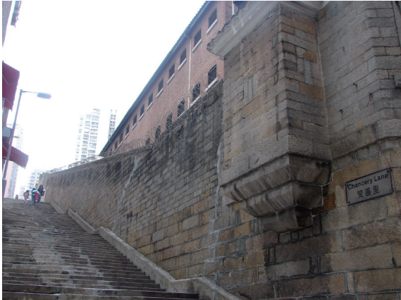
The historic steps on Chancery Lane
