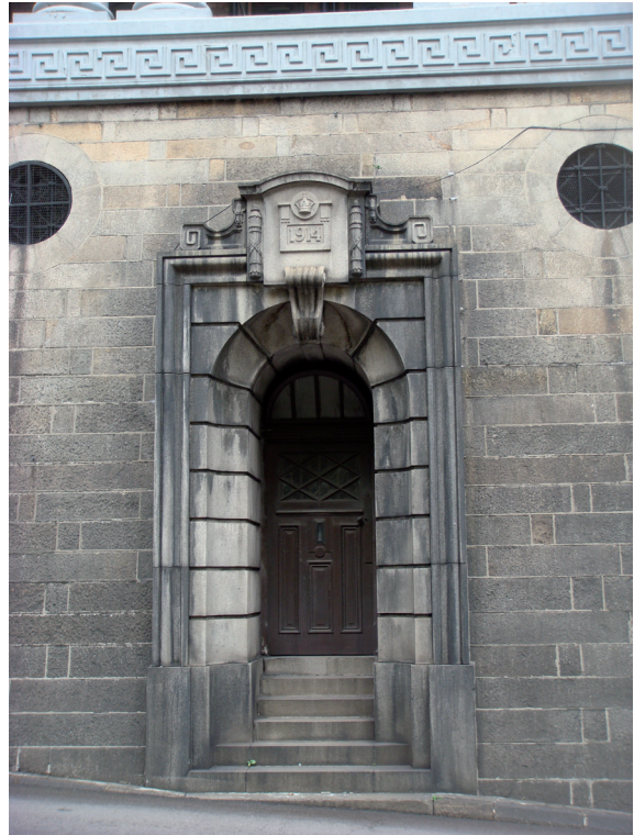
East Magistracy door at street level on Arbuthnot Road
