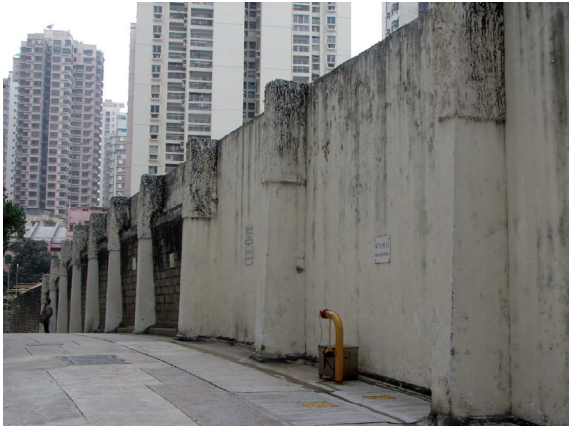
The security wall on Chancery Lane
