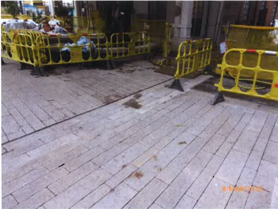
Fig. 10 The access near the planter appears clean and tidy.
