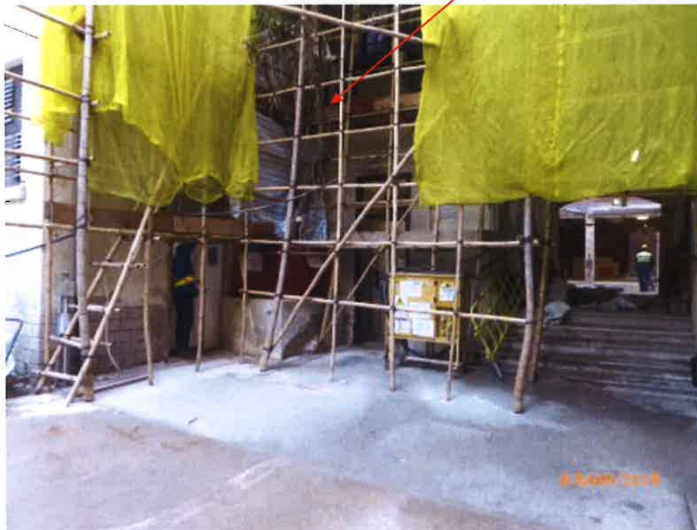
Fig. 10 Renovation works are in progress near Tree-11 .
