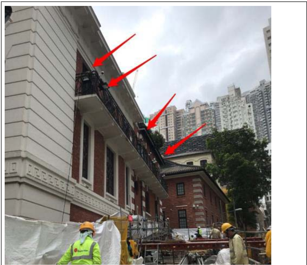
Photo 1: Four Light fittings on the external façade of Block 1 facing Old Bailey Street
