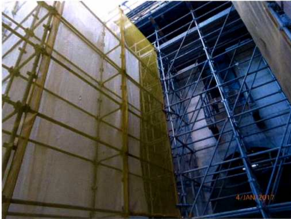
Fig. 10 Renovation works are in progress near Tree-11.
