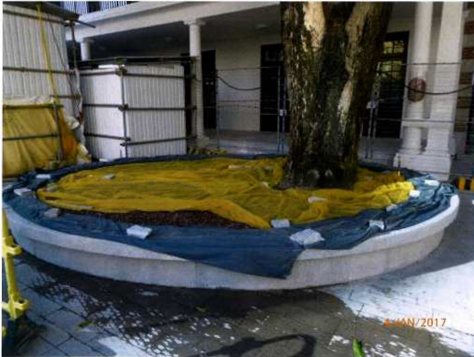
Fig. 10 The newly-built planter has been backfilled with top-soil in December 2016.
