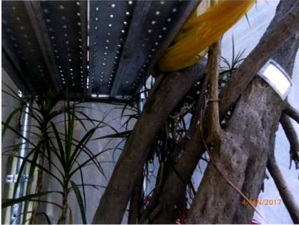
Fig. 8 The working platform still set up close to Tree-11.
