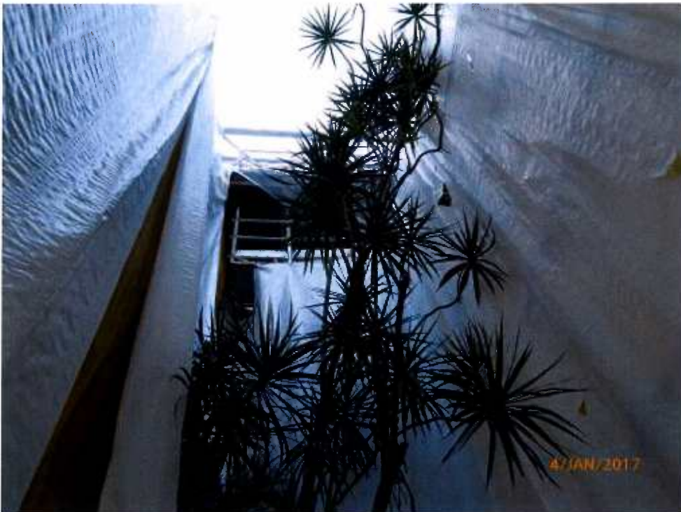
Fig. 9 A temporary shelter is erected to protect the tree.
