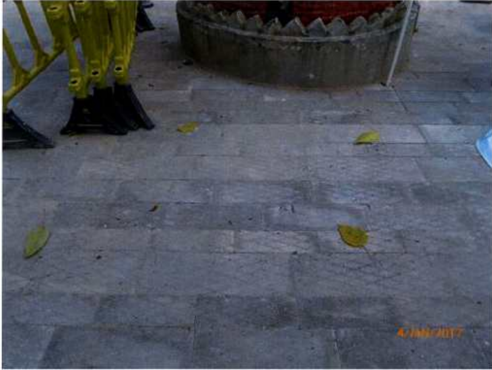
Fig. 10 The site near the planter is clean and tidy.
