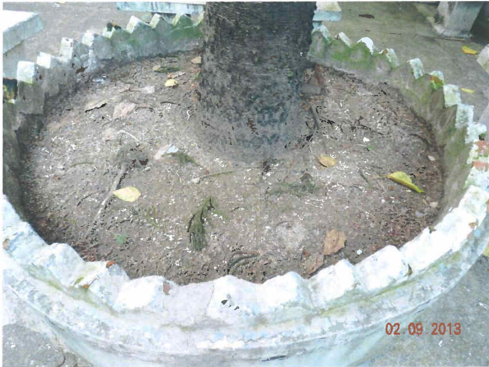
Fig 2. The planter and the site are clean and tidy at the time of inspection.
