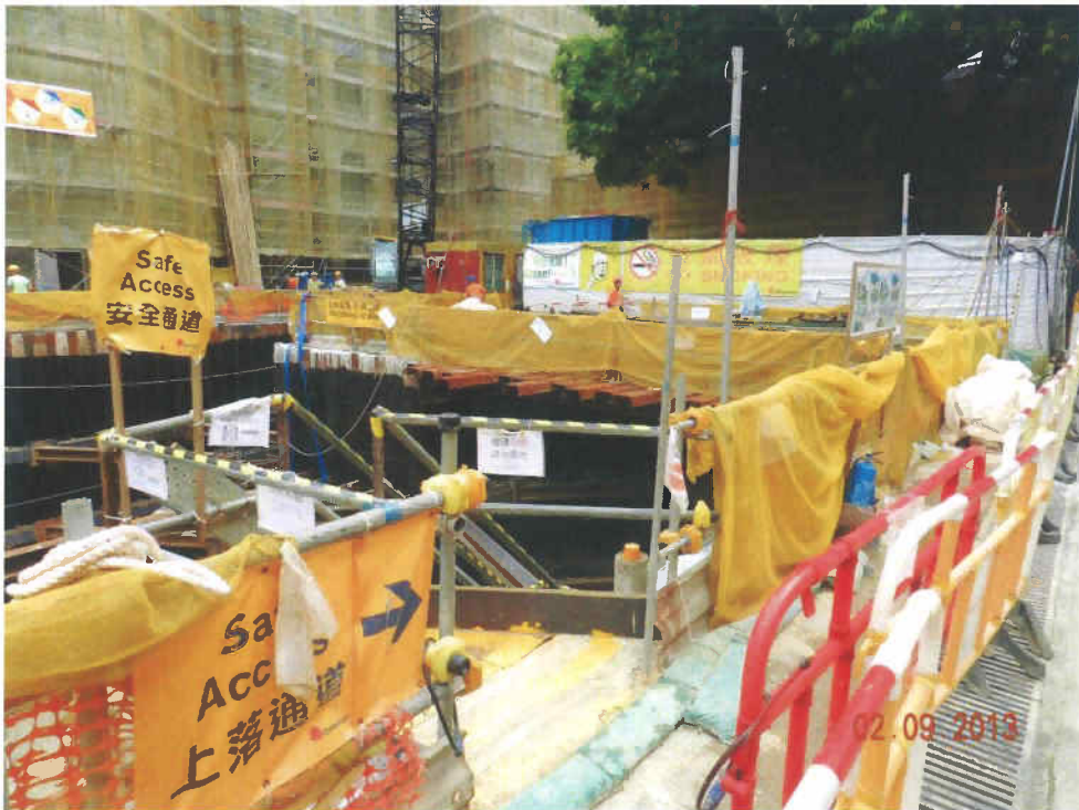
Fig. 7 Construction works are in progress outside the cordon zone.
