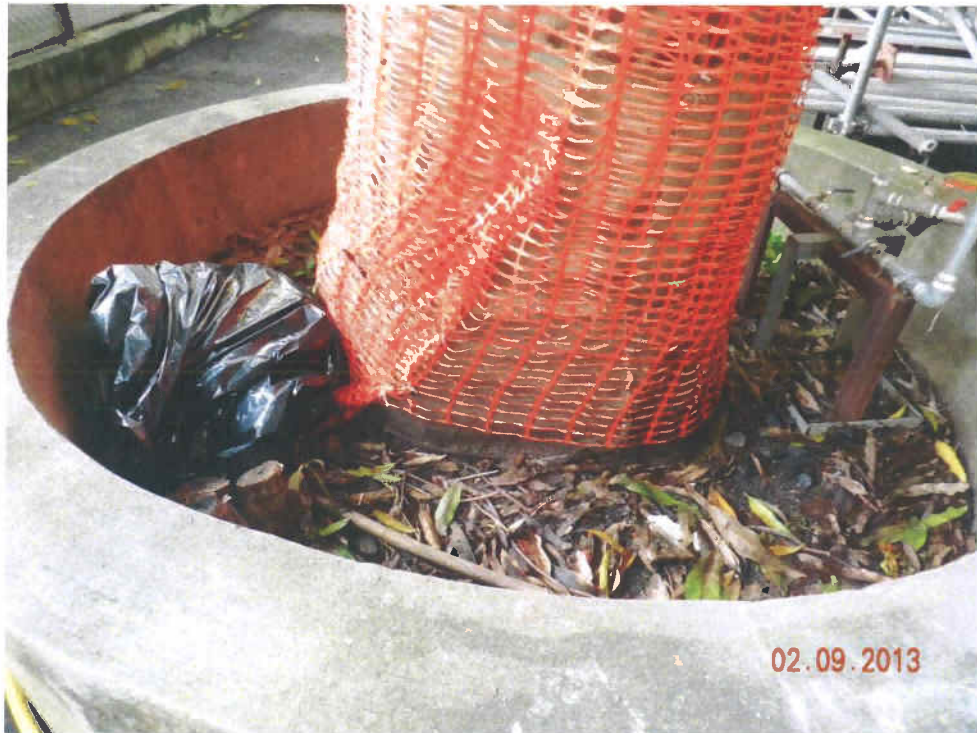
Fig 2. The planter is full of fallen leaves and cleansing tools. Cleanliness of the planter is not acceptable.
