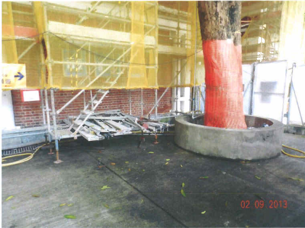
Fig. 4 A large scaffold set up near the tree for renovation work.
