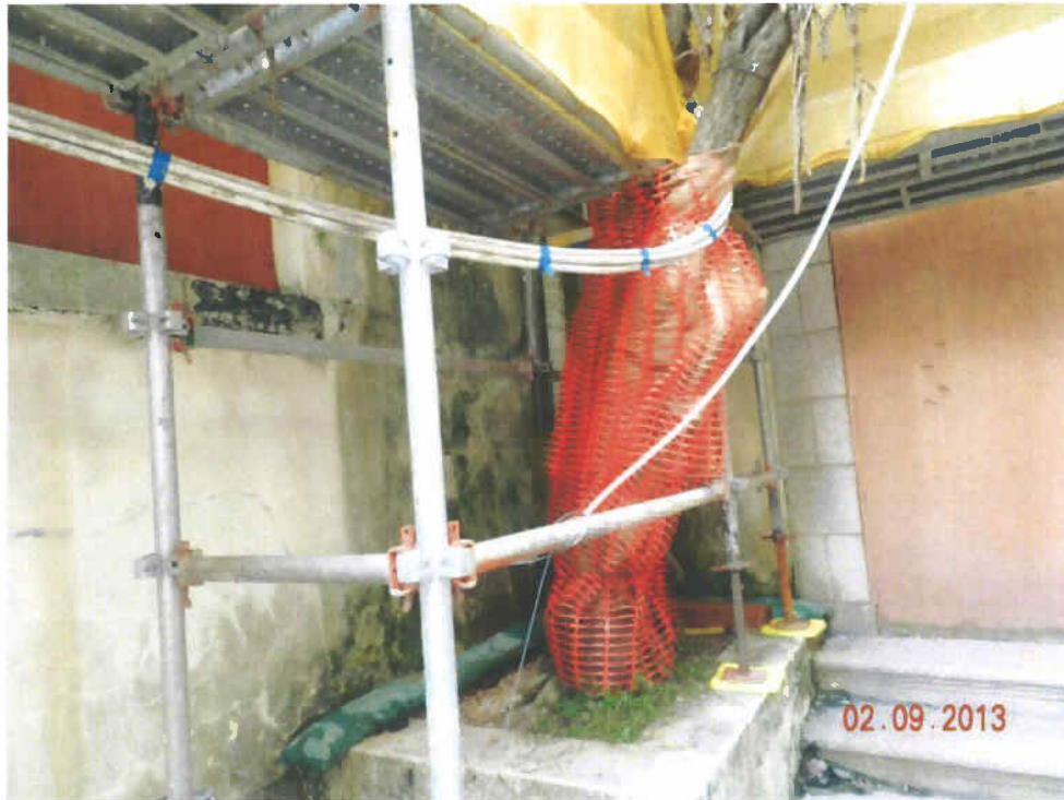
Fig. 4 A large scaffold set up near Tree-11. The tree has been wrapped with hessian cloth and reflex net so as to protect the trunk.
