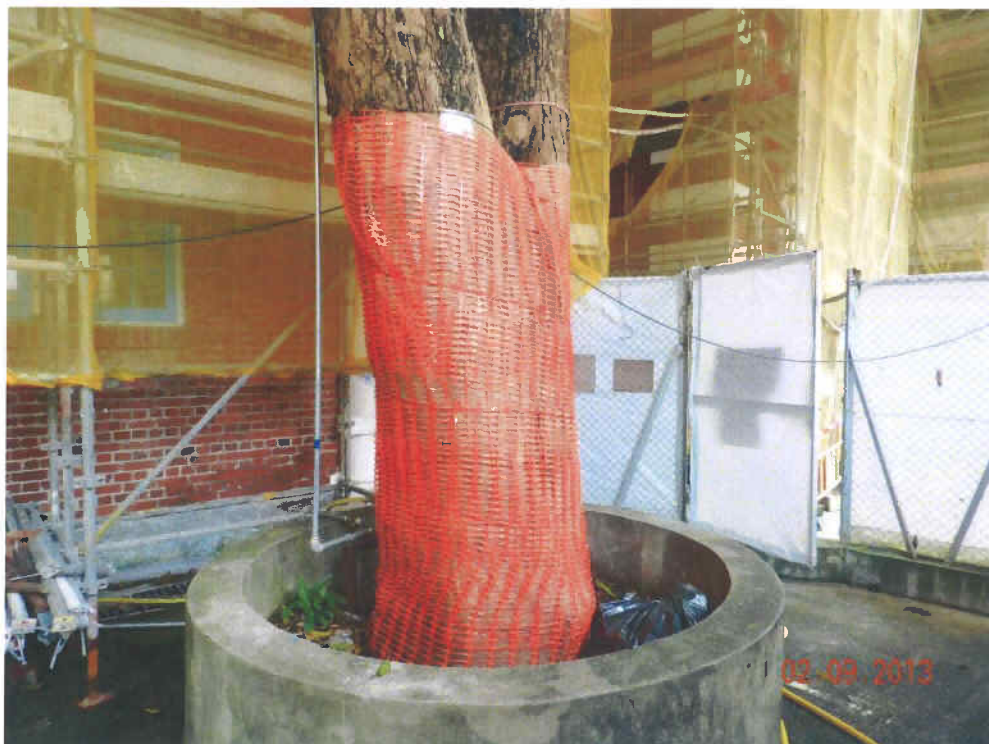
Fig. 3 The tree has been wrapped with hessian cloth and reflex net so as to protect the trunk.
