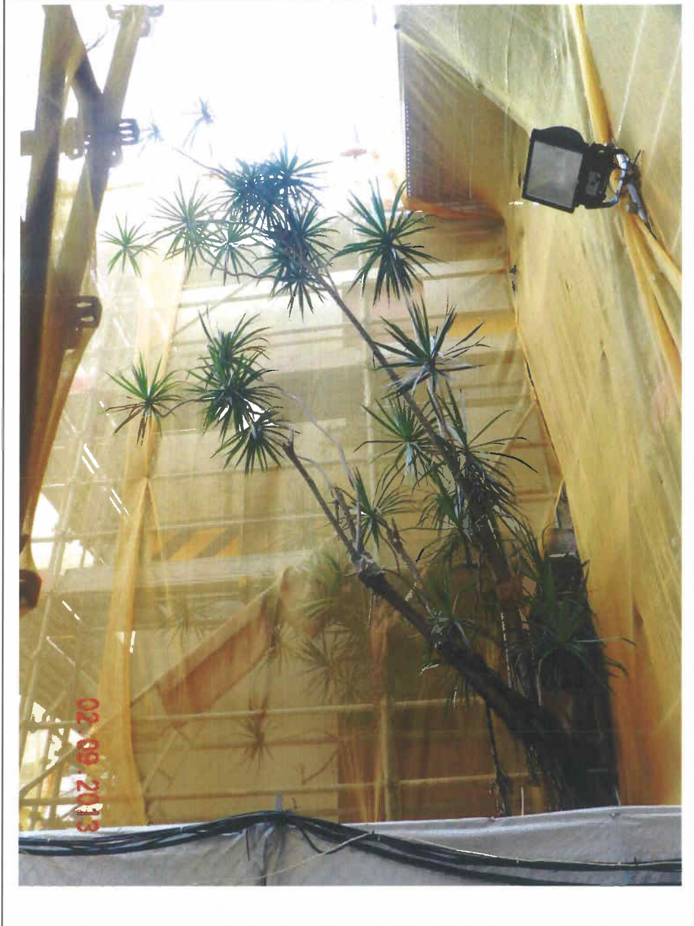
Fig. 8 Overall view of Tree-11 during inspection on 2 nd September 2013.
