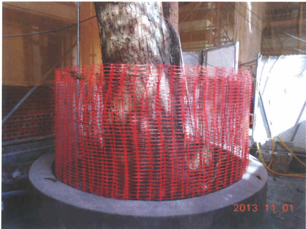
Fig. 5 A small cordon zone is set up round the planter to protect the tree.
