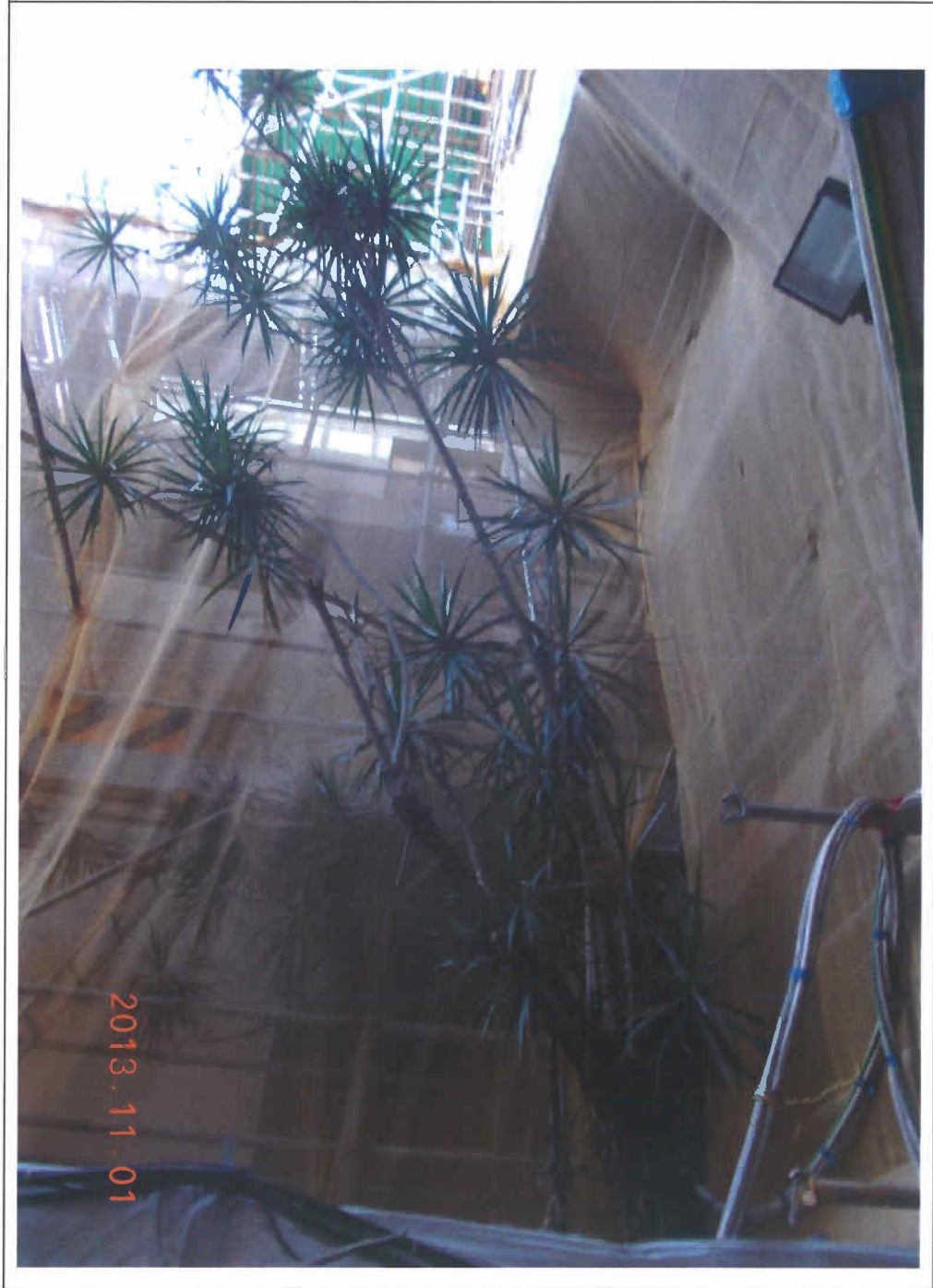
Fig. 8 Overall view of Tree-11 during inspection on 1 st November 2013.
