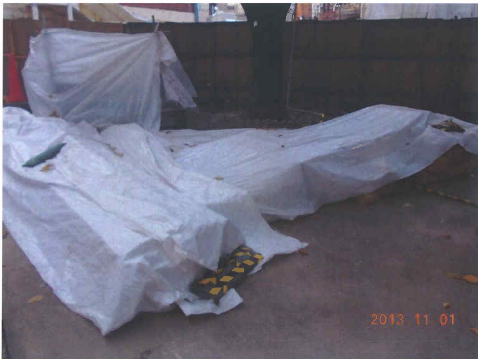
Fig. 3 Several heaps of construction materials are placed inside the cordon zone but cause no disturbance to the tree.
