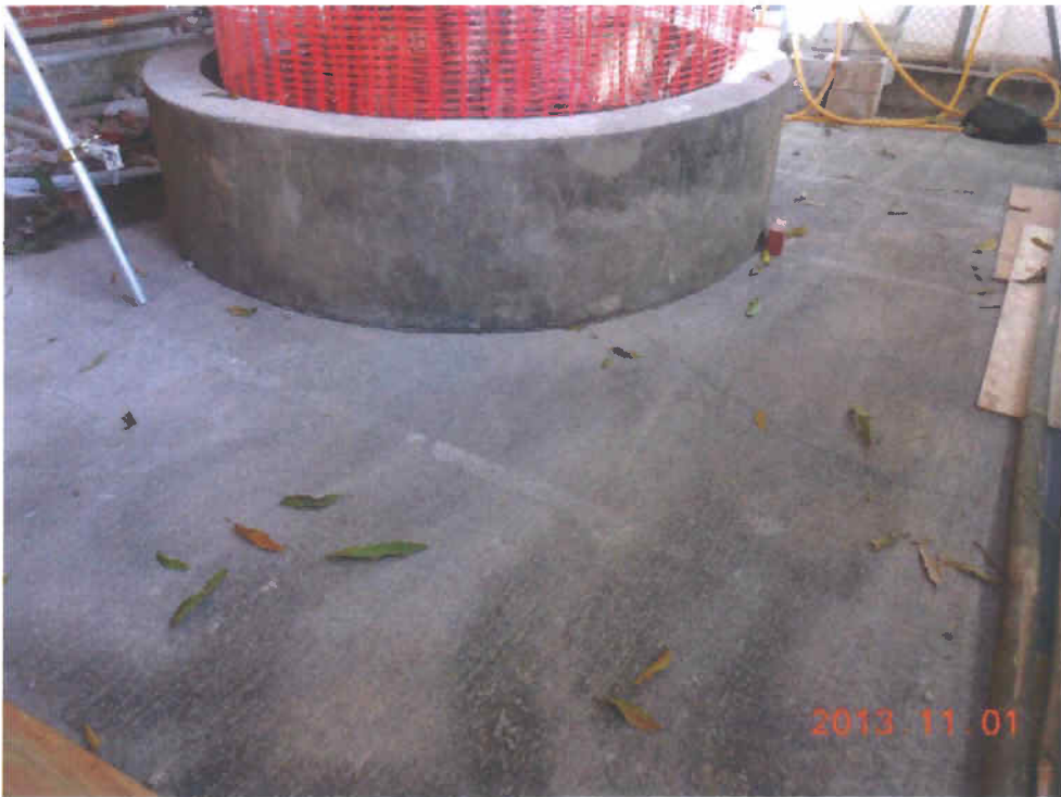
Fig. 3 Cleanliness of the site is acceptable..
