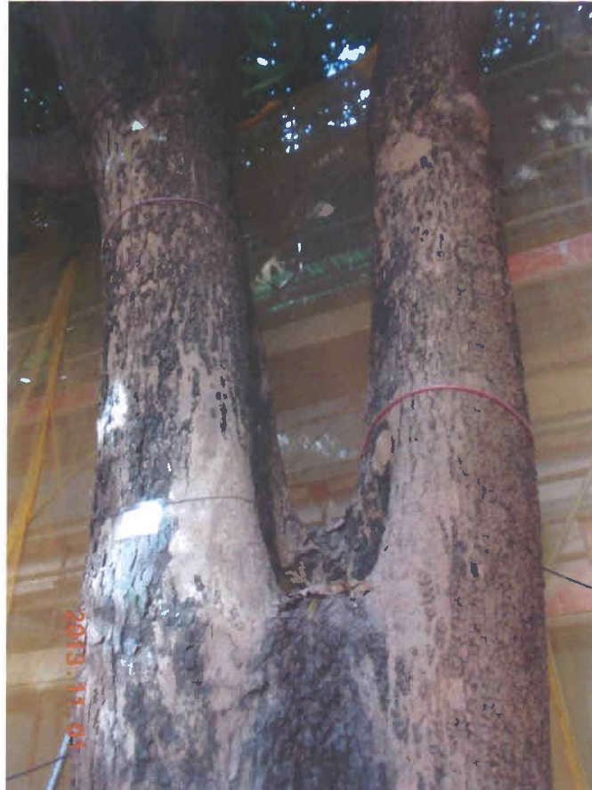
Fig. 6 The trunk is in good condition.
