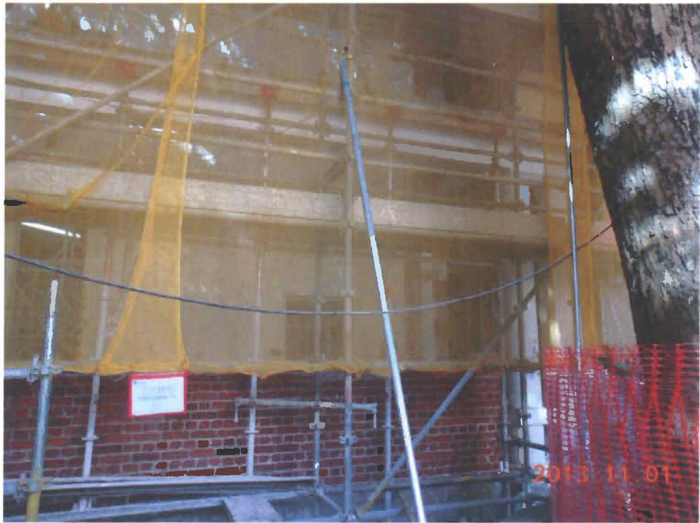
Fig. 4 The scaffold is still at site for renovation work.
