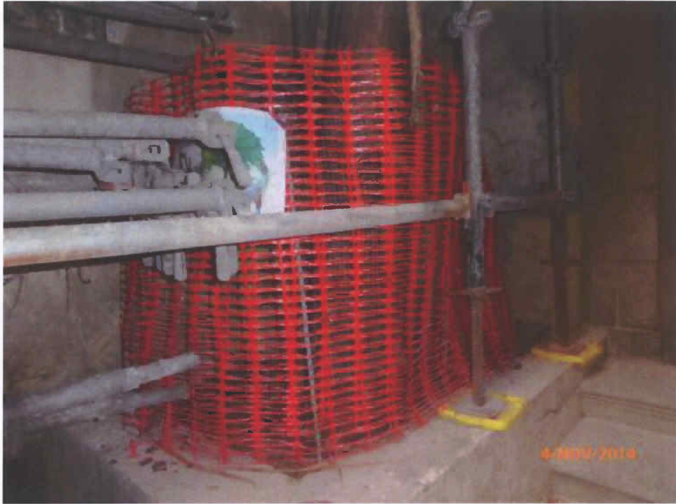
Fig. 8 The small cordon zone is in order.
