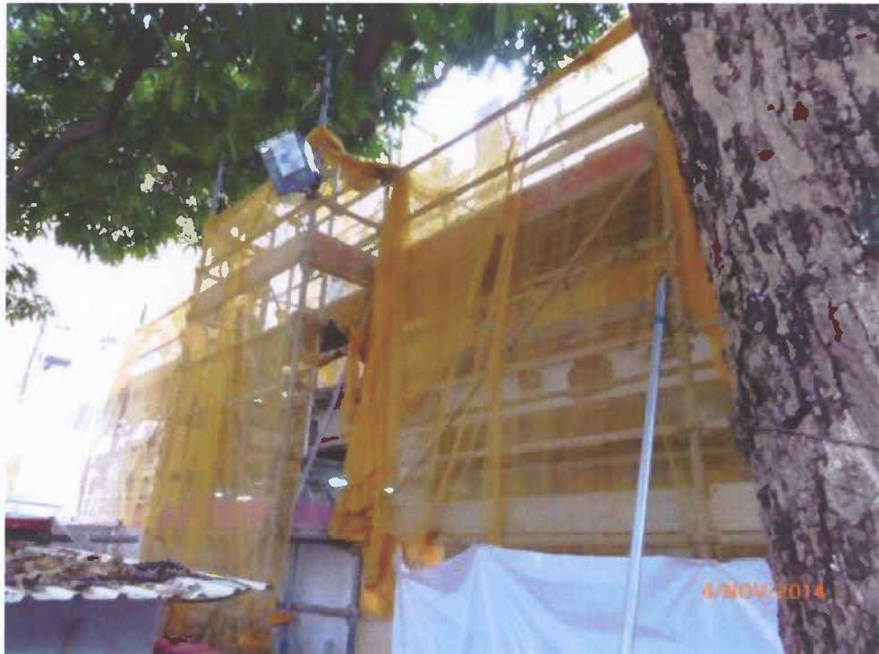
Fig. 6 Renovation work is in progress near the tree.
