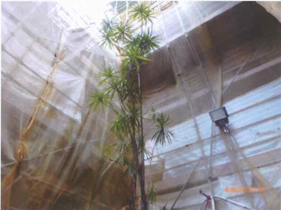
Fig. 11 Renovation work is in progress near Tree-11.
