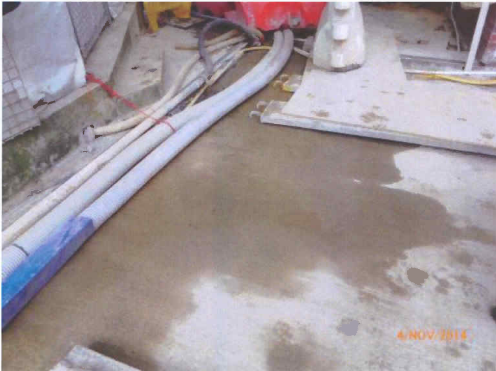
Fig. 9 The site outside the cordon zone also is clean and tidy.
