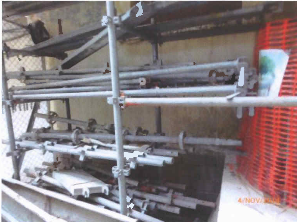
Fig. 10 Many metal tubes are still placed near the planter.
