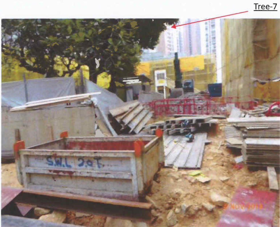
Fig. 9 Construction works are in progress outside the cordon zone.
