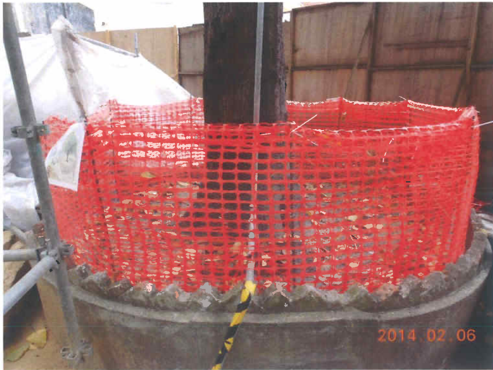
Fig. 6 A small cordon zone is newly set up to protect the tree.
