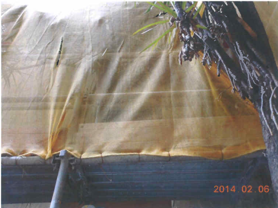
Fig. 7 Scaffold is still set up at site for renovation work.
