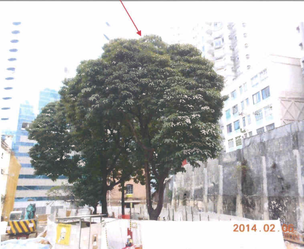
Fig. 9 Front view of Tree-6 during inspection on 6 th February 2014.
