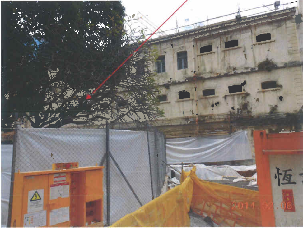
Fig. 6 Construction works are in progress near Tree-8.
