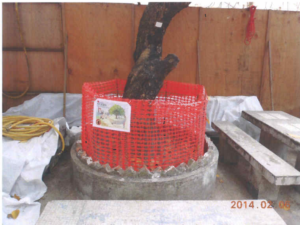
Fig. 3 A small cordon zone is newly set up to protect the tree.
