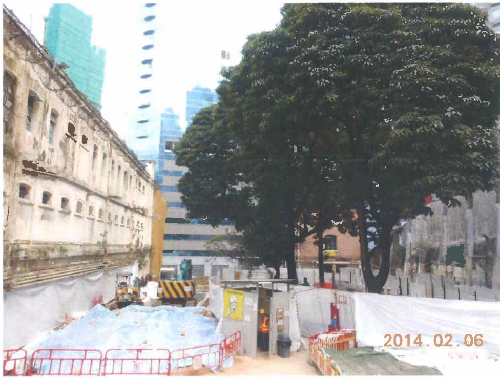
Fig. 10 Construction works outside the cordon zone are nearly completed.
