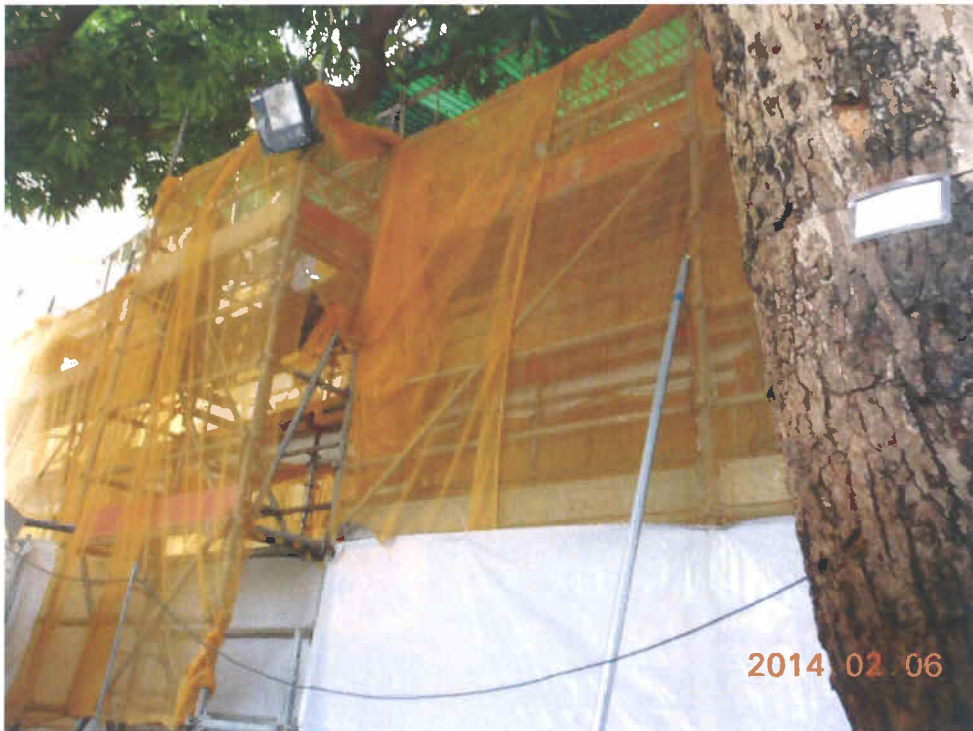
Fig. 9 Renovation works are in progress in the vicinity of the tree.
