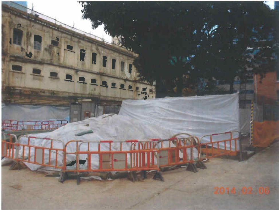
Fig. 8 Construction works are nearly completed in the vicinity of the tree.
