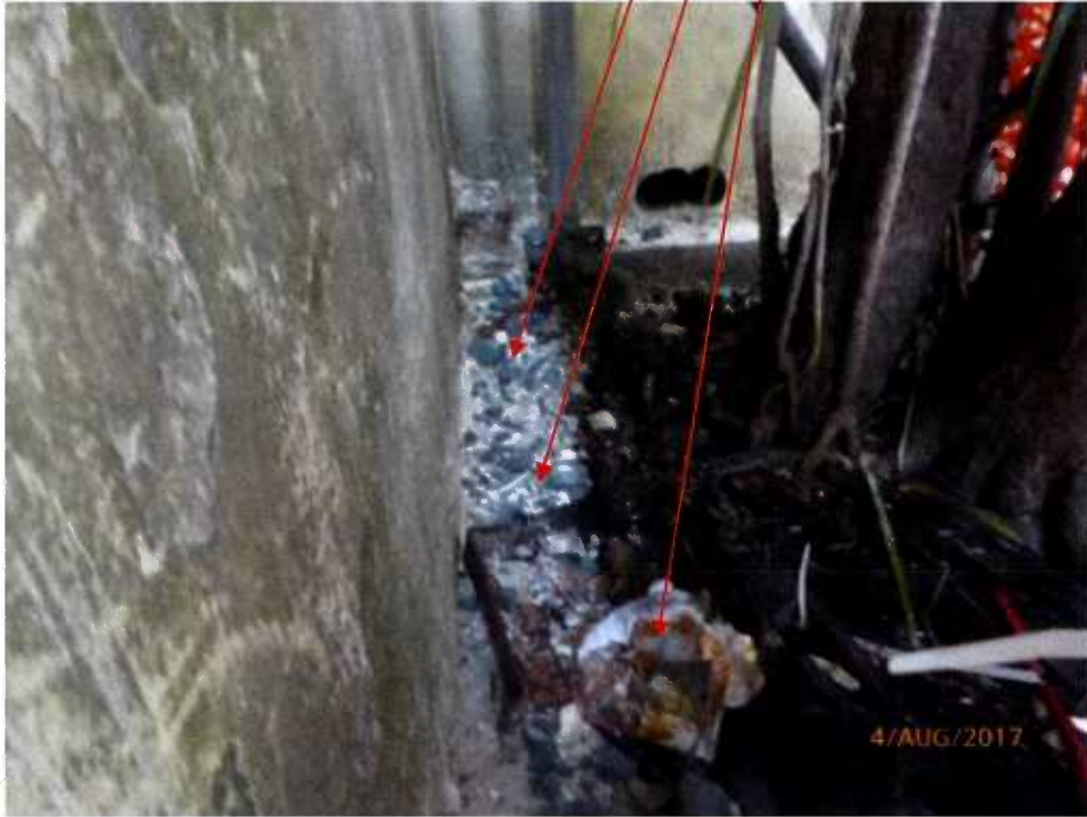
Fig. 2 Root collar is normal. Lots of construction debris remain at the corner of the planter.
