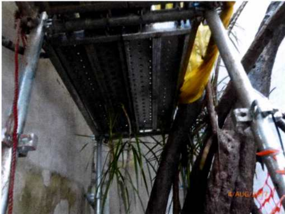
Fig. 9 A working platform is set up close to Tree-11.
