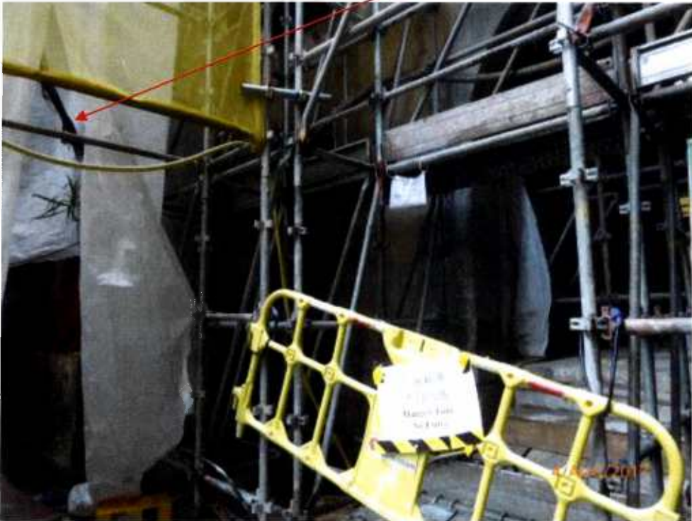
Fig. 11 Renovation works are in progress near Tree-11 .
