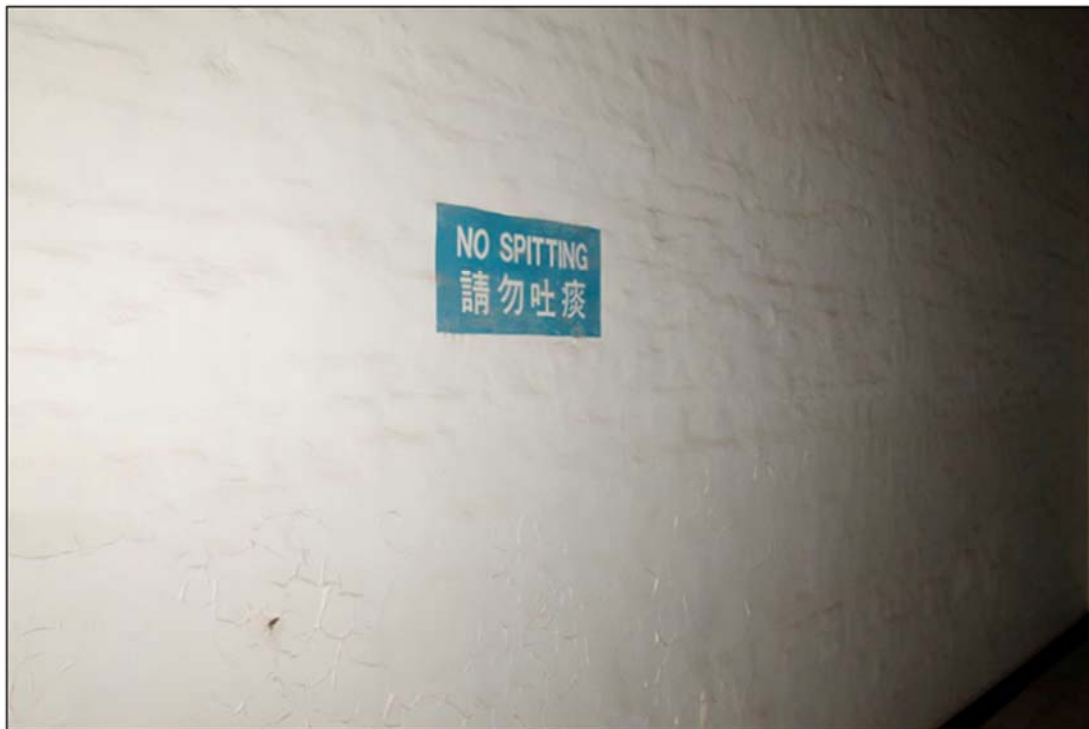
Photo 03-2F-230 General view of the wall (21-3-2012)
