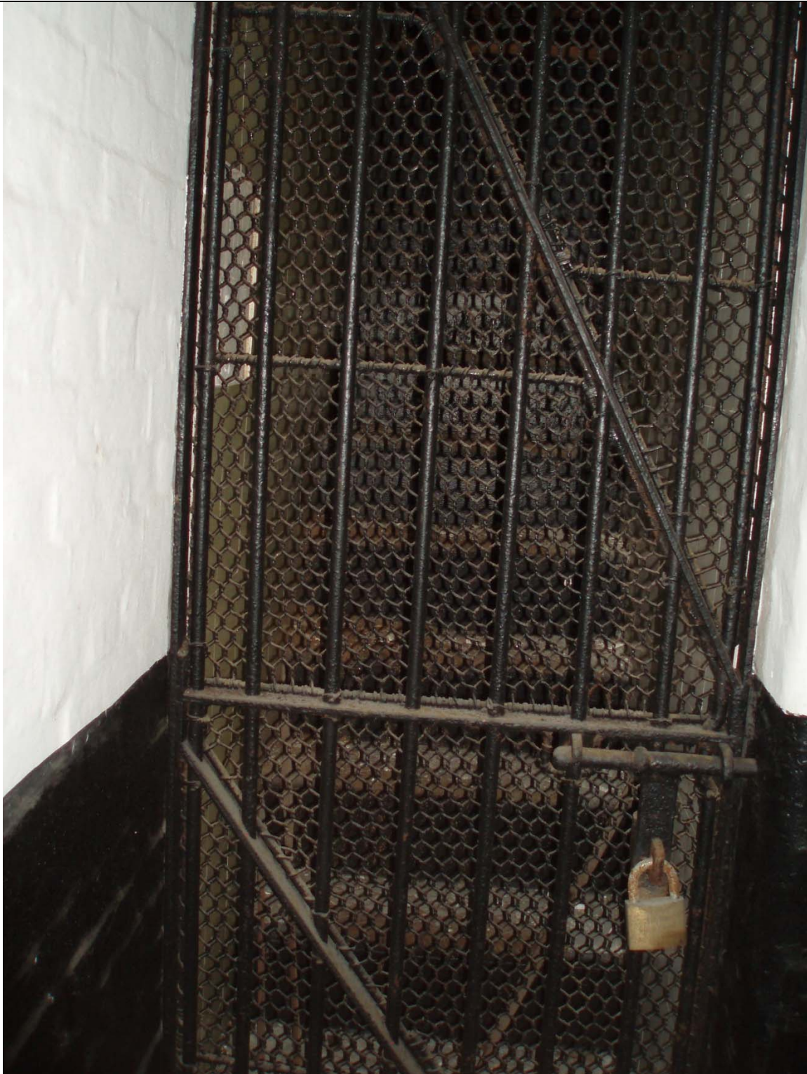
Above, photograph taken on 27 th July 2009, showing the overall view of the metal gate leading to the staircase upstairs.
