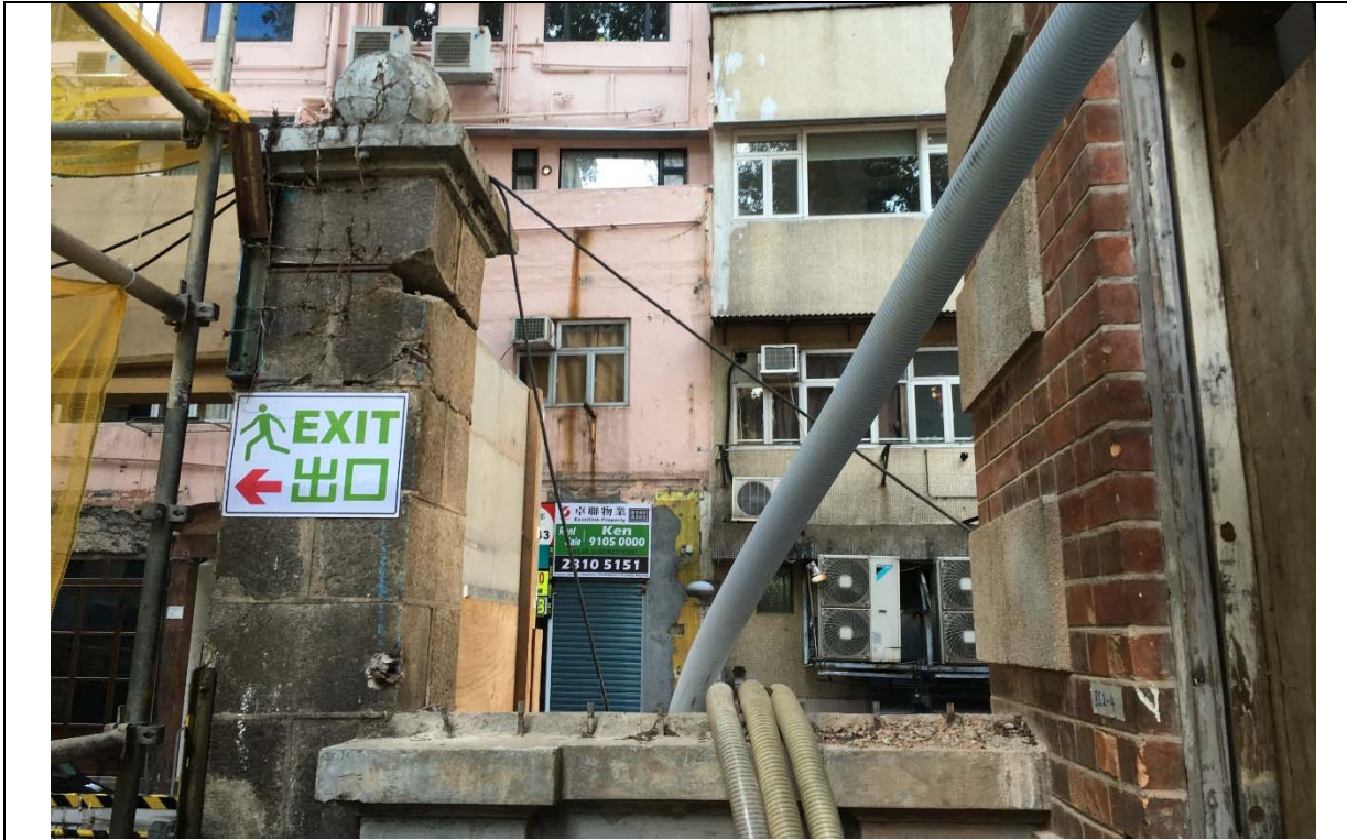
Above, photograph taken on 25 th January 2016, showing the fence was missing.
