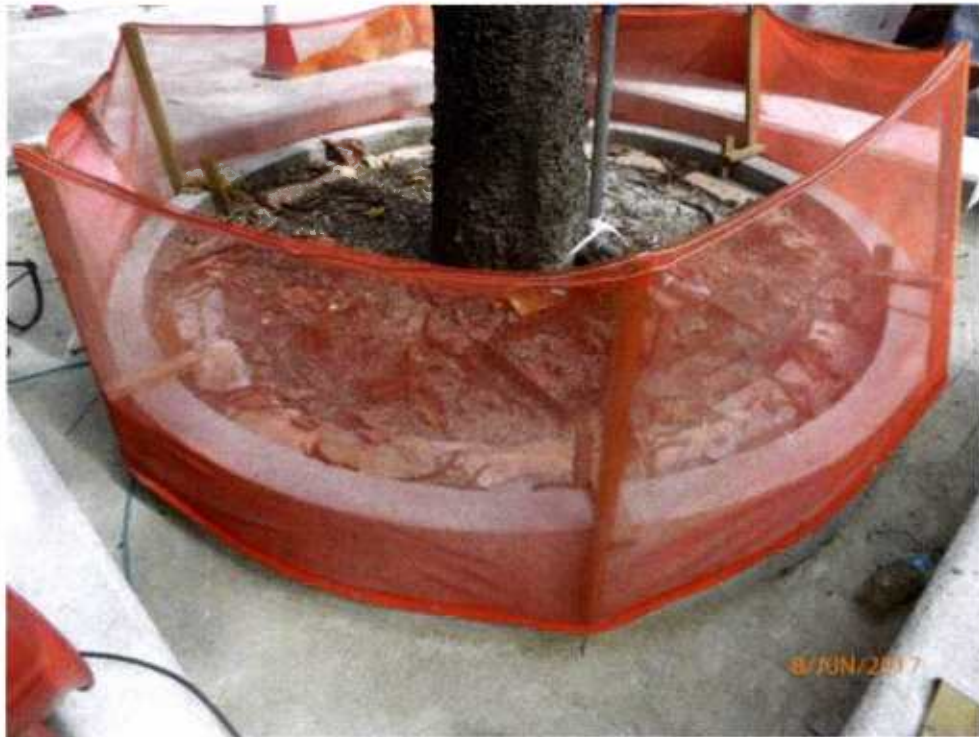
Fig. 9 A Tree Protection Zone is newly erected to protect the tree.
