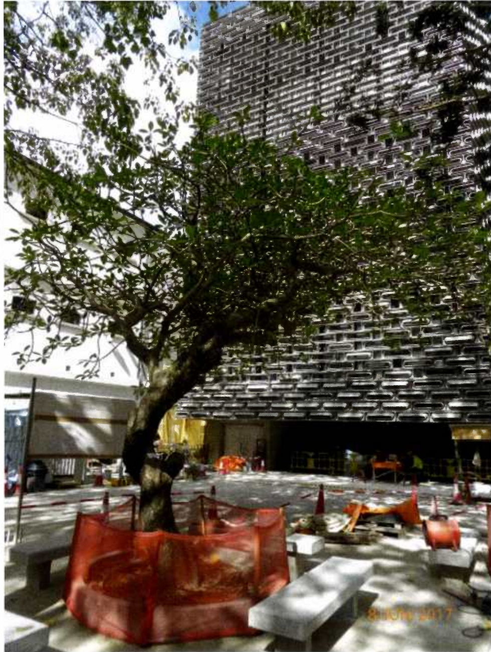
Fig. 12 Overall view of Tree-8 during inspection on 8 th Jun. 2017.
