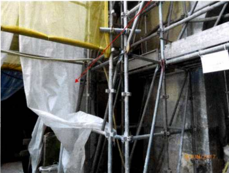
Fig. 11 Renovation works are in progress near Tree-11 .
