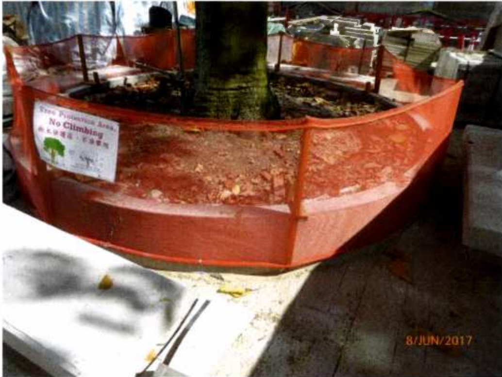
Fig. 10 A Tree Protection Zone is newly erected to protect the tree.
