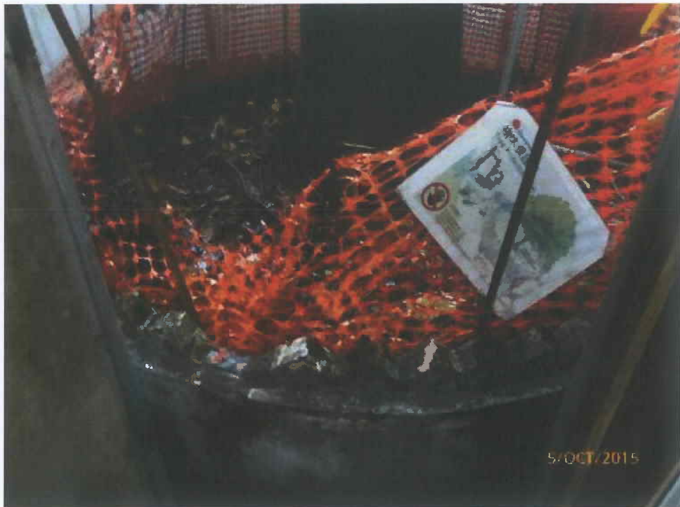
Fig. 9 The small cordon zone is in order at the planter.
