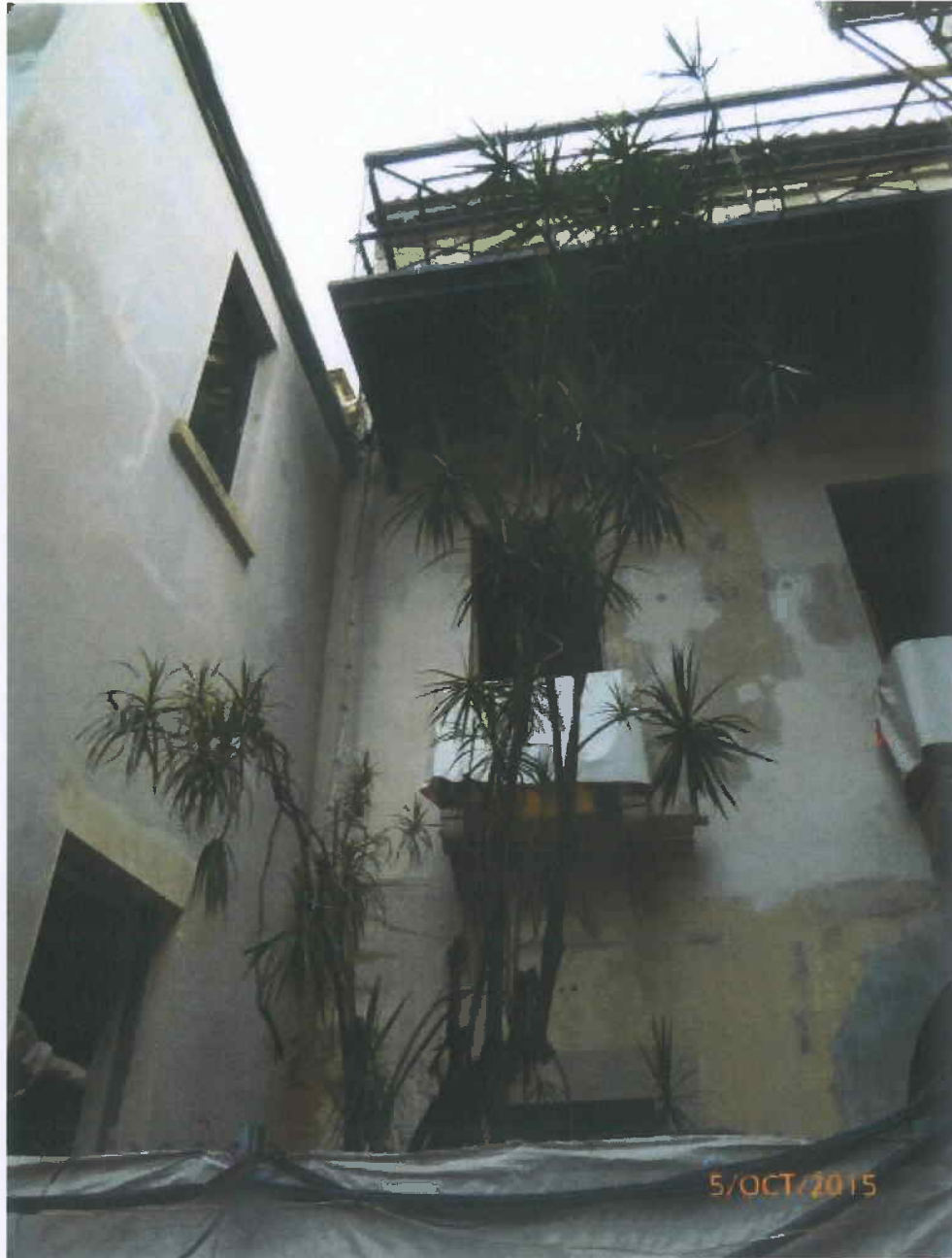
Fig. 12 Overall view of Tree-11 during inspection on 5 th October 2015.
