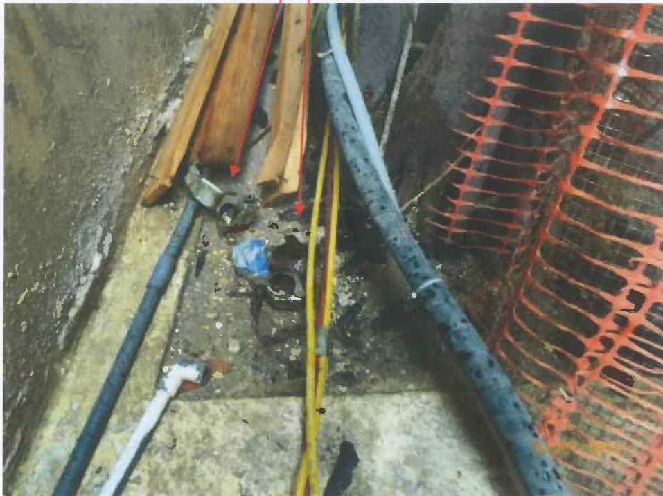
Fig. 3 Lots of construction debris are found on the bottom part of the tree.
