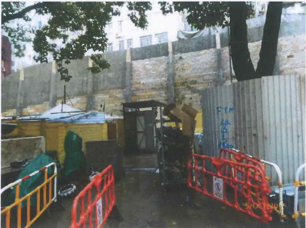
Fig. 11 Construction works are in progress near Tree-6.
