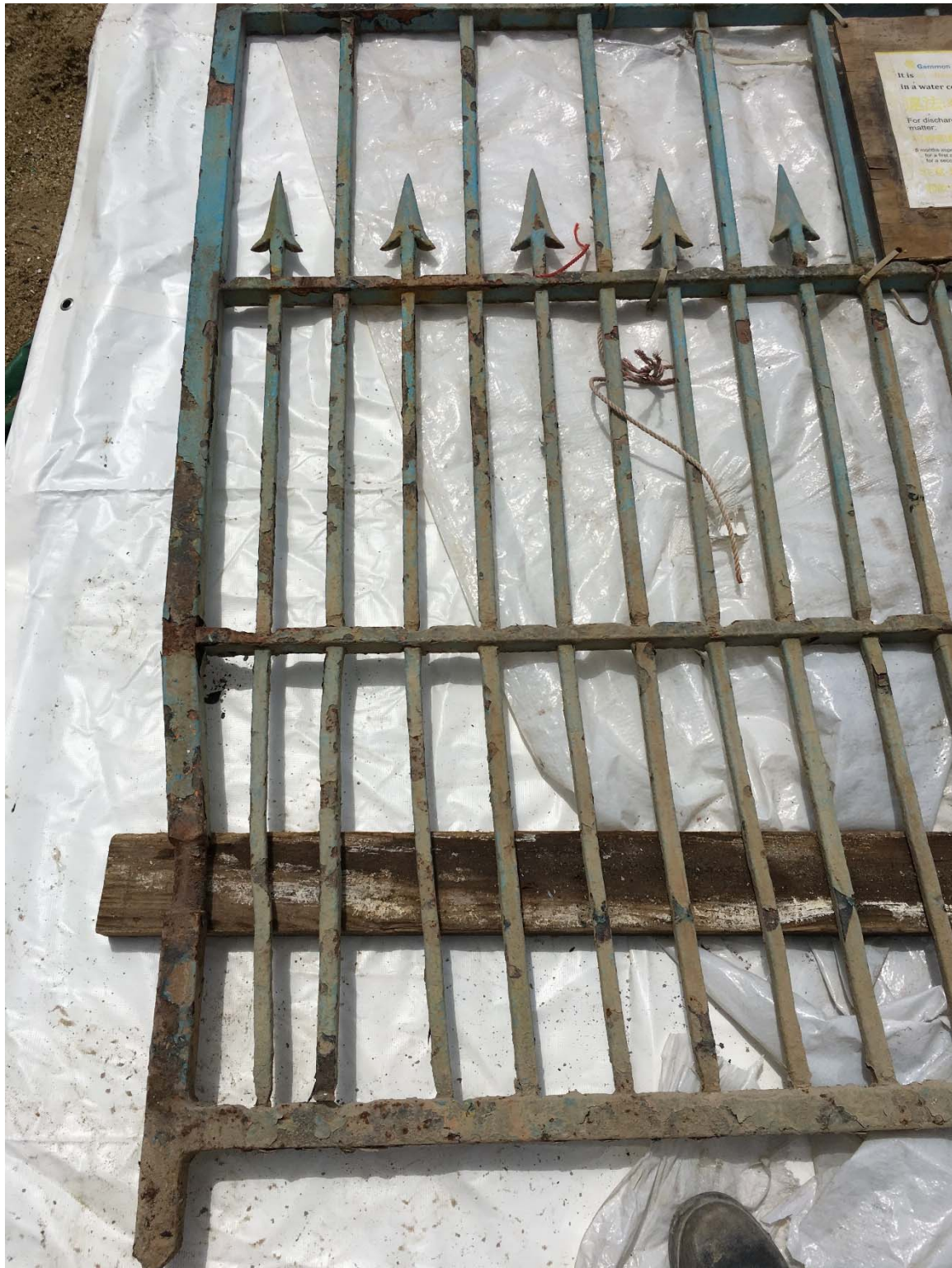
Above, photo taken on 21 st July 2016, showing the bottom of the right hand side leaf was out of shape.
