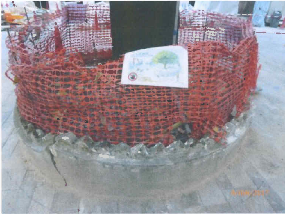
Fig. 10 We recommend to erect a Tree Protection Zone (similar to the following photo) at the planter especially during the nearby renovation works are in progress.
