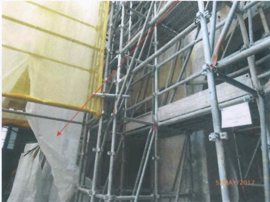
Fig. 10 Renovation works are in progress near Tree-11 .
