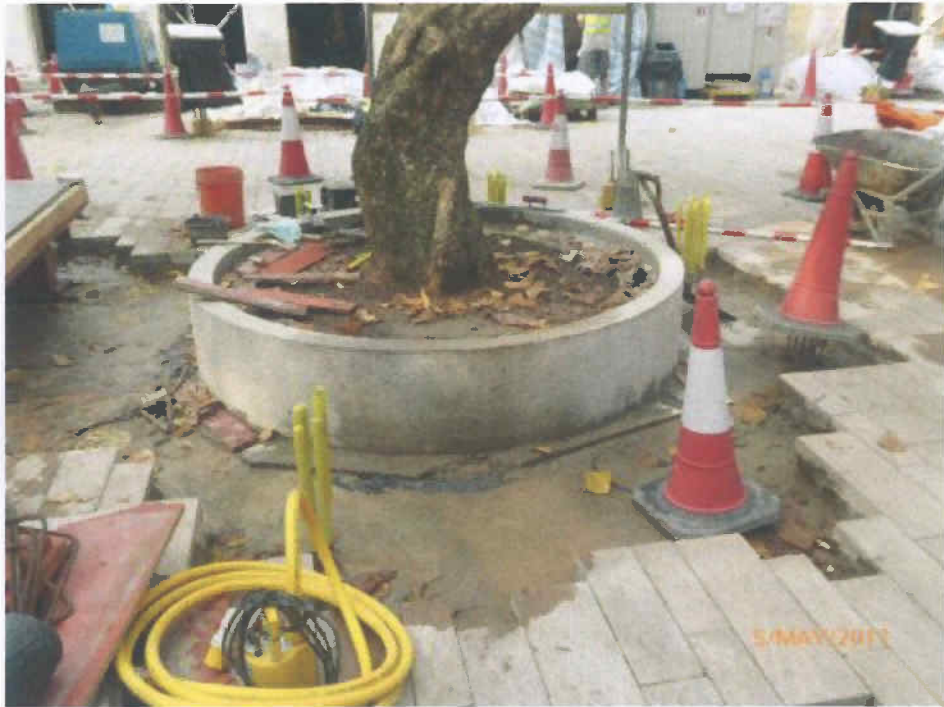
Fig. 8 Repairing of the planter is nearly completed. It seems that the workers just poured some polluted water into the planter.
