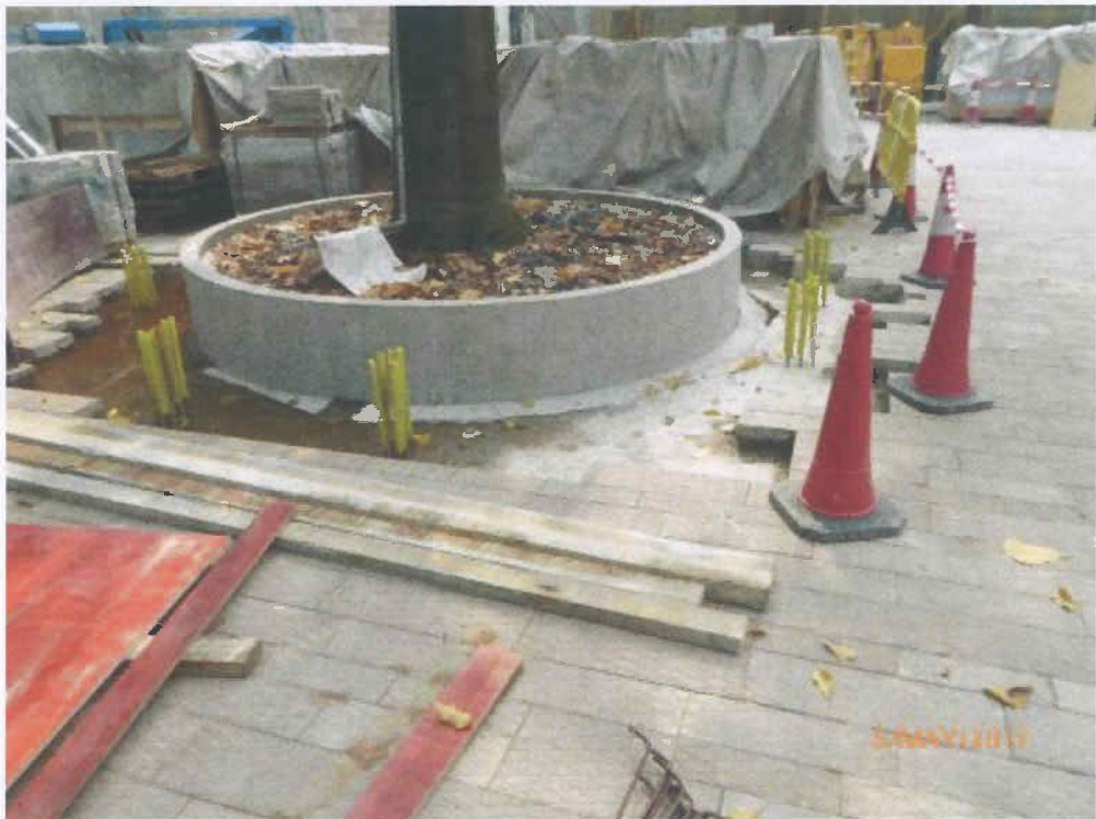
Fig. 9 Repairing of the planter is nearly completed.
