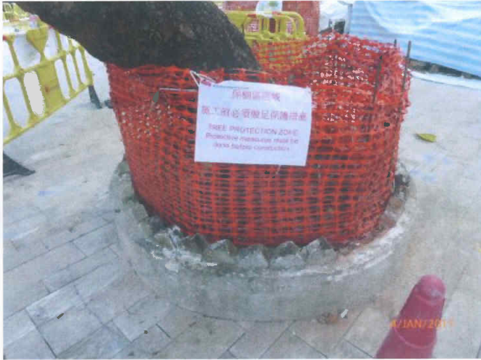
Fig. 10 We recommend to erect a Tree Protection Zone (similar to the following photo) at the planter especially during the nearby renovation works are in progress.
