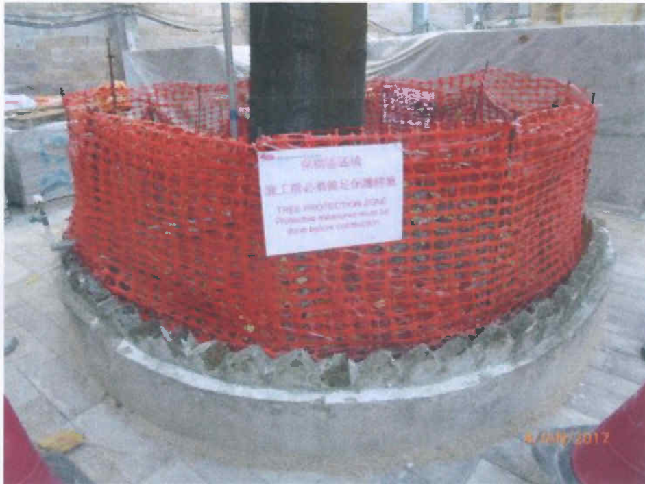
Fig. 10 We recommend to erect a Tree Protection Zone (similar to the following photo) at the planter especially during the nearby renovation works are in progress.
