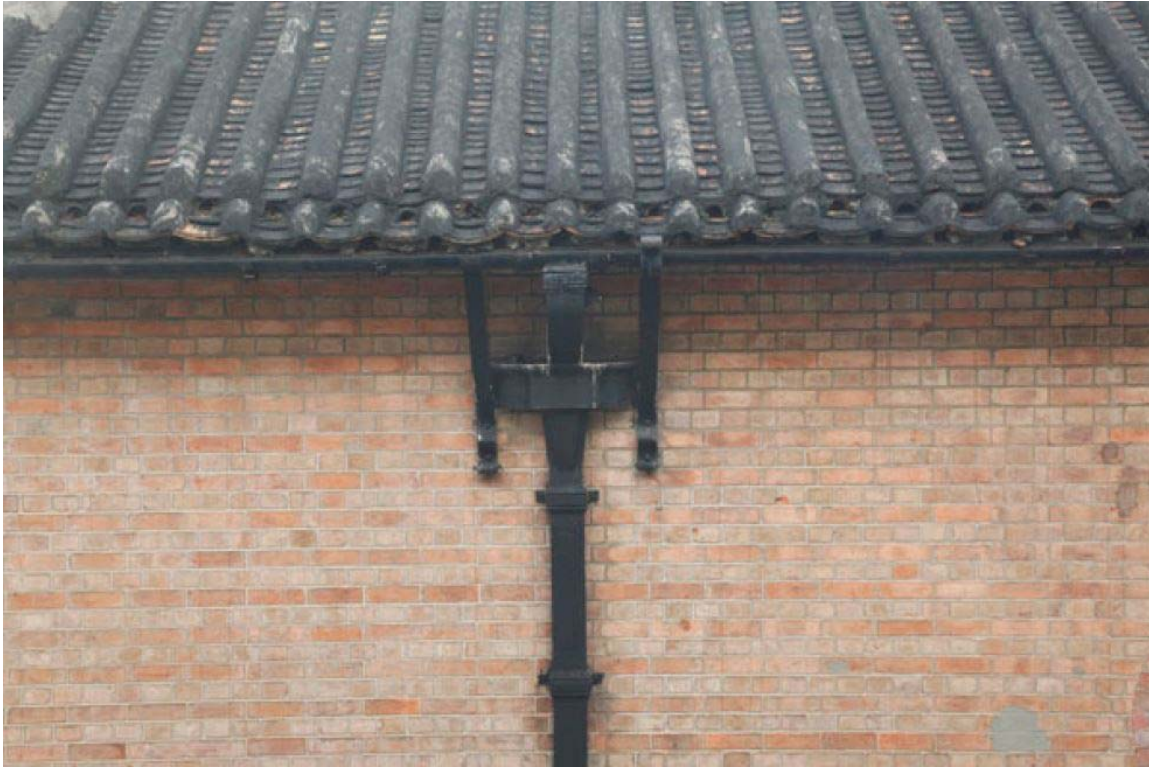
Above, photo taken on 17 th August 2011, showing the historic hopper at its location.
