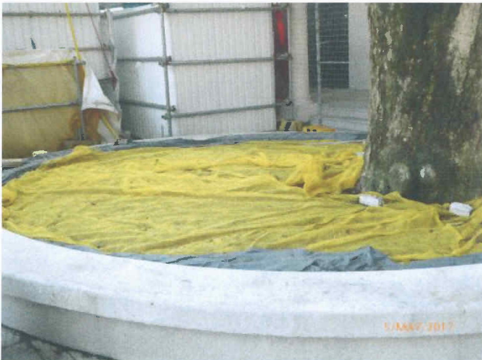
Fig. 9 Repairing of the planter is nearly completed.
