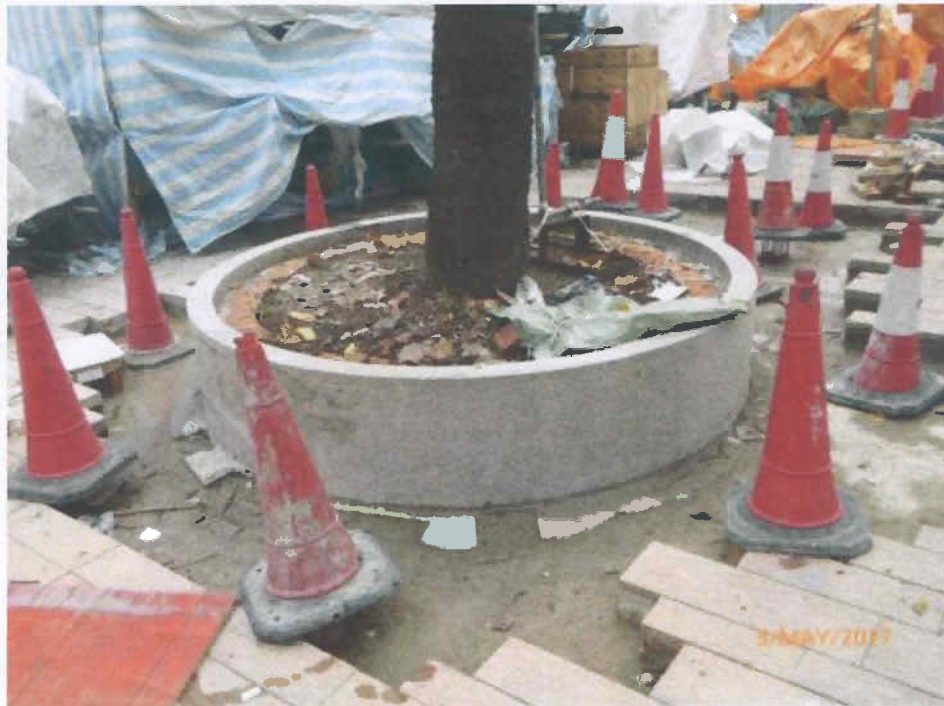
Fig. 9 Repairing of the planter is nearly completed.
