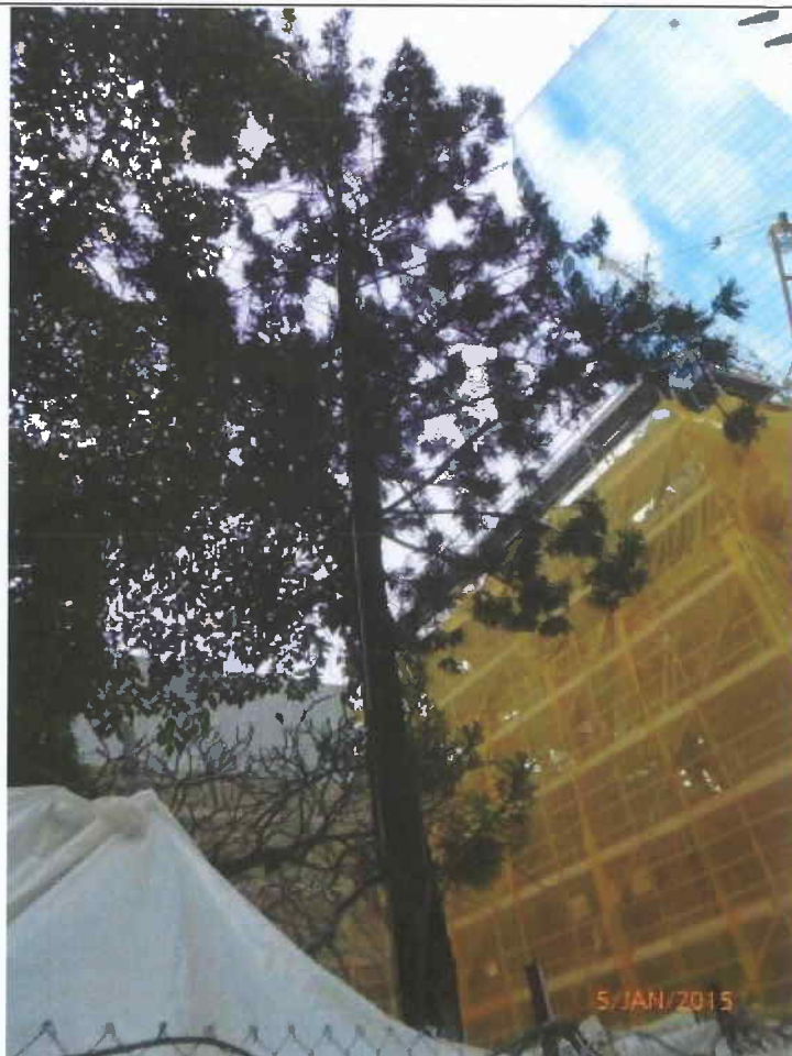
Fig. 11 Side view of Tree-9 during inspection on 5 th January 2015.
