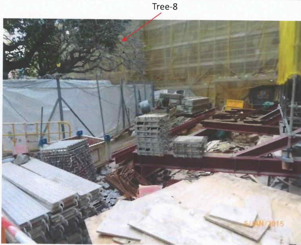
Fig. 10 Construction works are in progress outside the cordon zone.
