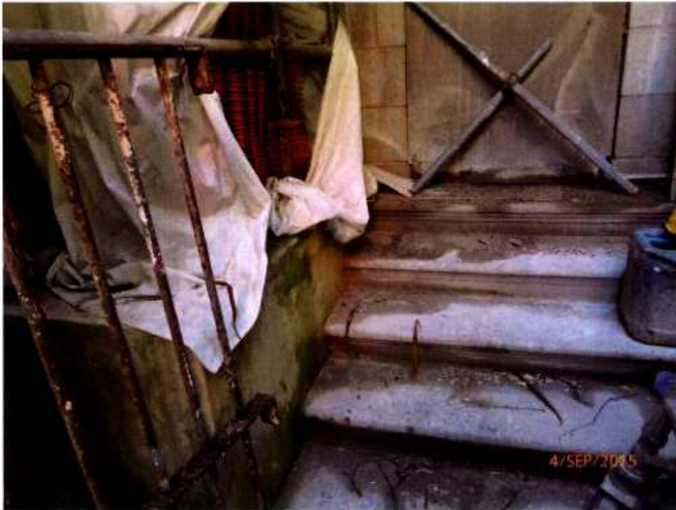
Fig. 10 Cleanliness of the site near Tree-11 is acceptable.
