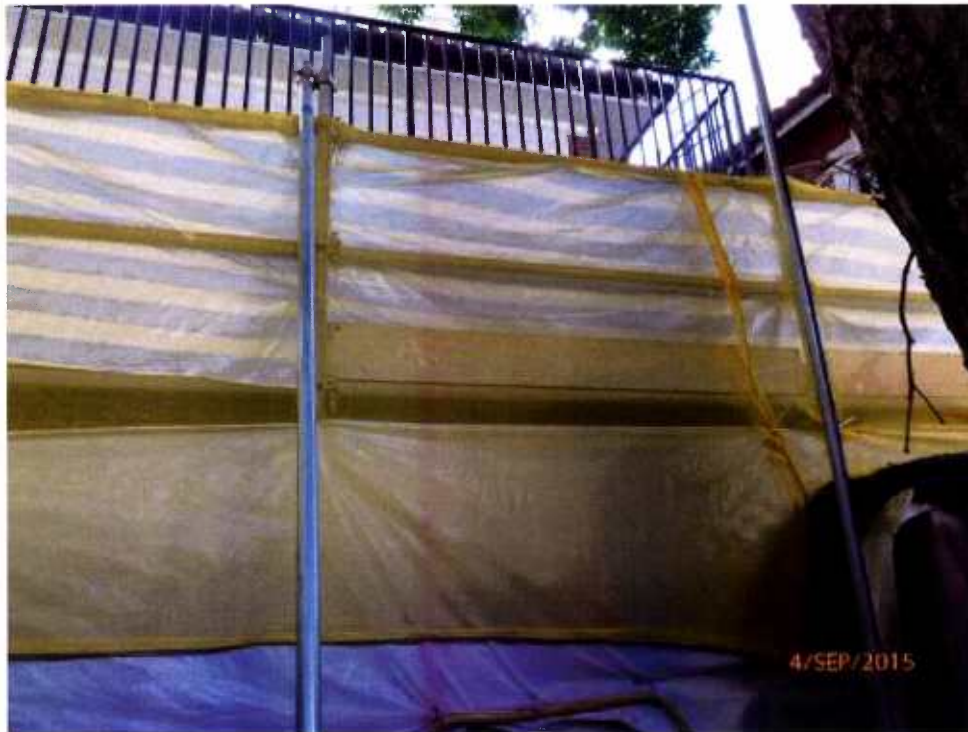
Fig. 8 Renovation works are in progress near Tree-5.
