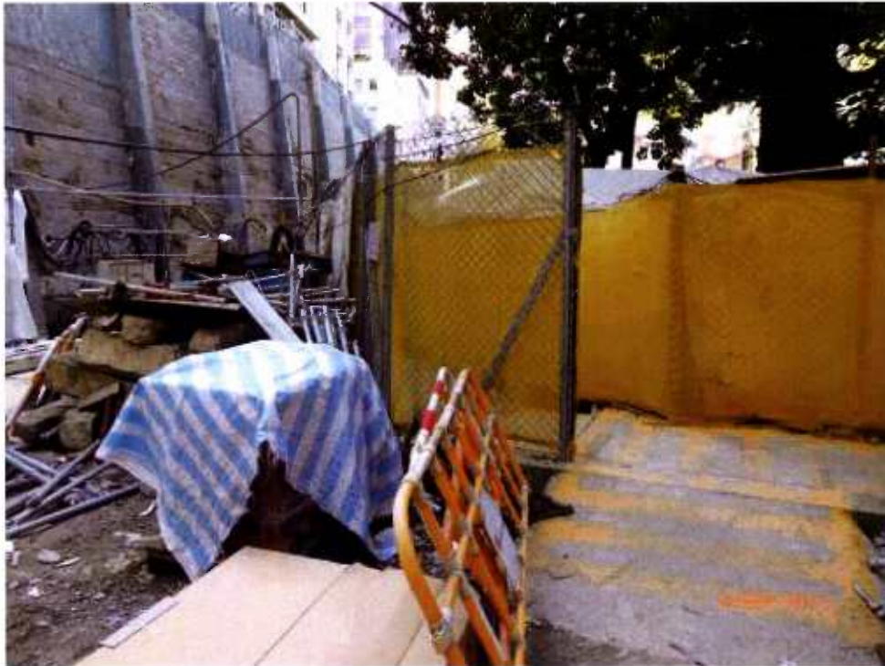
Fig. 10 Construction works are in progress outside the cordon zone.
