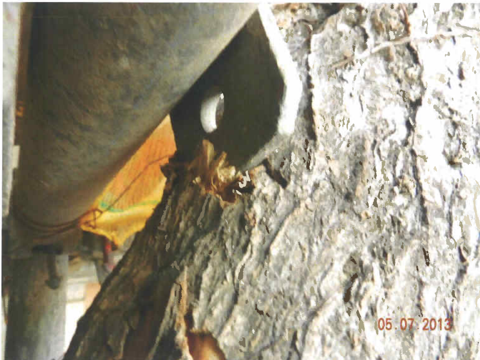
Fig. 5 The sharp edge of the scaffold has stabbed into the tree.
