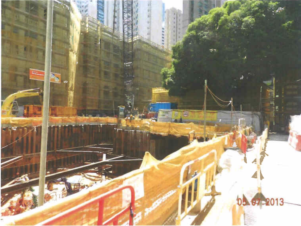
Fig. 6 Construction works are in progress outside the cordon zone.
