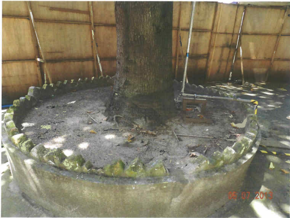
Fig 2. The planter keeps clean and tidy.
