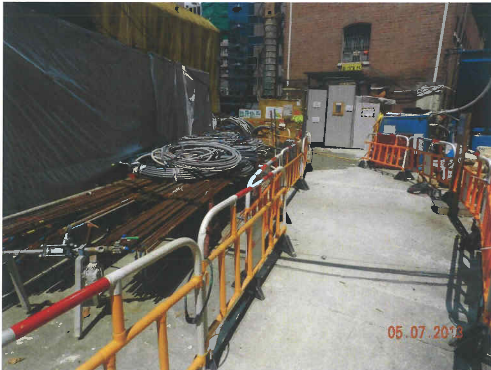
Fig. 7 The site outside the cordon zone is clean and tidy.
