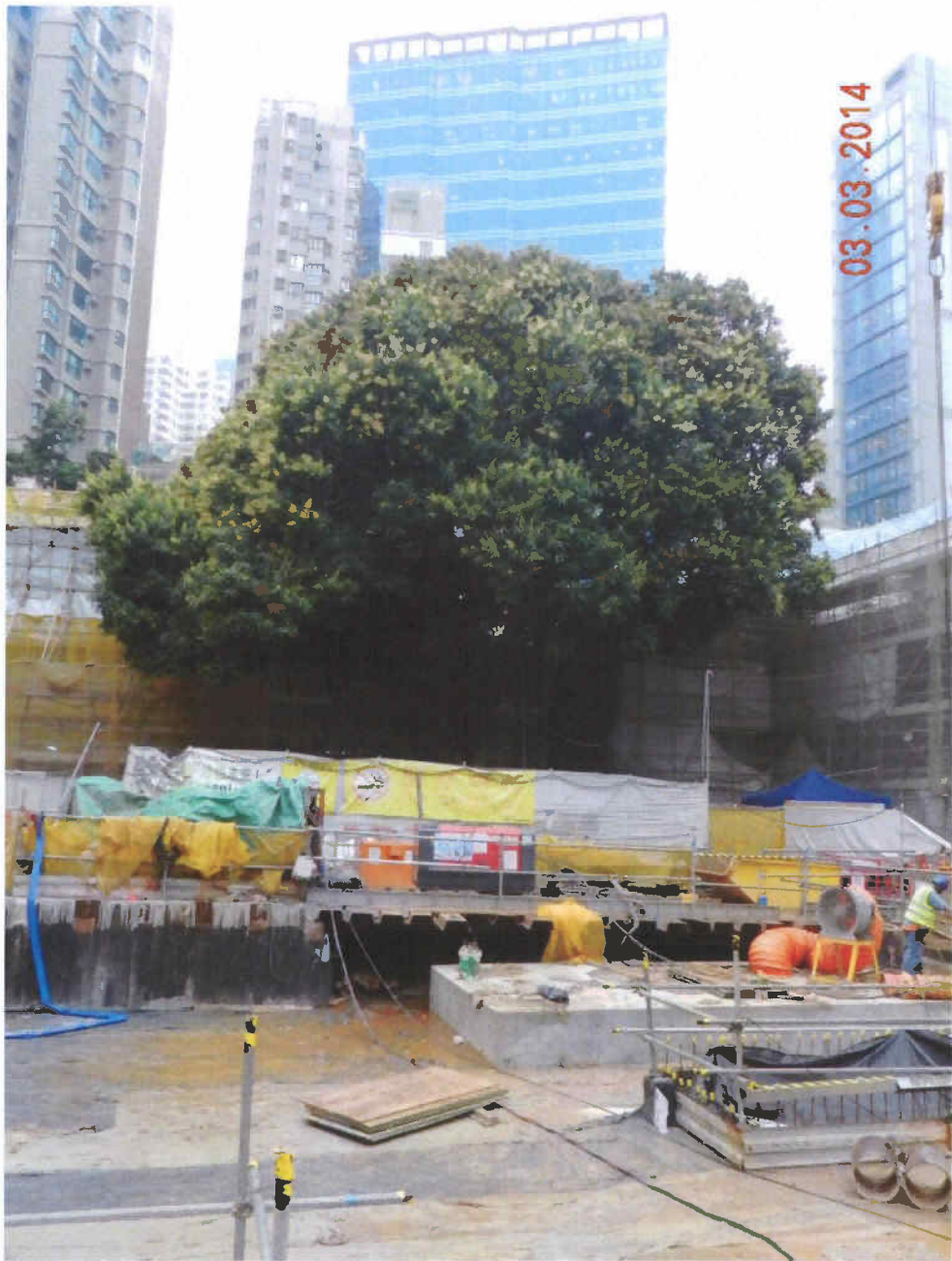
Fig. 10 Overall view of Tree-5 during inspection on 3 rd March 2014.
