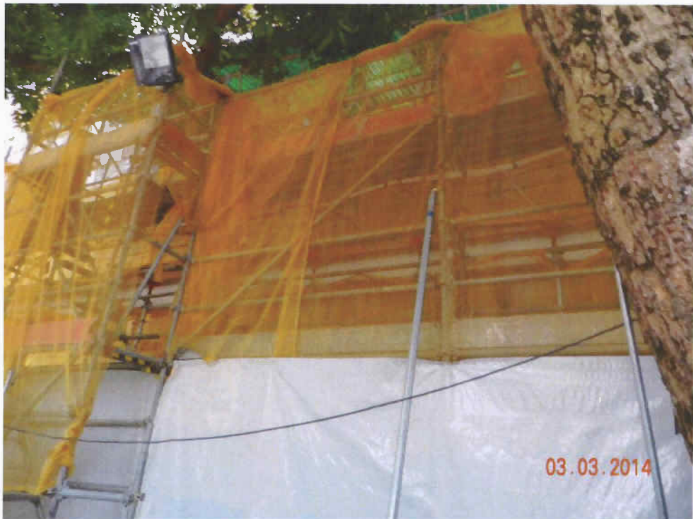
Fig. 5 Renovation works are in progress in the vicinity of the tree.
