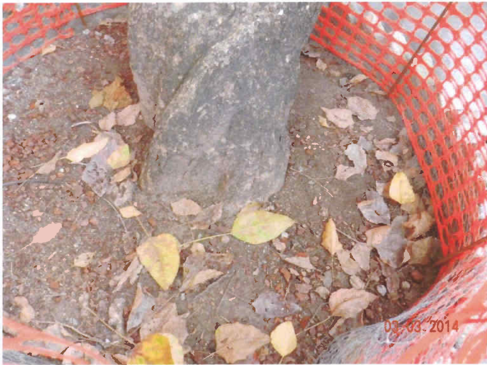
Fig 2. The root collar is normal, some small pieces of mulch have been added on the planter.
