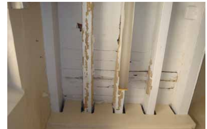
Figure 6 - Exposed ceiling structure in the second floor staircase hall
