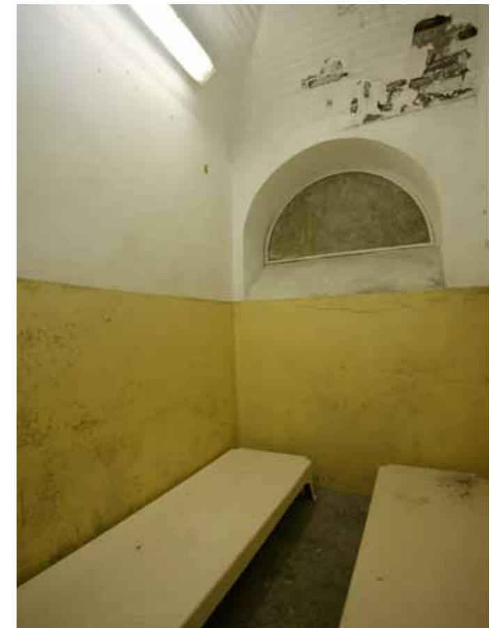
Figure 9 - A typical west wing first floor cell
