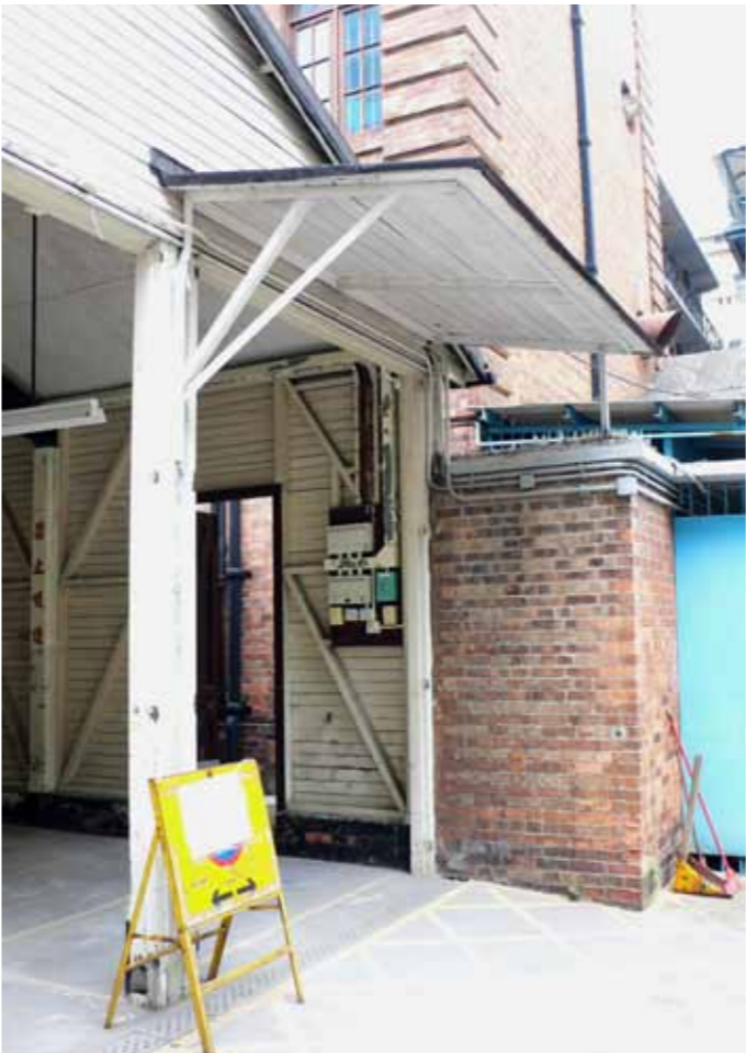
Figure 2 - Detail view of a sunshade on the west side
