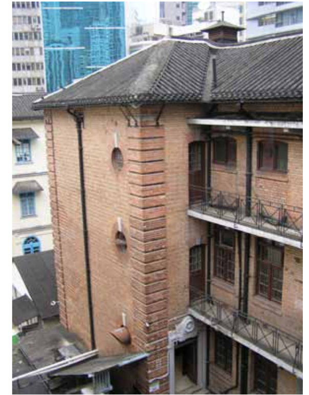
Figure 3 - West staircase block
