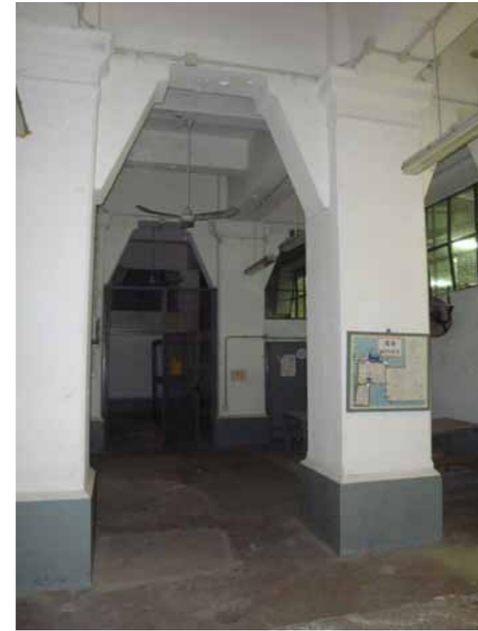
Figure 7 - View of the basement (undercroft) of E Hall with interesting columns
