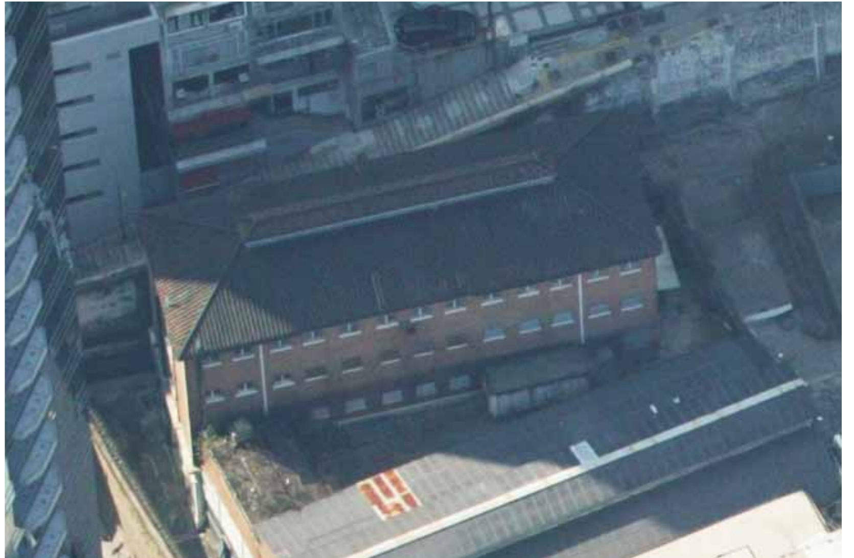
Aerial photograph of the building, where north is to the bottom of the image
