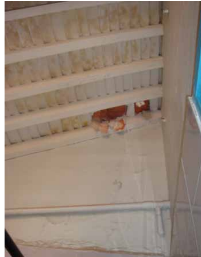
Figure 8 - Typical roof construction with the underside of the tiles visible over the staircase areas
