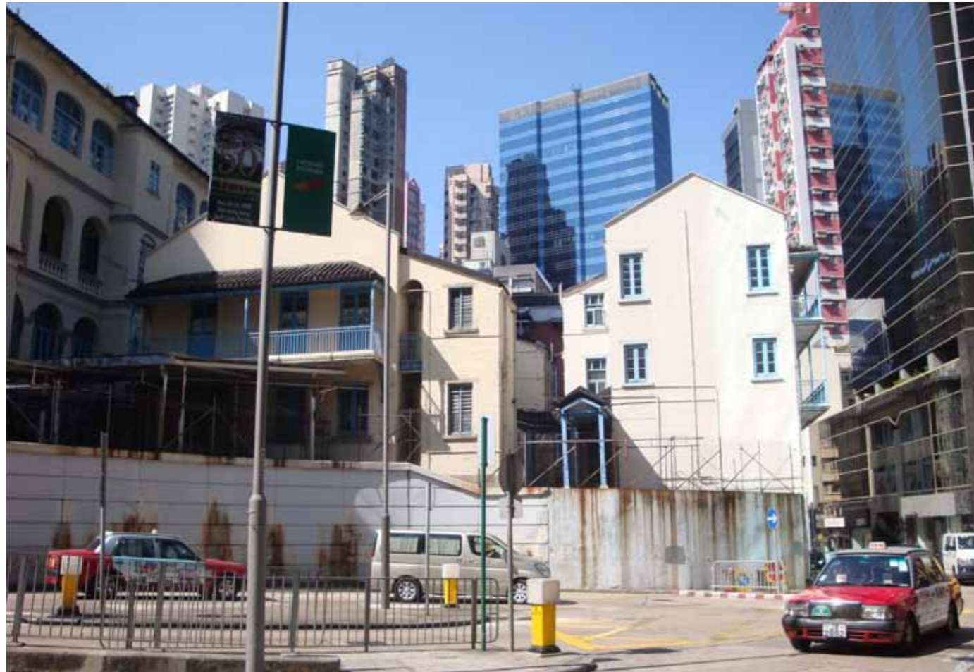
Figure 1 - East elevation of the building overlooking Arbutnot Road. Building 07 is on the right side of the image.
