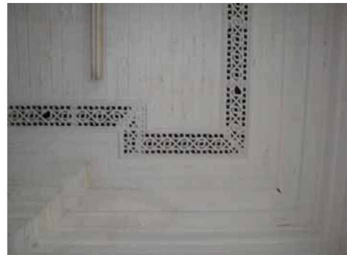
Figure 10 - Third floor ceiling with metal ventilation grille c.1929
