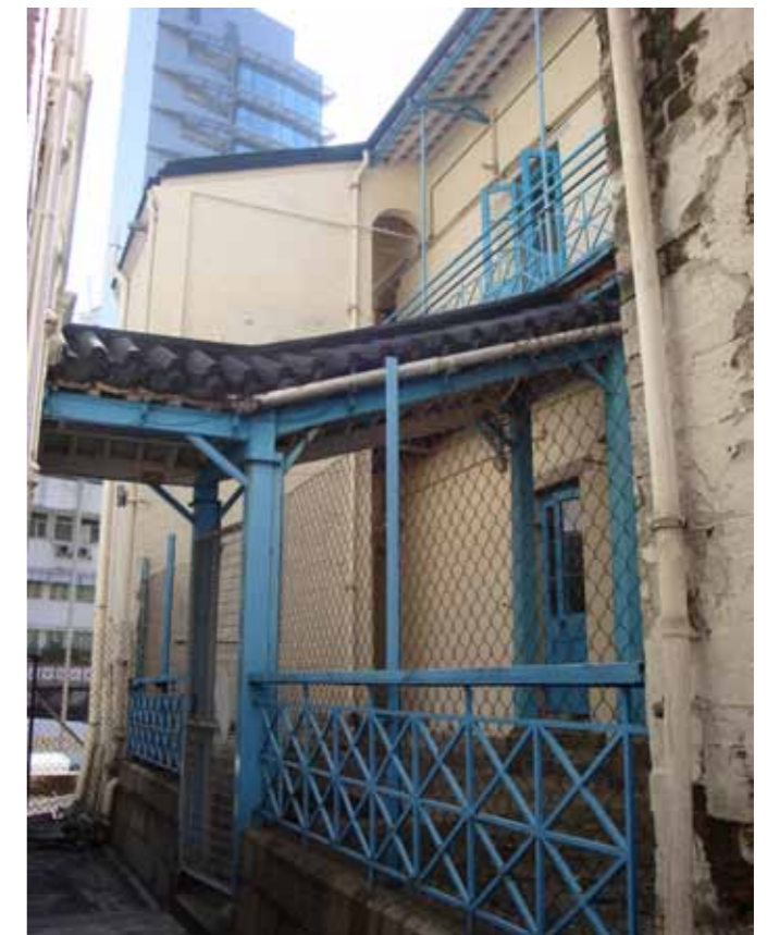
Figure 6 - Covered walkway leading to Building 07
