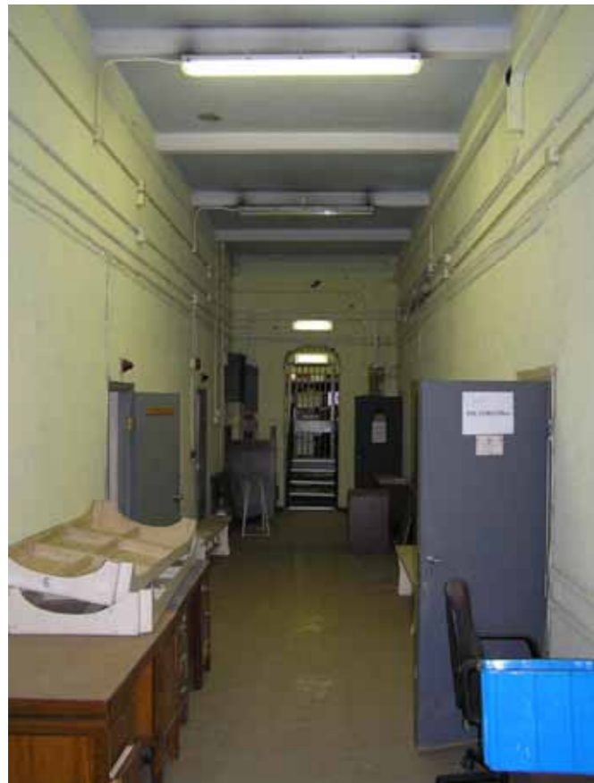
Figure 19 - The east wing ground floor corridor
