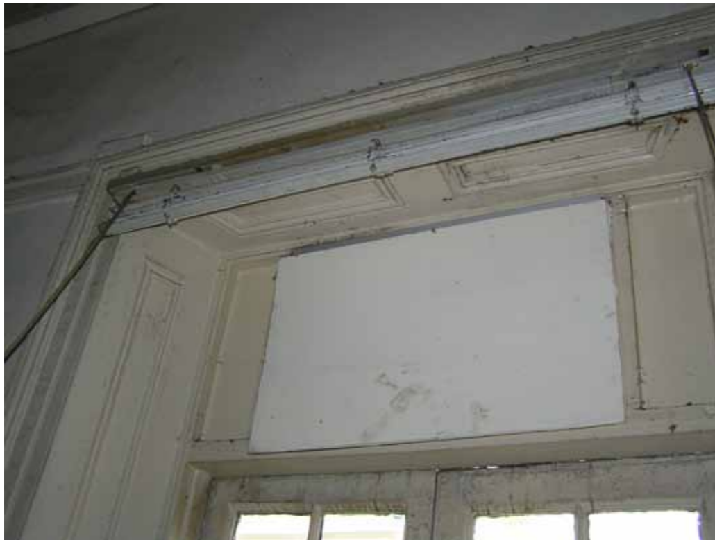
Figure 14 - Detail of panelled surrounds to a window
