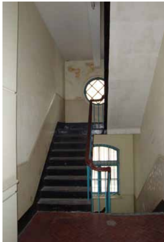
Figure 13 - Secondary staircase at west end
