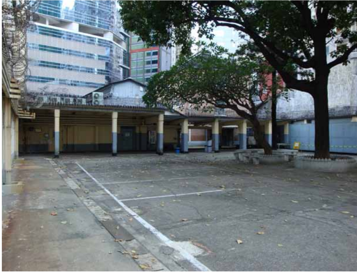
Figure 1 - View of west elevation from the Prison Yard showing columns of the covered walkway
