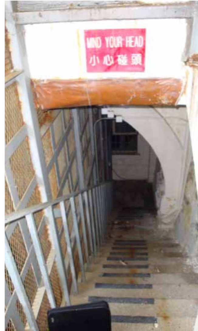
Figure 16 - The stairs leading down into the basement
