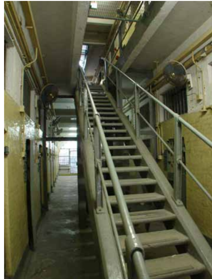
Figure 7 - One of the central staircases viewed from the ground floor
