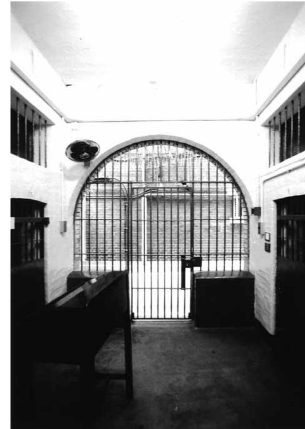
Interior view of each archway while prison still in use
