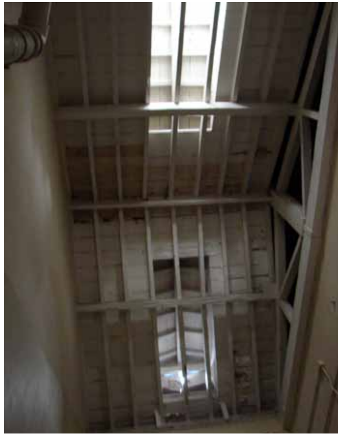
Figure 6 - Gabled roof over the main staircase
