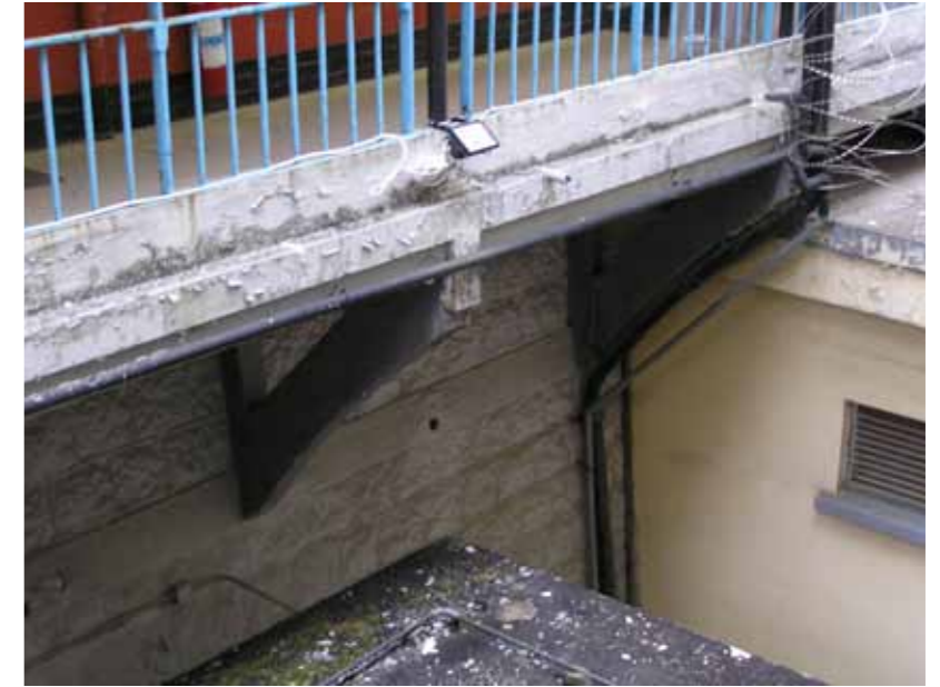
Figure 4 - Supporting brackets for the balconies
