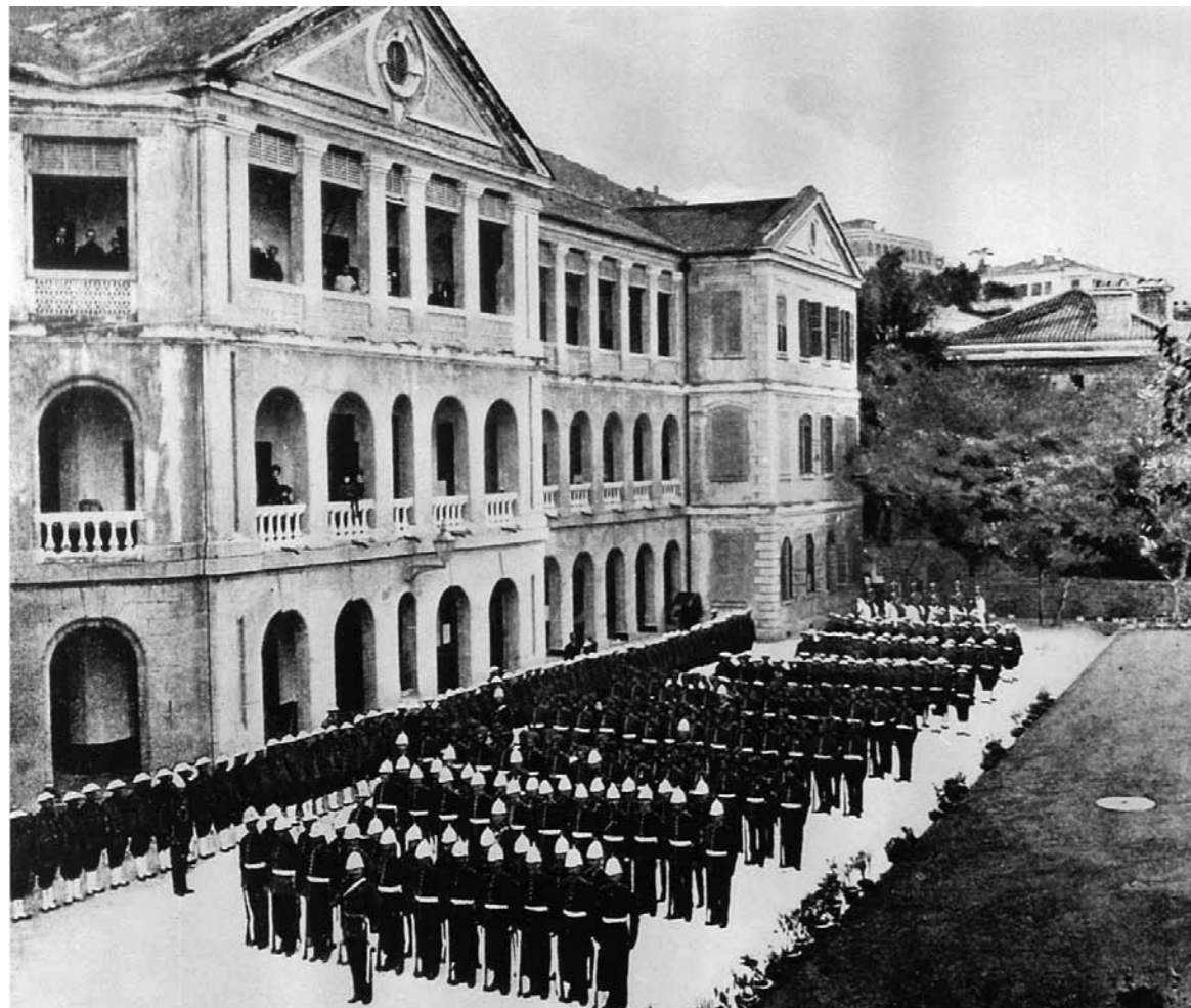
Late 19th century photograph of the Barracks Block (Building 03) showing the original gable of the same design as the Superintendent's House. This was lost in 1906 when a third floor was added.
