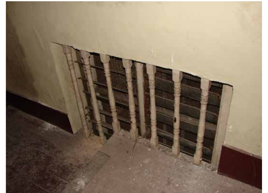
Figure 11 - Balustrade on a window opening in the main staircase wall
