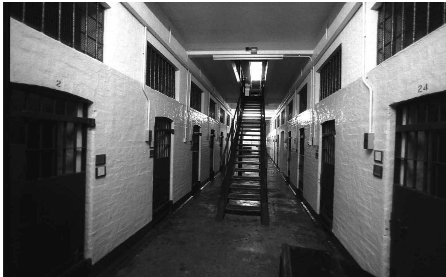
AMO photograph of the building still in use as a prison block. Note that each room only has two name card holders (indicating space for two prisoners per cell). At the time of decommissioning each cell was used by three prisoners at maximum capacity.
