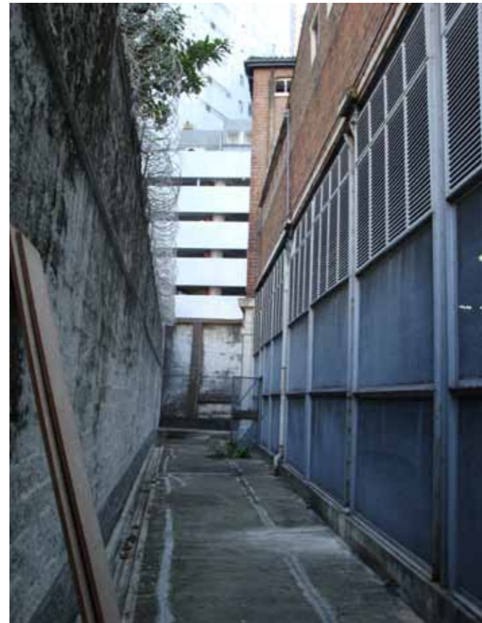
Figure 3 - The narrow alleyway on the east side ground floor between the Arbutnot Road wall and the east elevation of the Laundry
