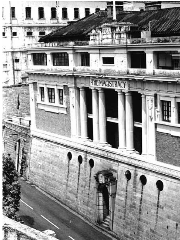
AMO photograph of the east elevation
