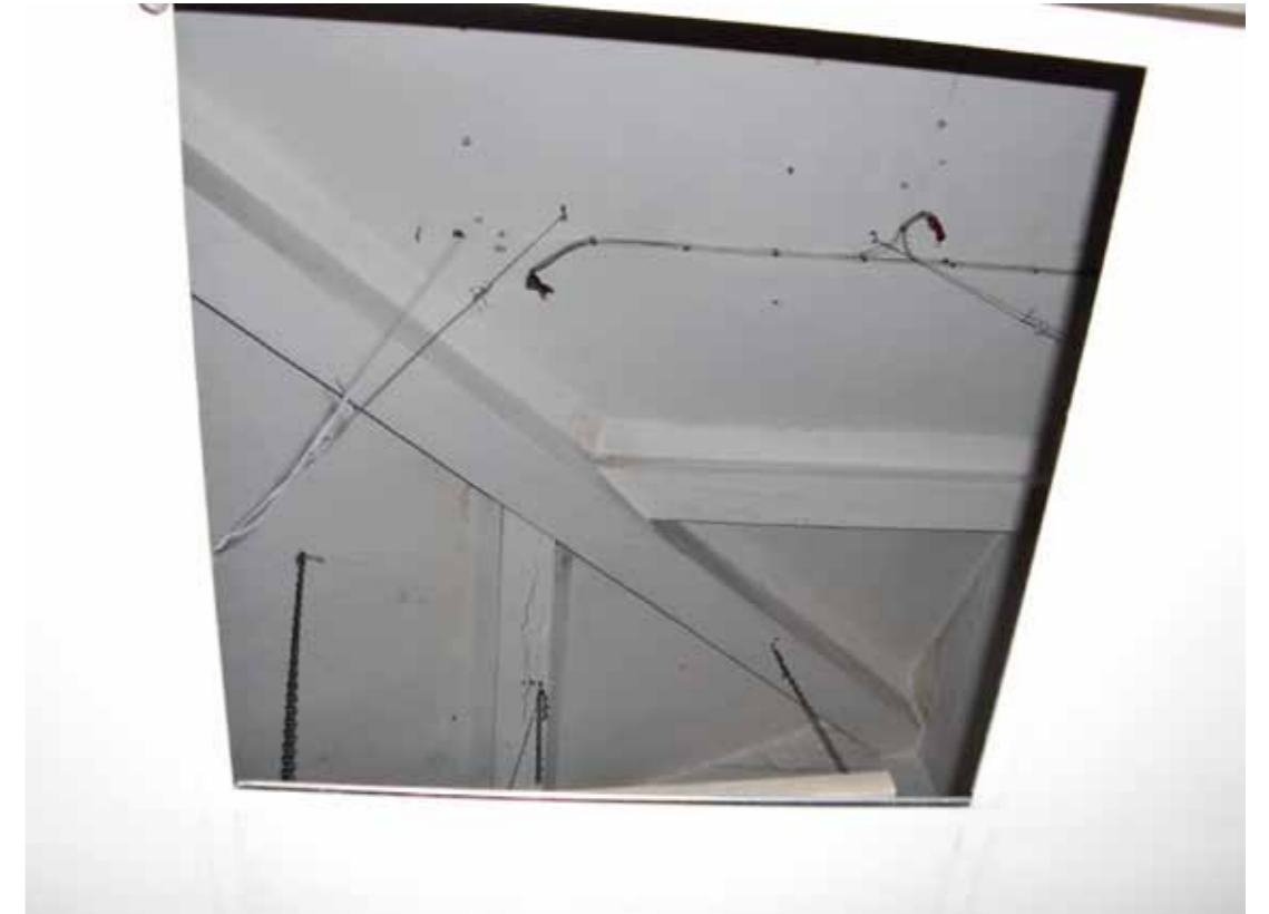
Figure 7 - Ceiling structure in 02/F/09
