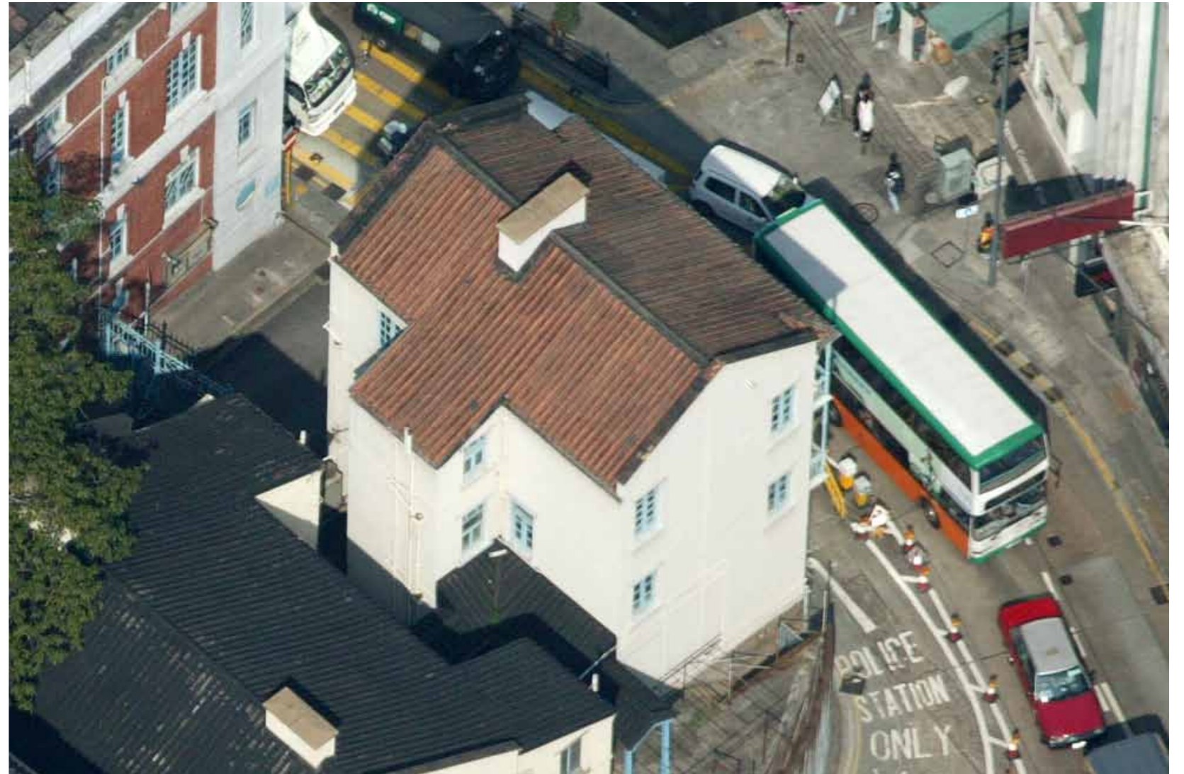
Aerial photograph showing Building 07, where north is to the upper left of the image
