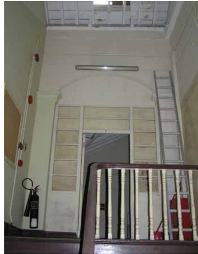
Figure 7 - Blocked archway leading into the west rooms on the first floor; these are thought to have been verandahs
