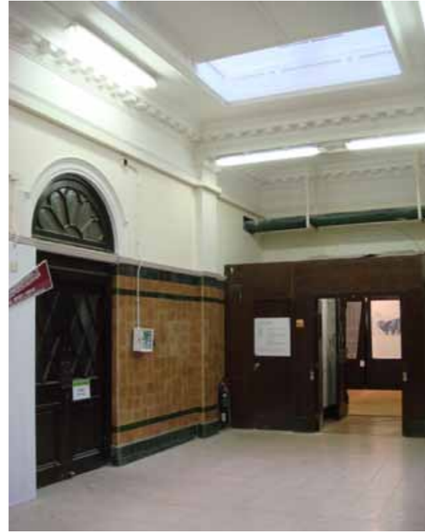
Figure 17 - Ground floor entrance hall
