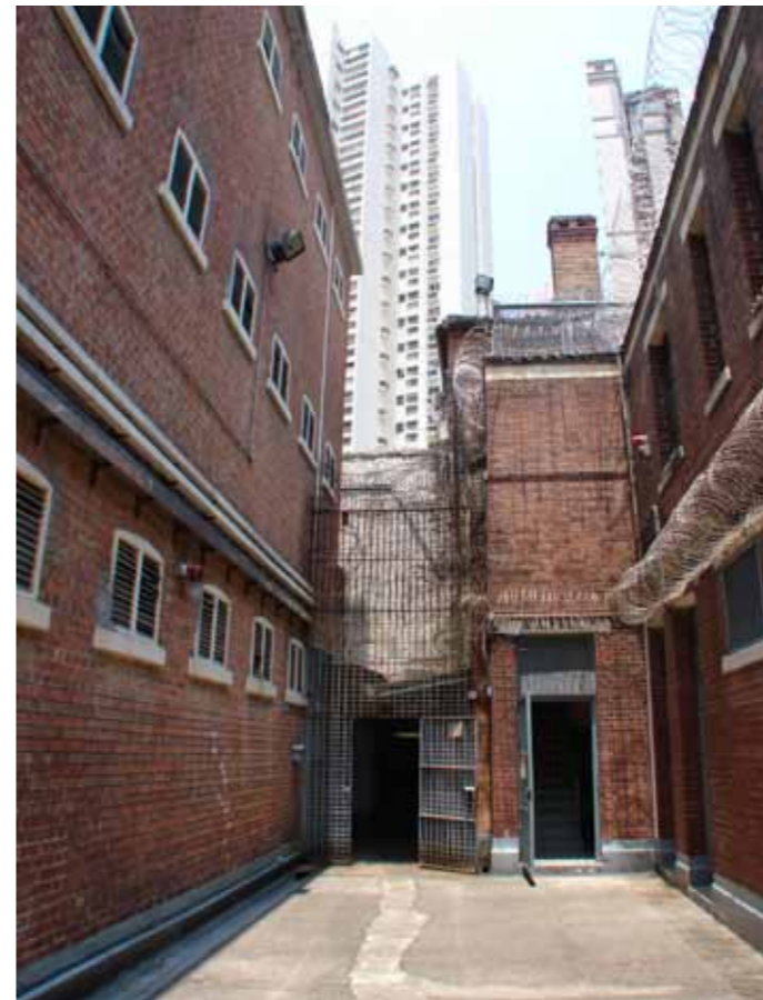
Figure 4 - The area between A and B Halls looking west, B Hall is on the left
