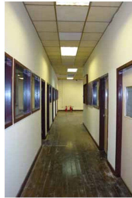
Figure 12 - Former dormitory on the first floor now divided up by modern partitions
