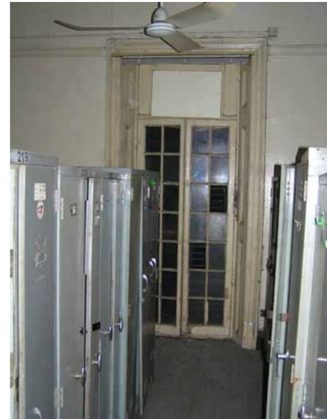
Figure 8 - Double French doors with panelled surrounds
