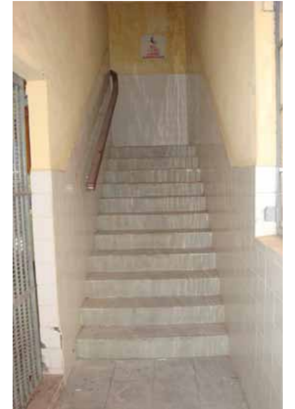
Figure 9 - The southwest stair
