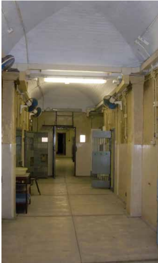
Figure 14 - View of the ground floor corridor of the west wing
