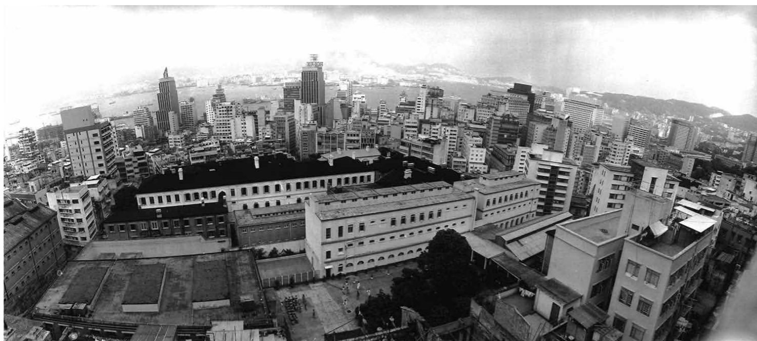
Aerial view of the site in the late 20th century. The south elevation of the Barracks Block is visible.
