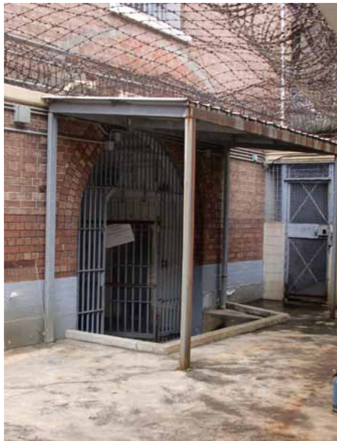
Figure 8 - The ground floor west entrance of the building
