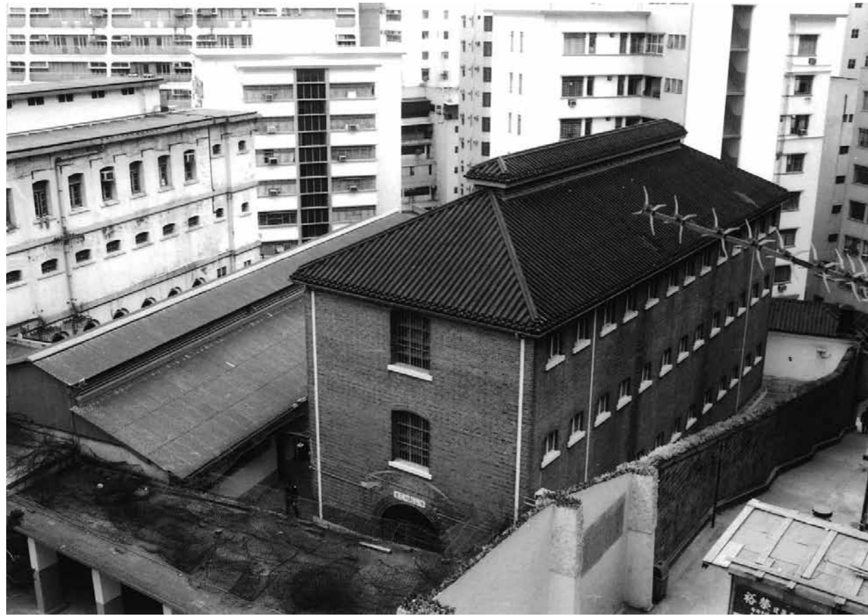
Historic photograph of the building exterior from the southwest
