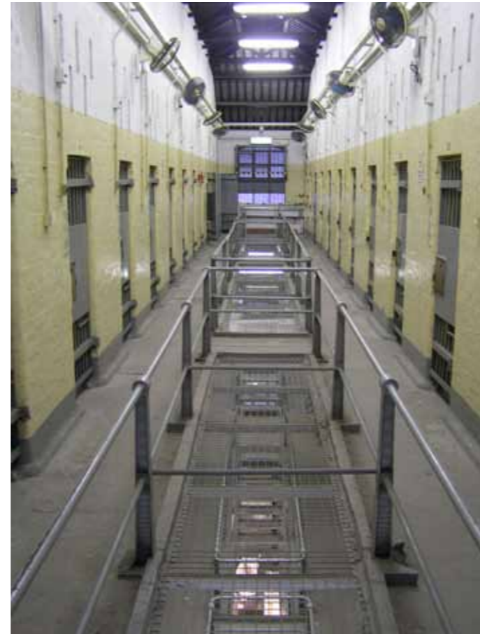
Figure 6 - View of second floor looking west
