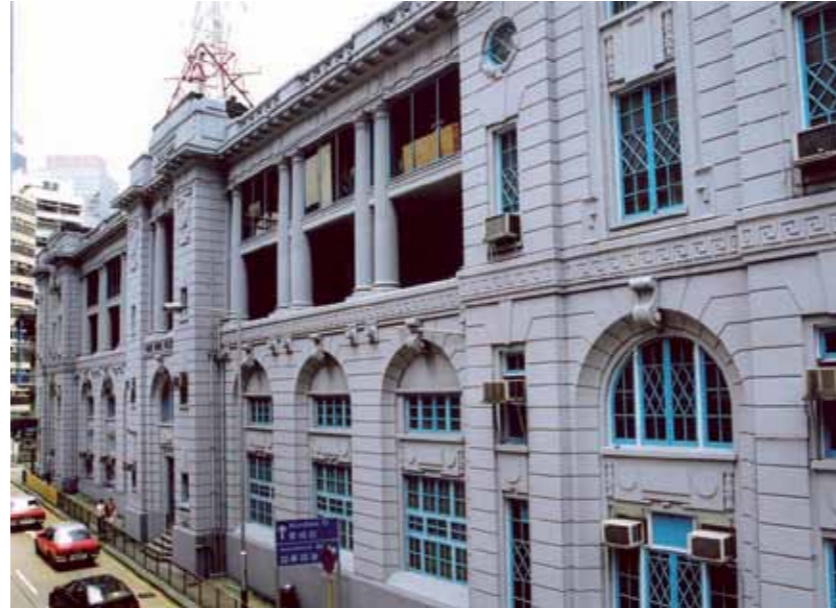
1990s photograph of the north elevation showing the radio mast over the central bay (AMO)
