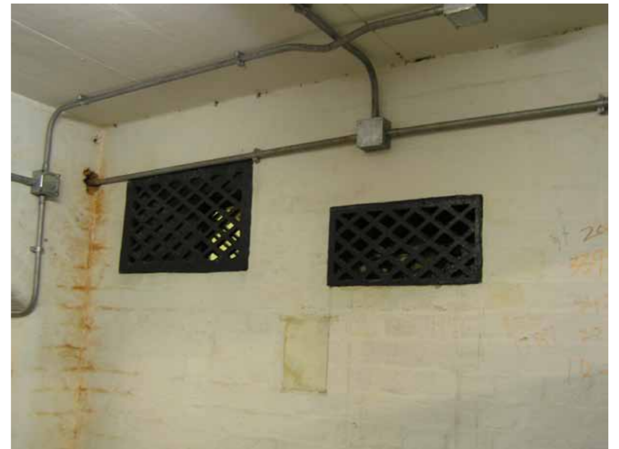
Figure 13 - Lattice ventilation grilles in the basement
