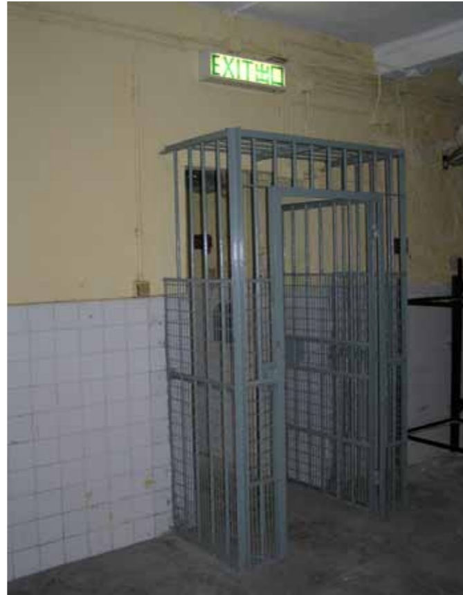
Figure 4 - Internal cage around first floor door
