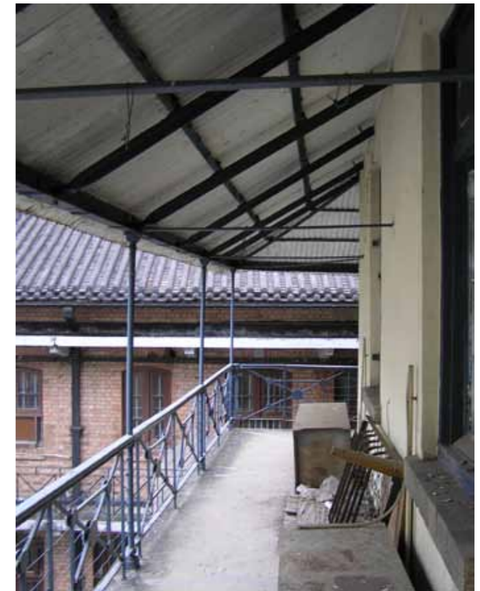
Figure 3 - Balcony on the north side
