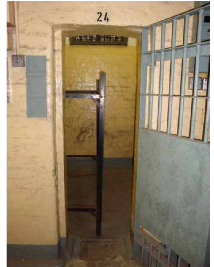
Figure 5 - Interior view of a typical cell
