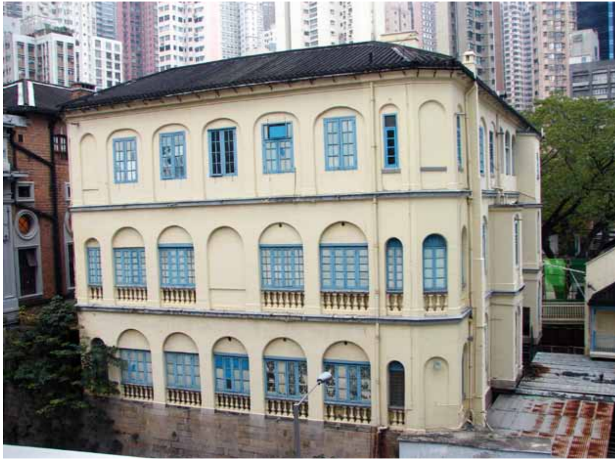
Figure 1 - East elevation overlooking Arbutnot Road; note the ground and first floor verandah infill
