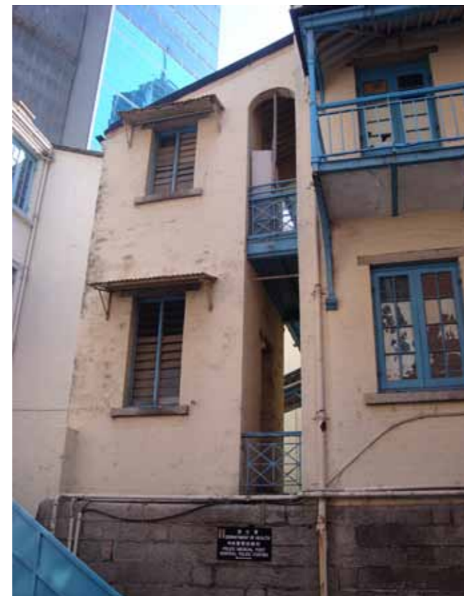
Figure 5 - Bathroom block on the north side
