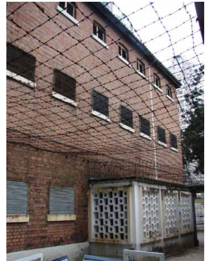
Figure 4 - The entrance to the Laundry, a perforated concrete surround over the stairs; this is adjacent to the north side of E Hall
