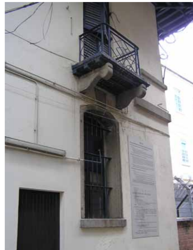
Figure 4 - Ground floor window and first floor balcony on east elevation
