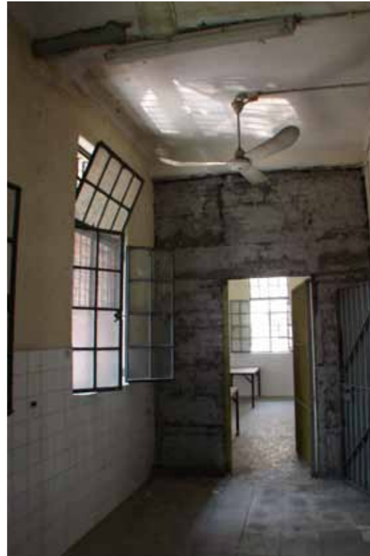
Figure 6 - The first floor west corridor
