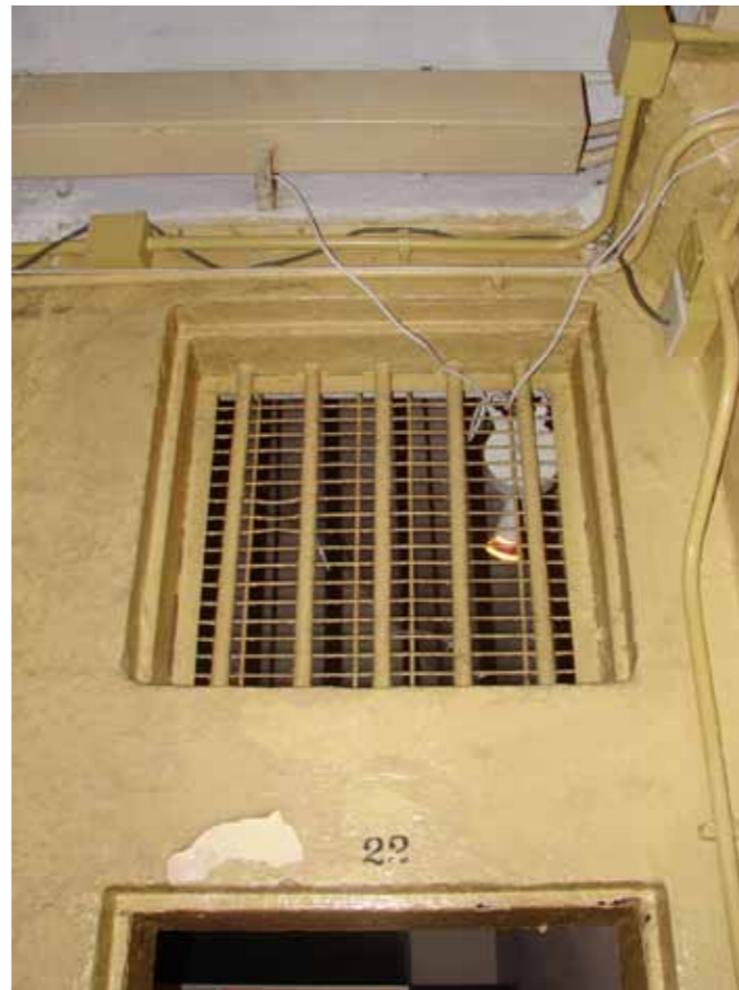
Figure 5 - A ventilation grille in the west wing ground floor
