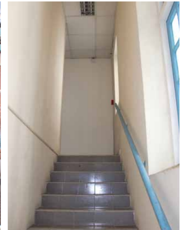
Figure 5 - Existing staircase in the south part of the building
