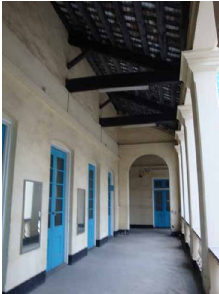
Figure 5 - Third floor verandah with exposed ceiling structure
