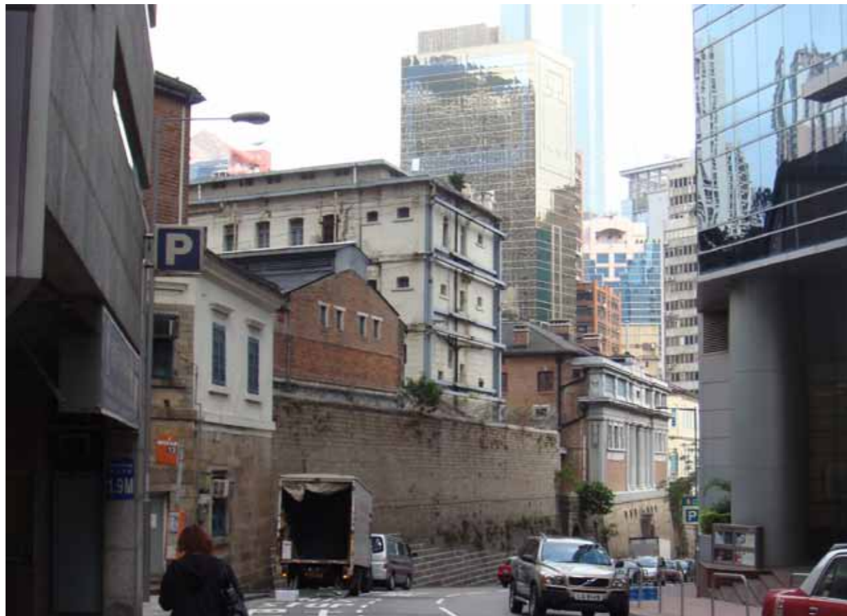
Figure 2 - South elevation of the west wing and west extension
