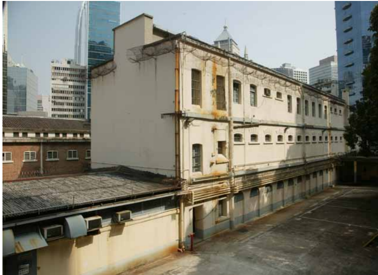
Figure 1 - View of the west wing, east and south elevations, as seen from Arbutnot Road
