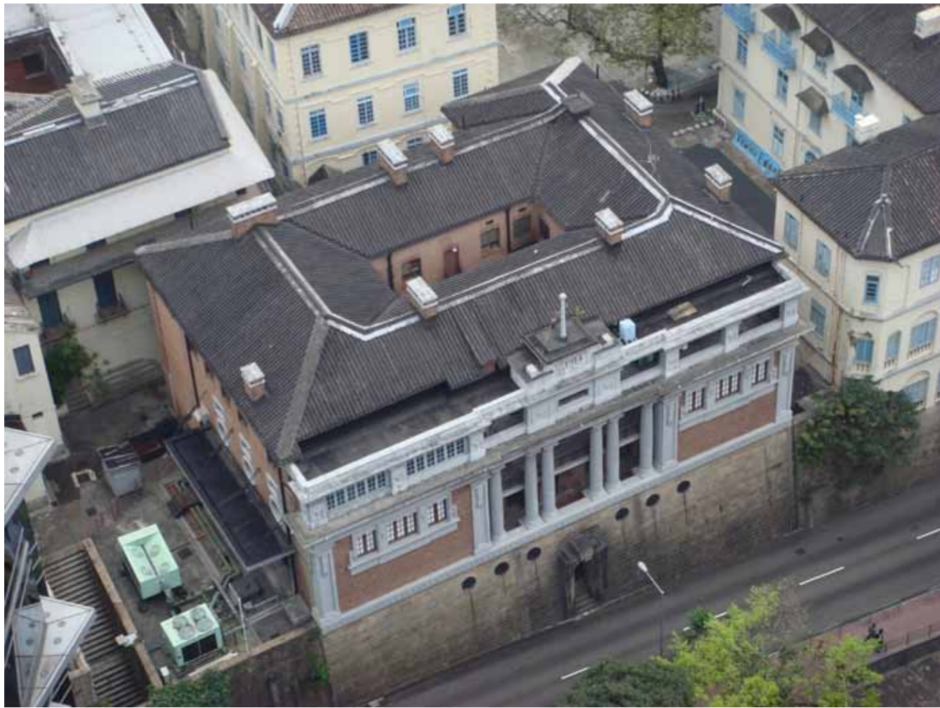
Figure 1 - Aerial view of the Magistracy, taken from the east
