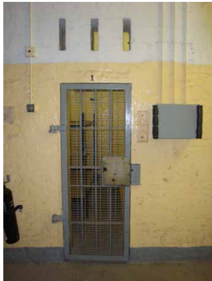
Figure 8 - A typical cell door in the west wing first floor
