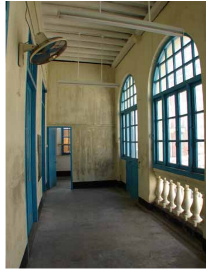
Figure 7 - Typical north verandah
