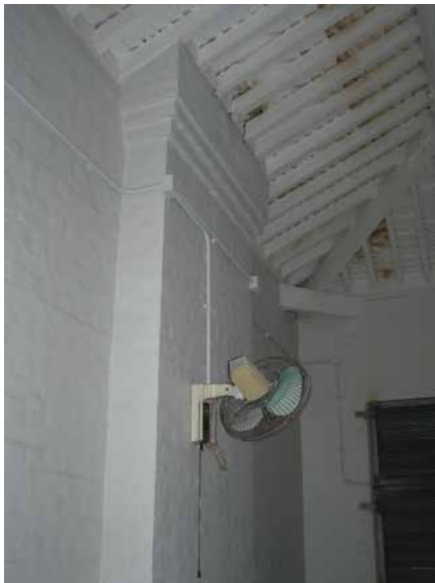
Figure 5 - First floor brick chimney breast
