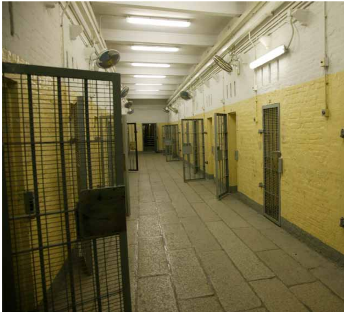
Figure 10 - The first floor west wing
