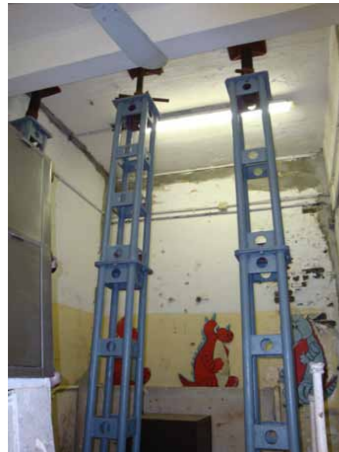
Figure 20 - Steel supports in the east wing first floor
