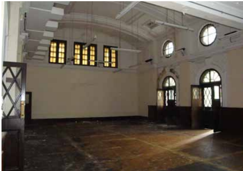
Figure 15 - Ground floor South Court
