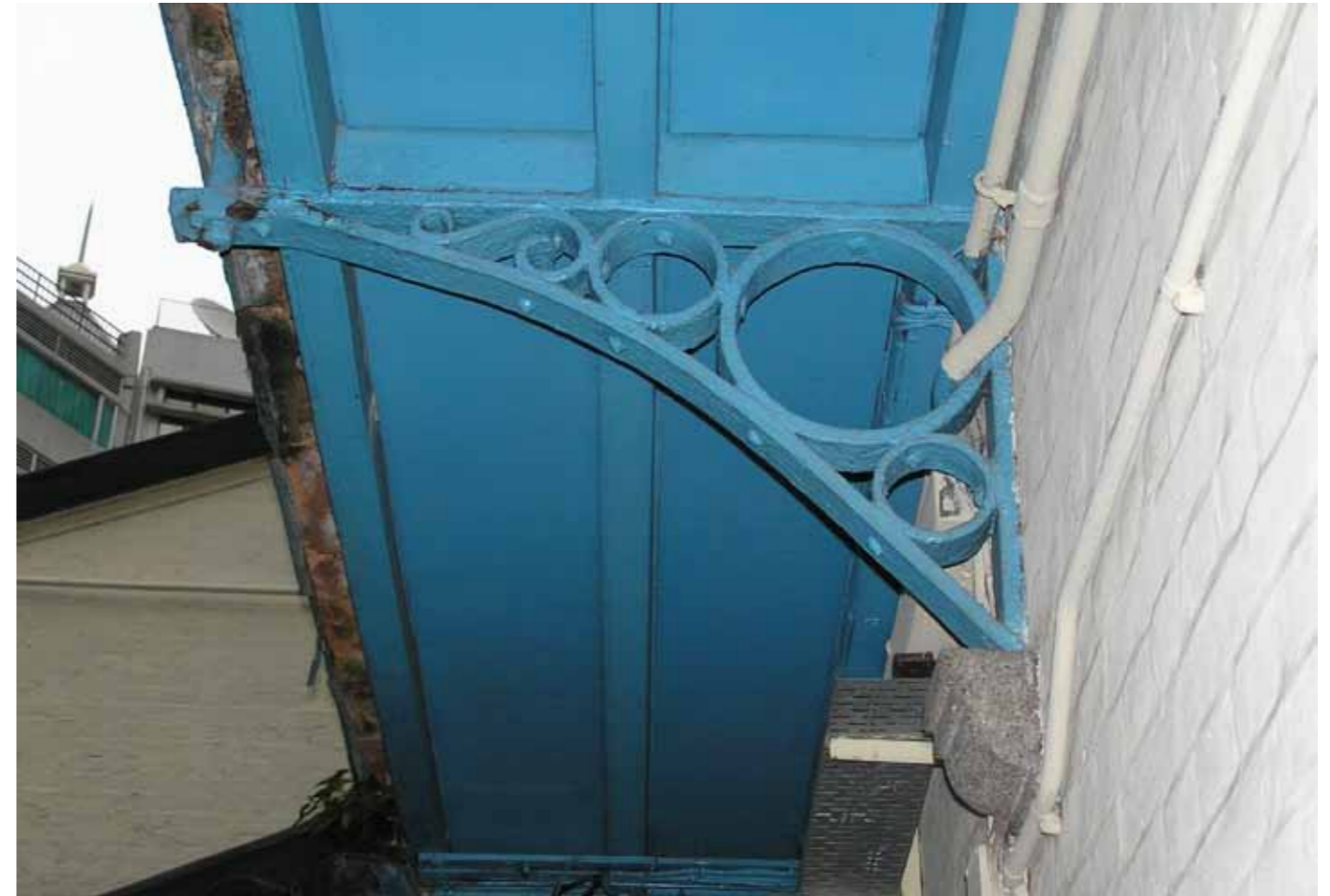
Figure 2 - Detail of the north balcony bracket and corbels
