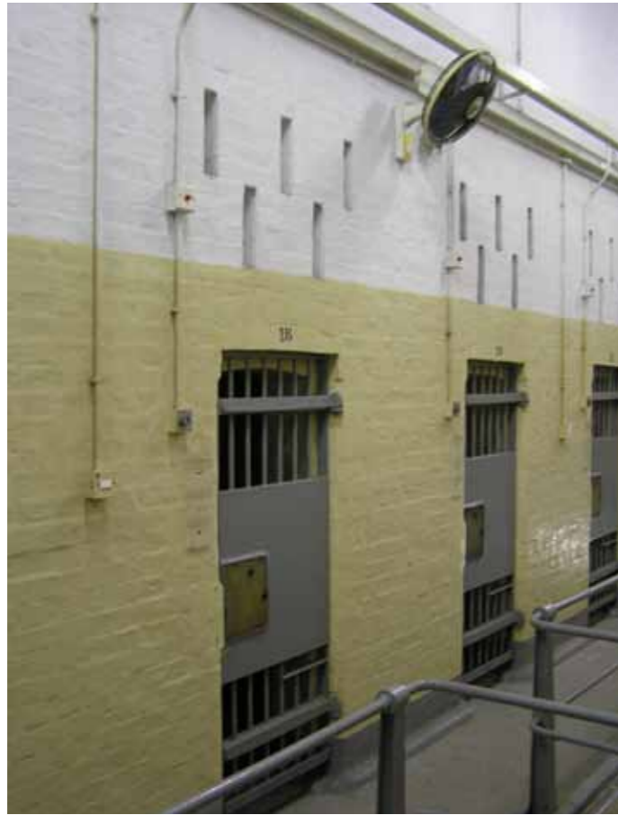
Figure 5 - A row of cells on the first floor
