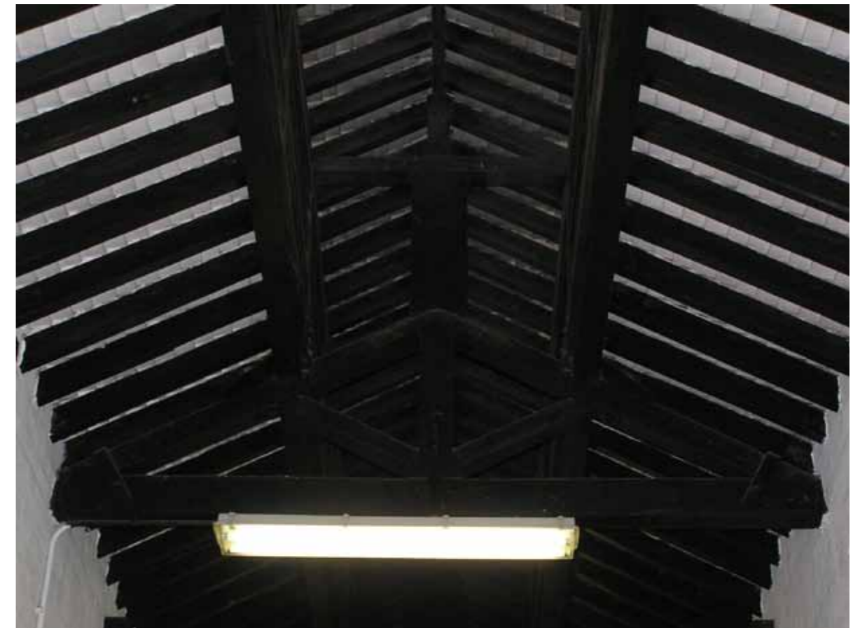
Figure 10 - The original timber frame roof
