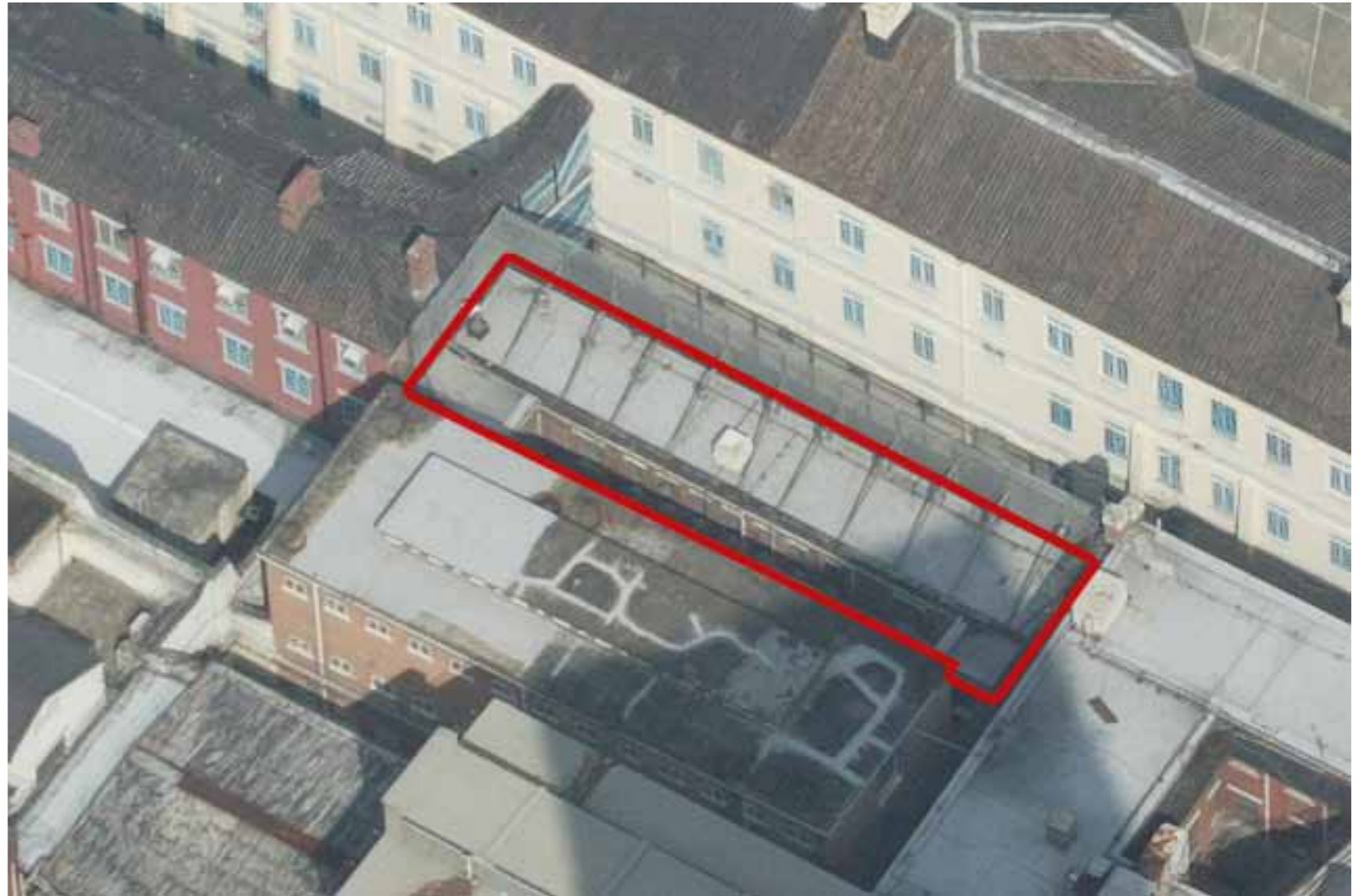
Aerial photograph of the building outlined in red, with north to the top of the image
