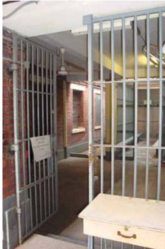
Figure 5 - Barred doors on west side of building leading into ground floor
