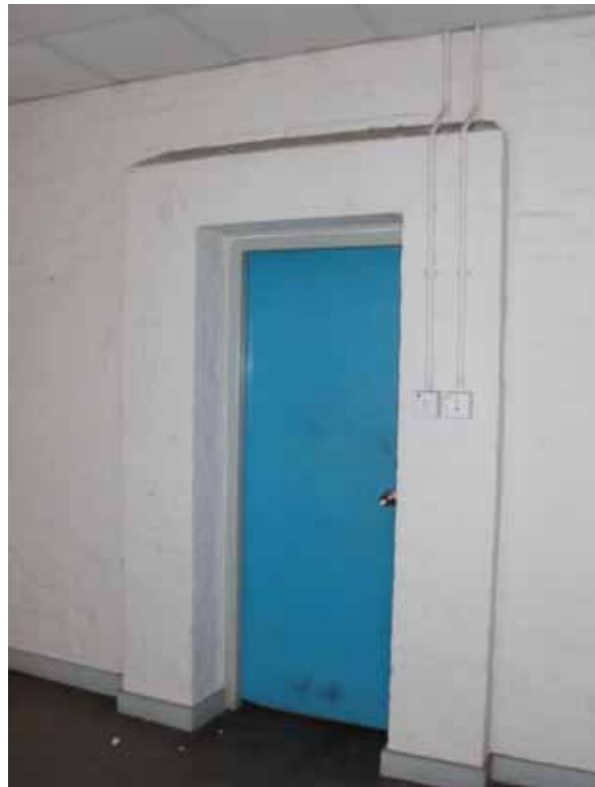
Figure 8 - Door into room 02/F/09
