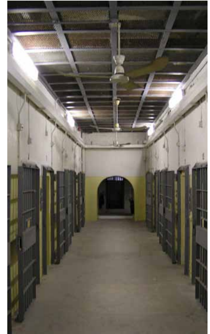
Figure 17 - Basement of the east wing
