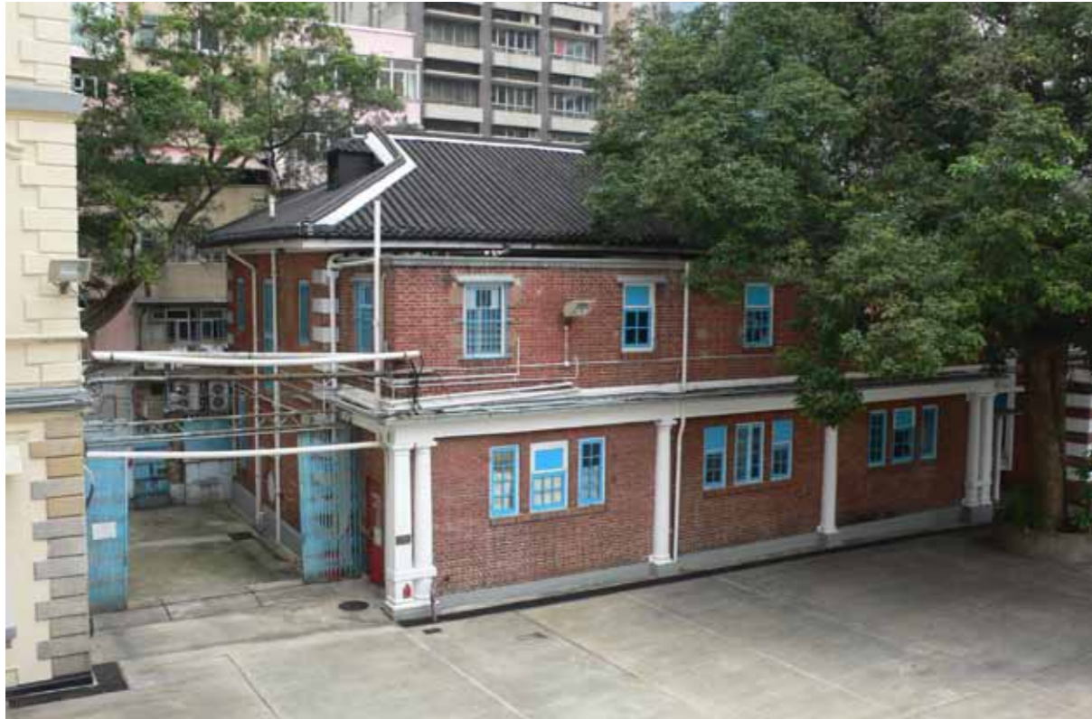
Figure 1 - East (Parade Ground) elevation showing the infilled ground floor arcade and the poor quality first floor addition
