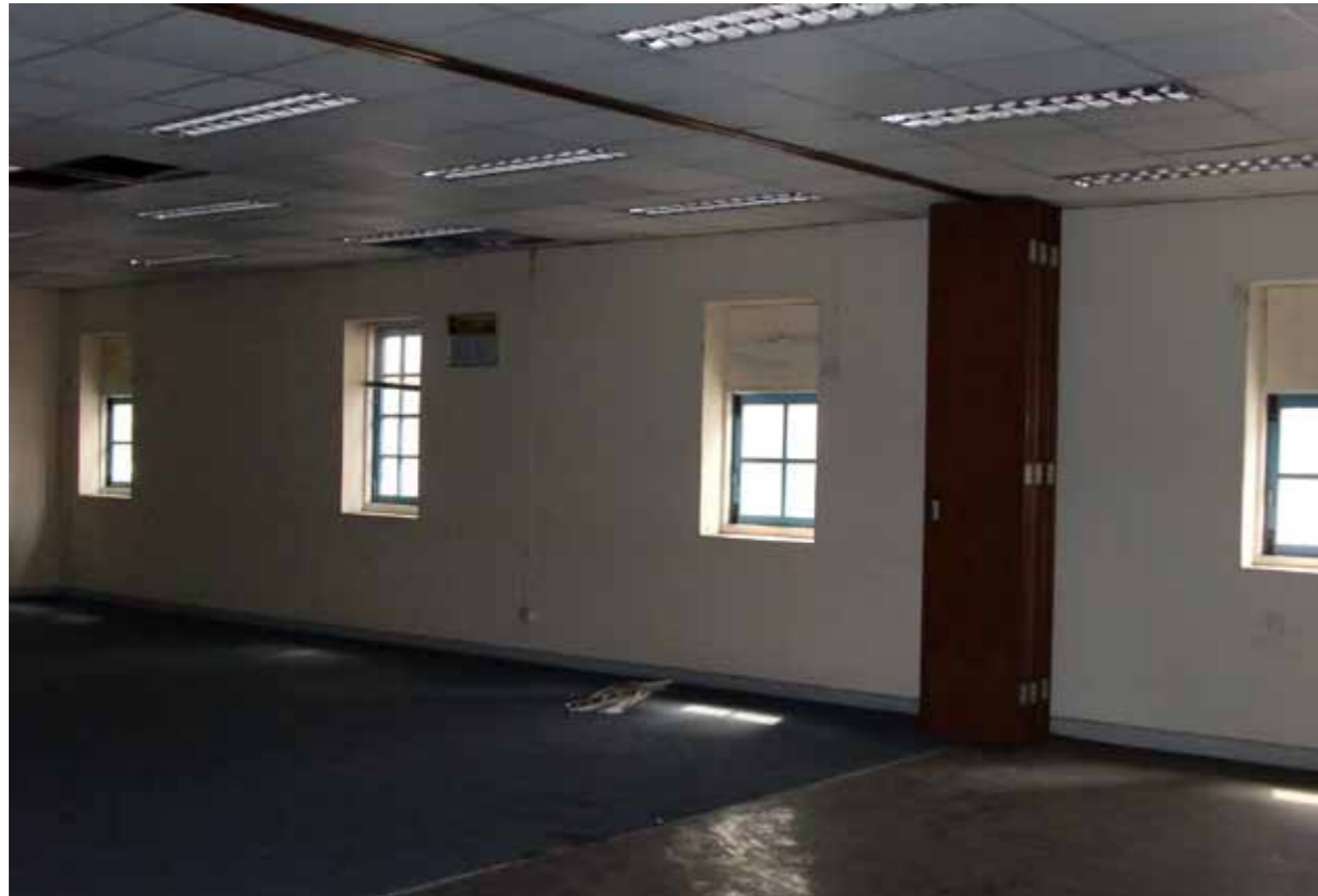
Figure 6 - First floor interior as fitted out for its final use by the Traffic Police
