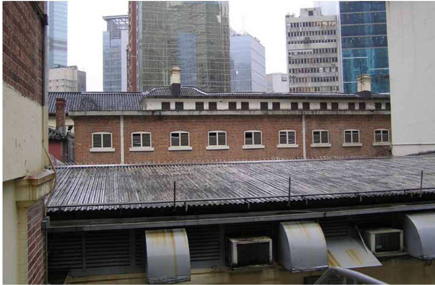
Figure 1 - View of the top floor from the south
