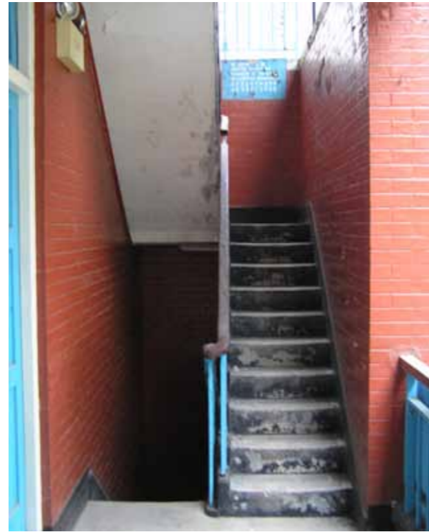
Figure 3 - The main stairs at the west end
