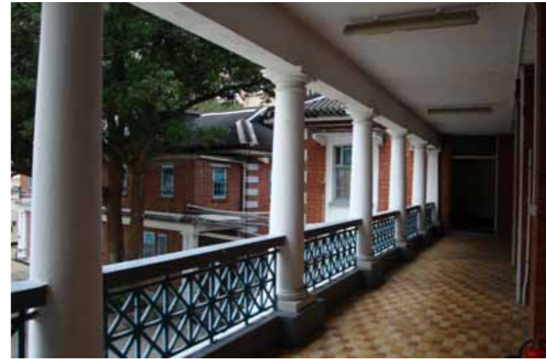
Figure 5 - Verandah on the south side, first floor
