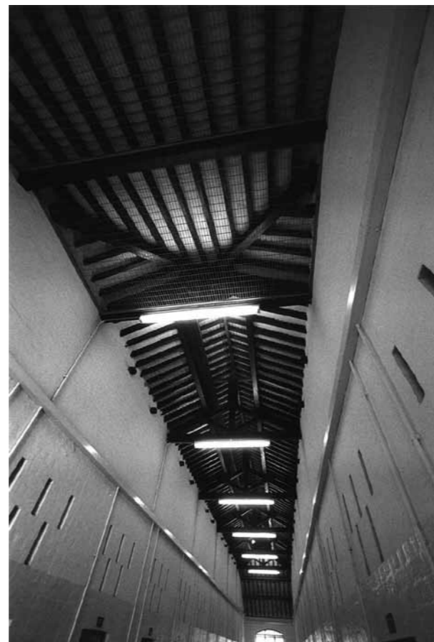
Historic photograph of the roof
