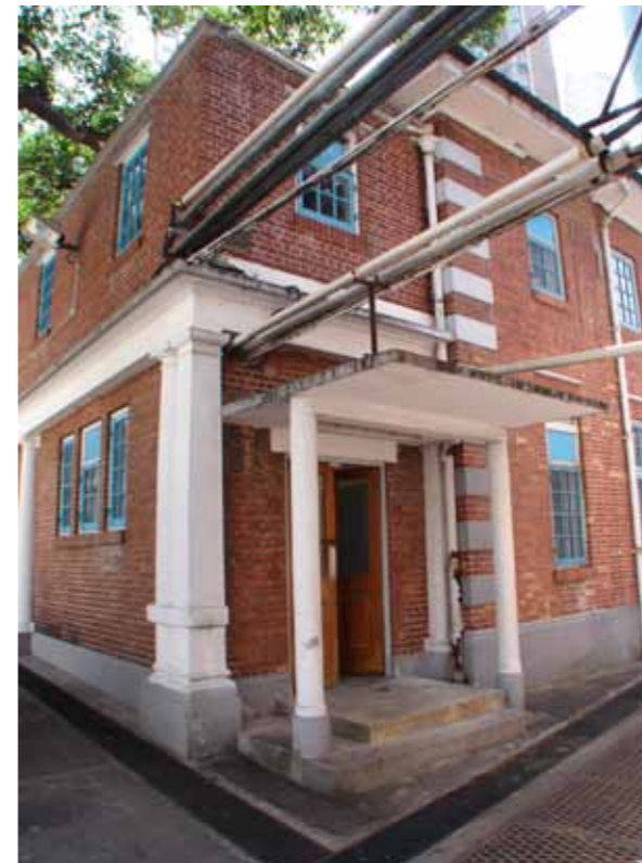
Figure 4 - Canopy on north elevation
