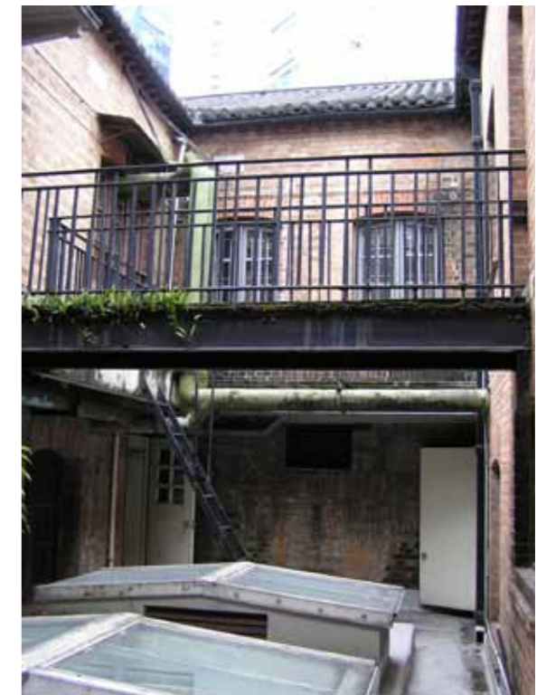
Figure 7 - View of the courtyard
