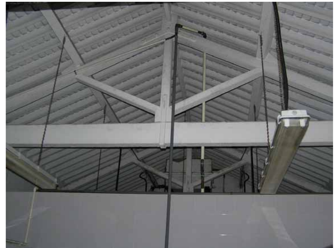
Figure 7 - View of the original timber frame roof
