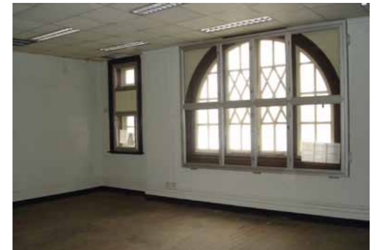
Figure 9 - View of the northwest room of LG2
