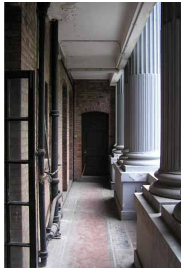
Figure 12 - Ground floor east verandah
