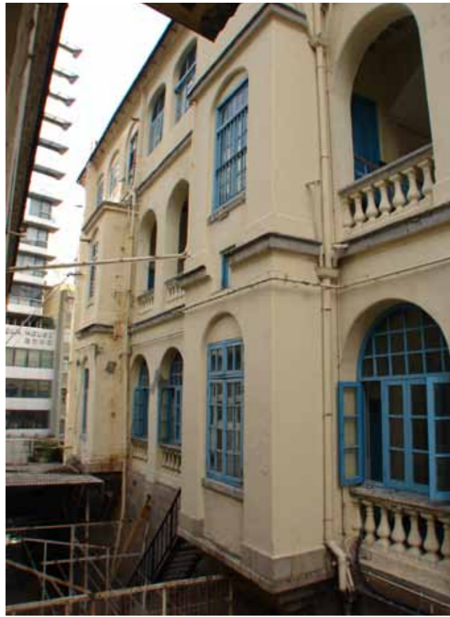
Figure 5 - North elevation detail showing projecting bay
