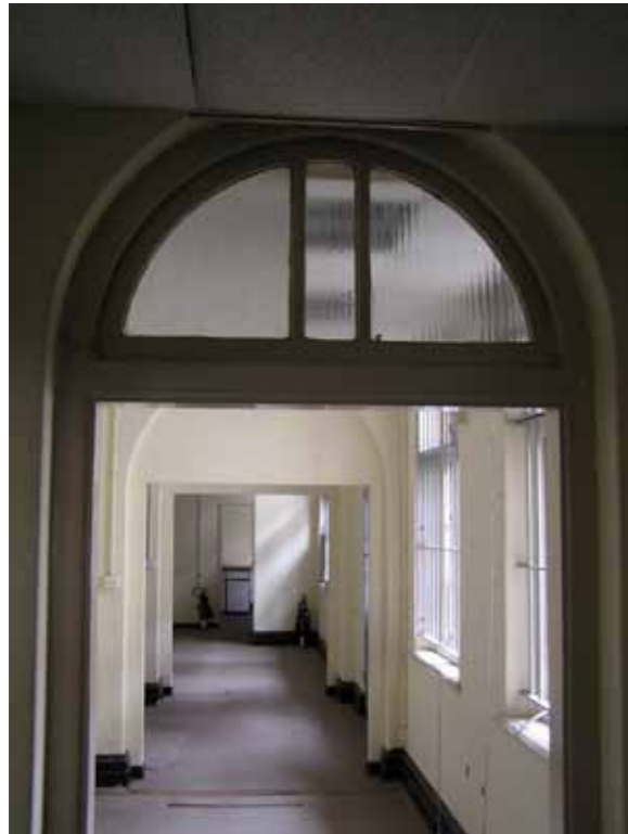
Figure 8 - First floor arched opening
