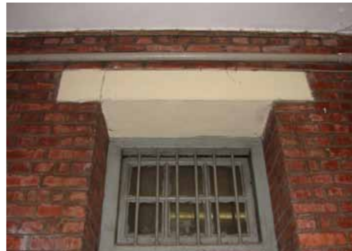
Figure 11 - Detail view of the door lintels at ground floor level
