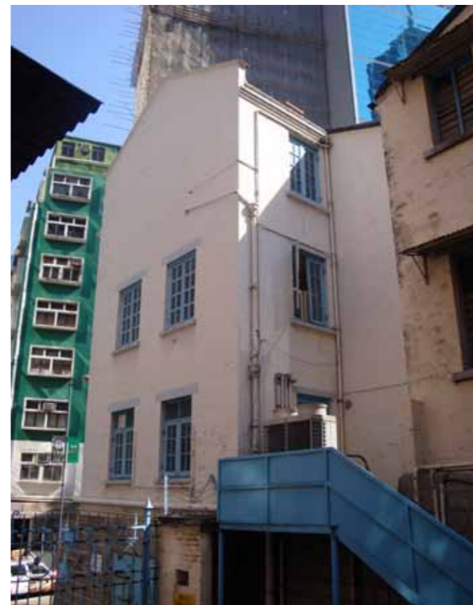
Figure 3 - West elevation overlooking the Pottinger Street entrance
