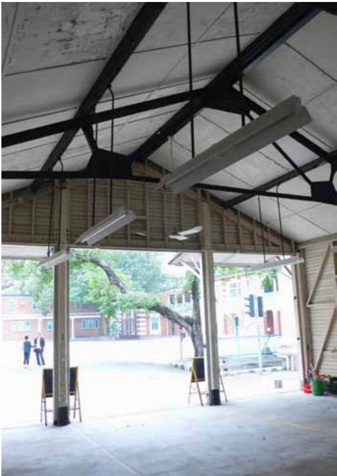
Figure 3 - View of the interior looking west
