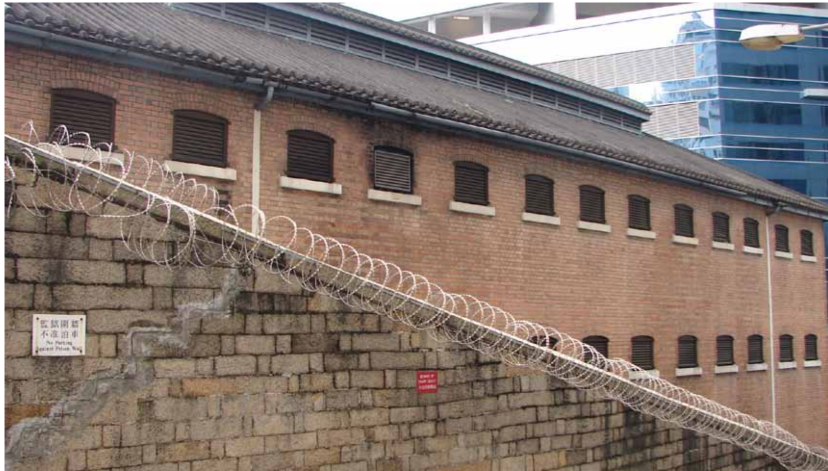
Figure 1 - View of the south elevation behind Chancery Lane boundary wall
