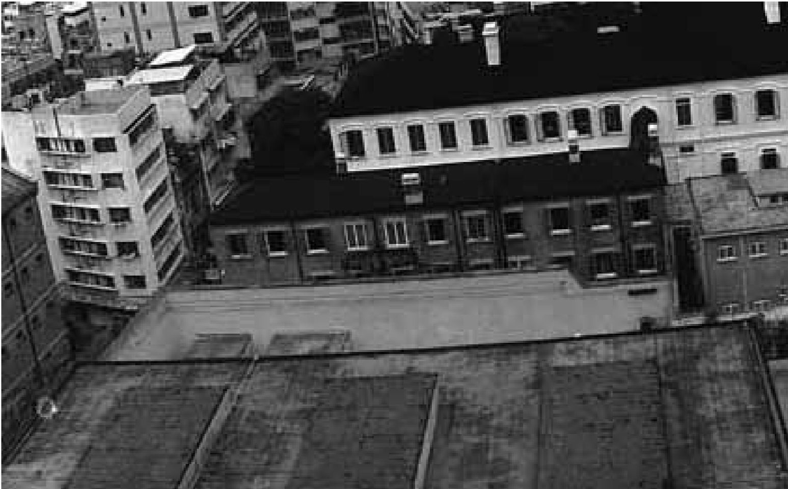
Aerial view of the south side of the building c1970s
