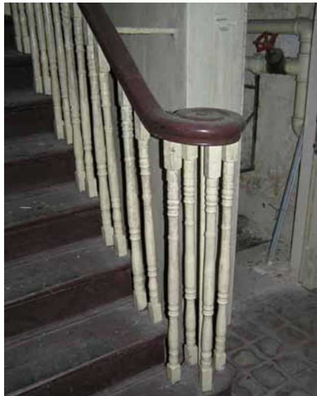
Figure 9 - Main staircase balustrade and moulded timber handrail, as viewed on the ground floor.
