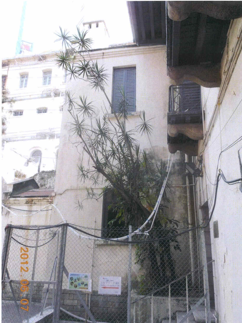
Fig. 6 Overall view of Tree-11 during inspection on 7 th June 2012.
