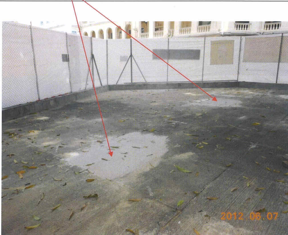
Fig. 5 Two trial pits have been reinstated prior to inspection.
