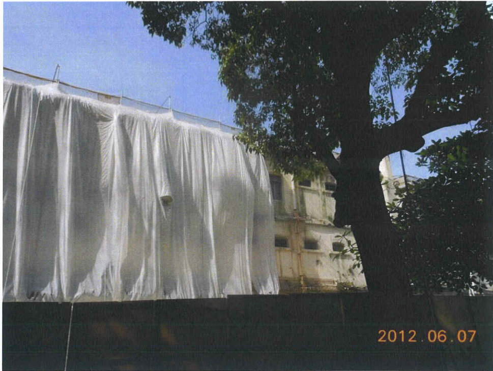
Fig. 6 Overgrown branches/leaves had been pruned on 1 st June 2012.
