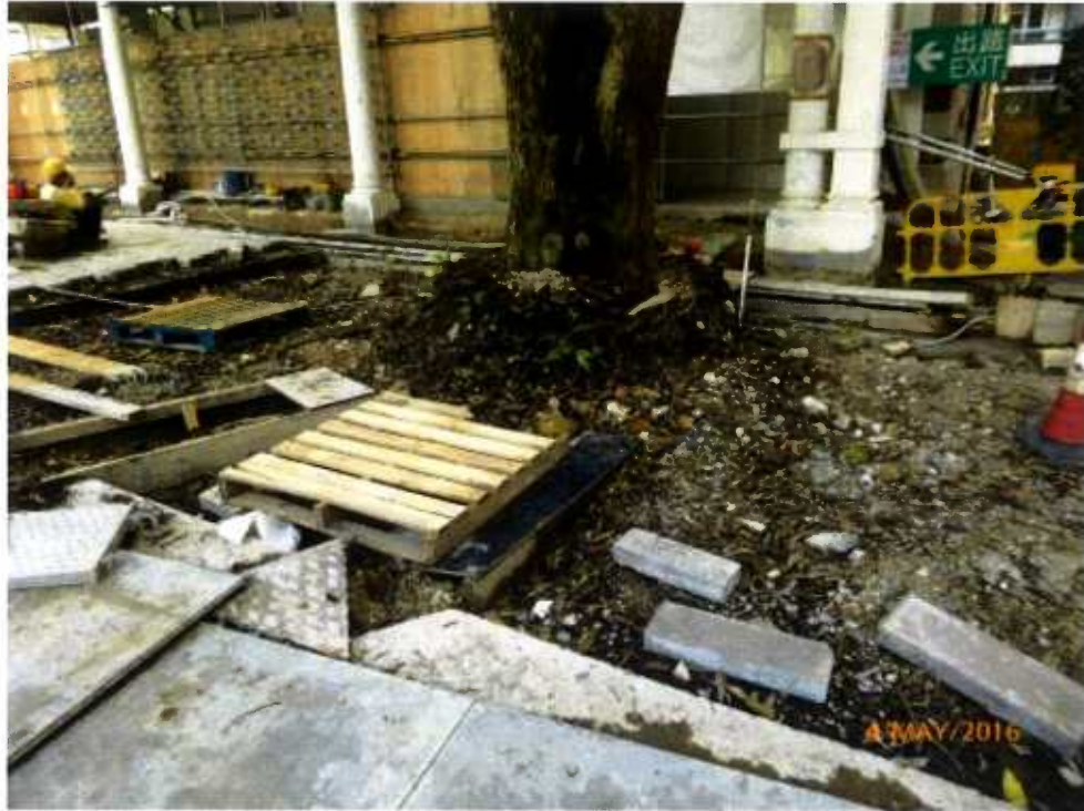
Fig. 10 Renovation work is in progress near the tree.
