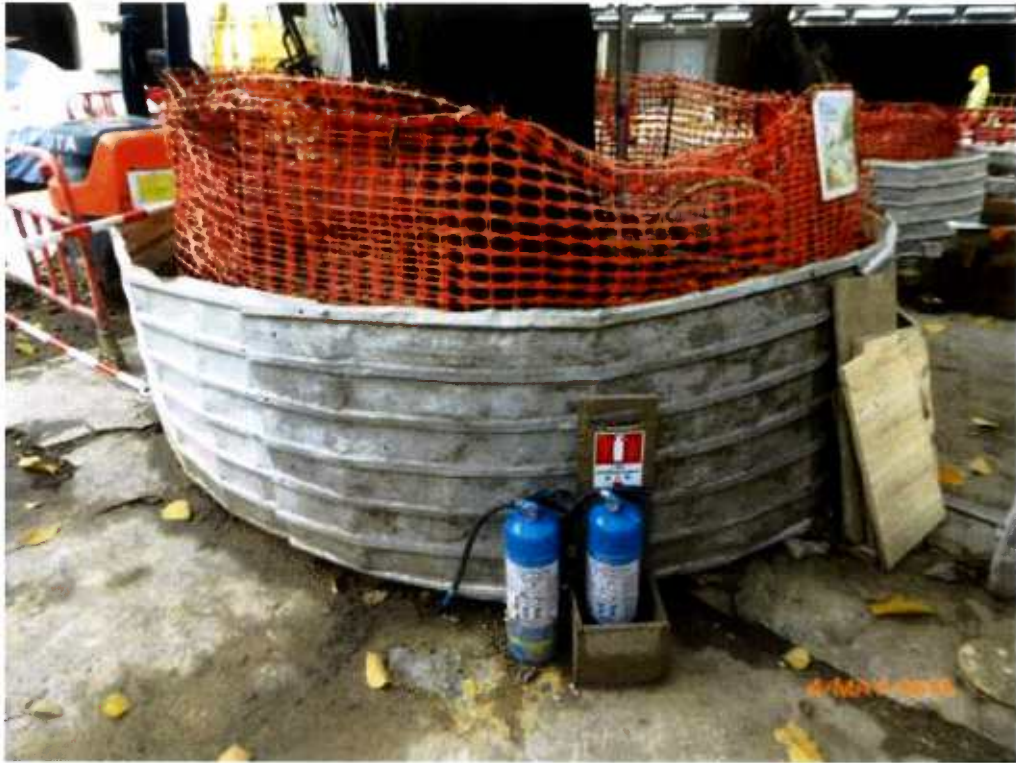
Fig. 10 The small cordon zone is in order.
