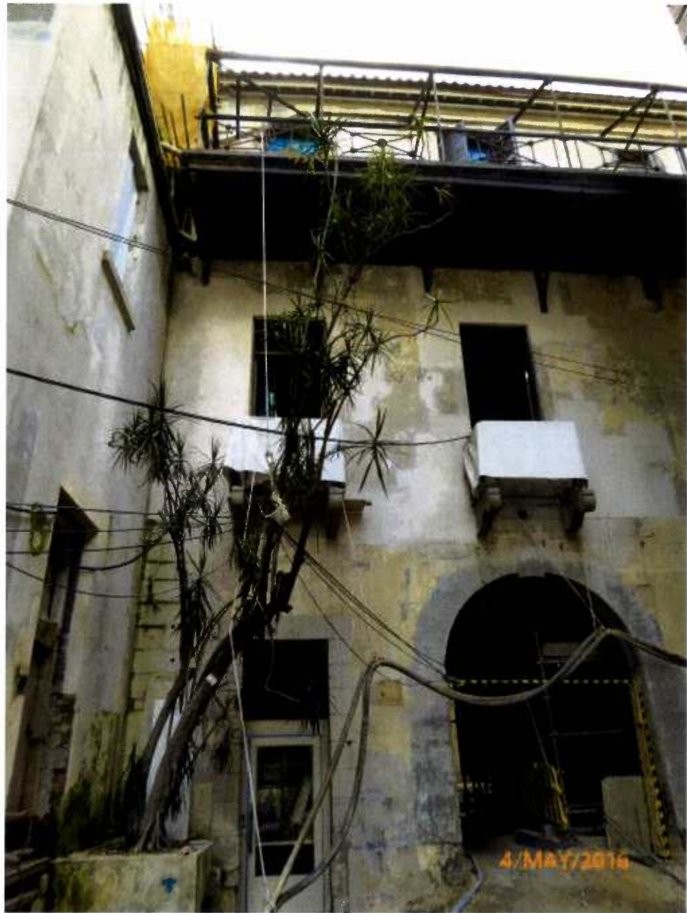
Fig. 12 Overall view of Tree 11 during inspection on 4 th May 2016.
