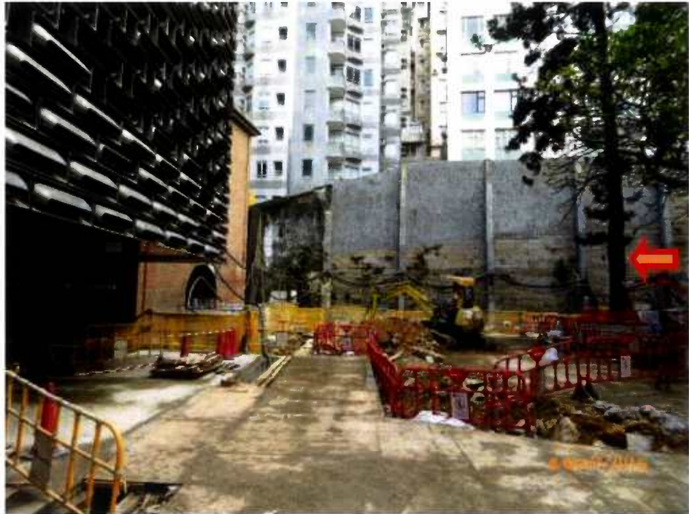
Fig. 10 Construction works are in progress near Tree-9.
