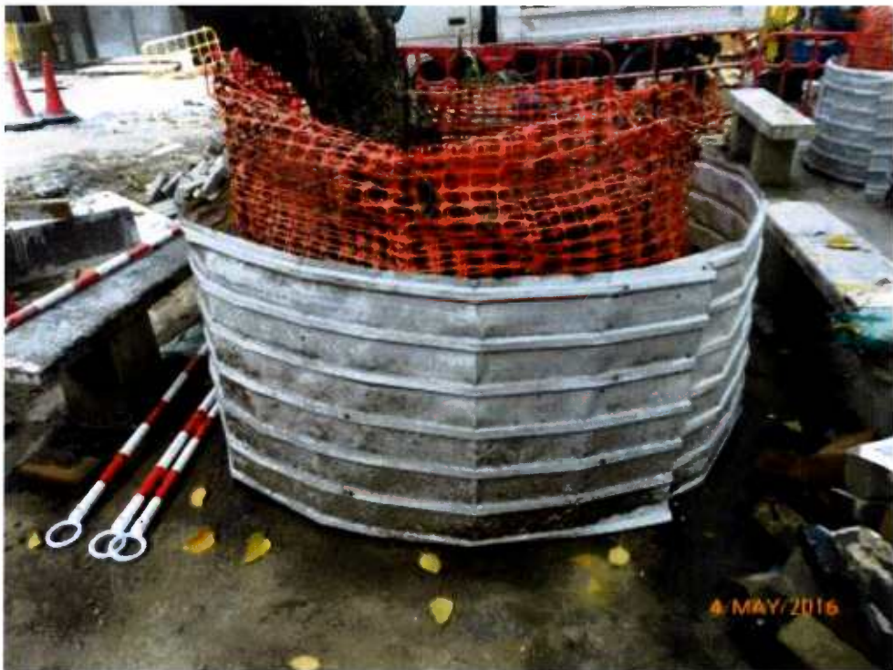
Fig. 9 The small cordon zone is in order.
