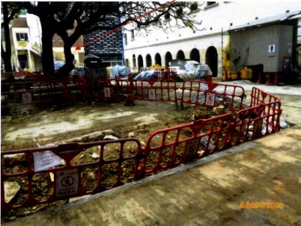
Fig. 11 Construction works are in progress near Tree-8.
