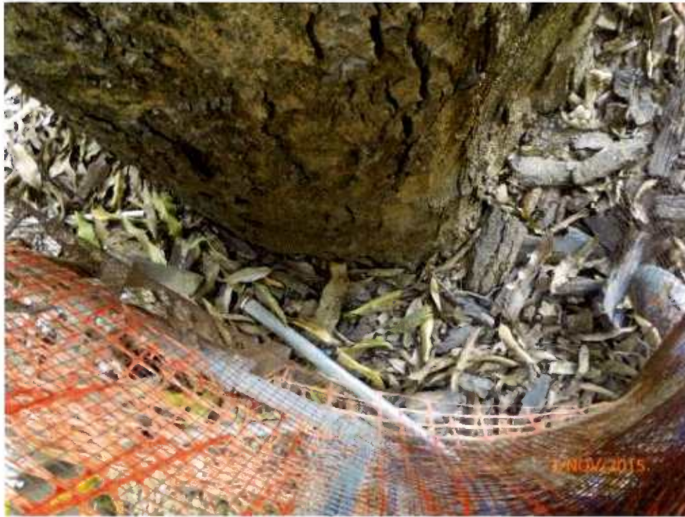
Fig 2. Root collar of Tree-5 is normal. The planter appears clean and tidy.
