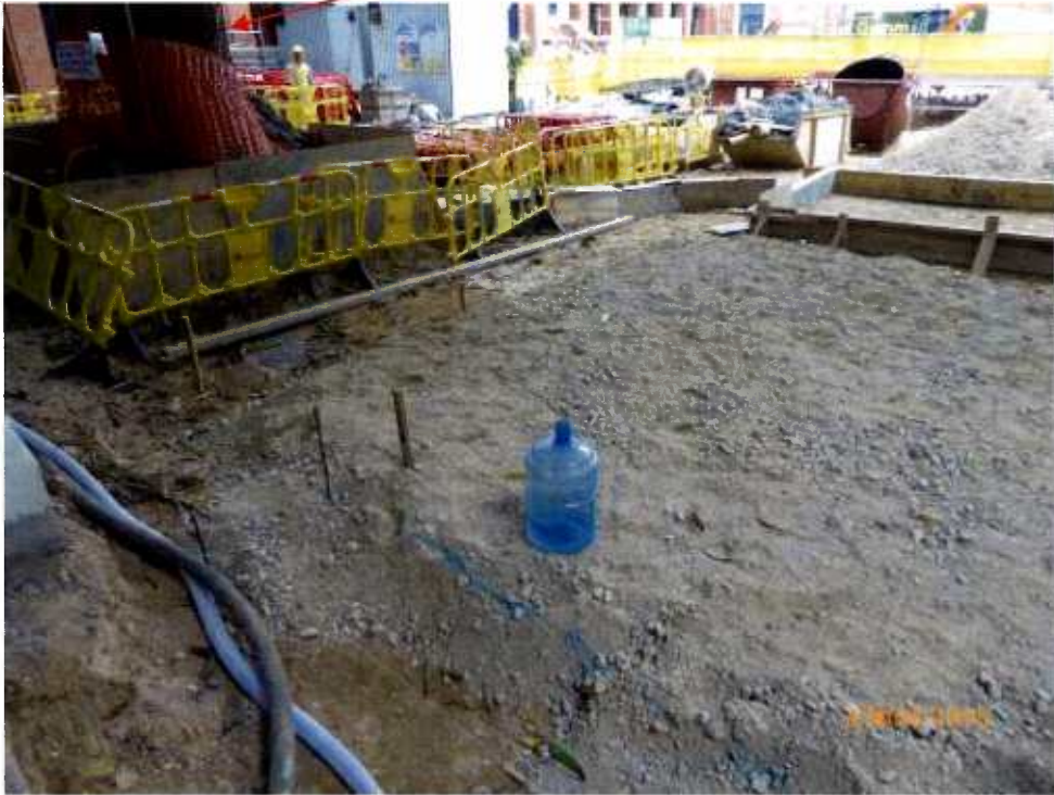
Fig. 8 Renovation work is in progress near Tree-5.
