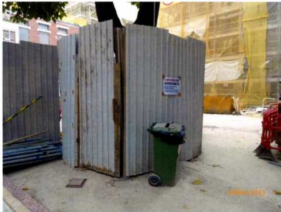
Fig. 7 The planter is surrounded by some metallic sheets to act as cordon zone.
