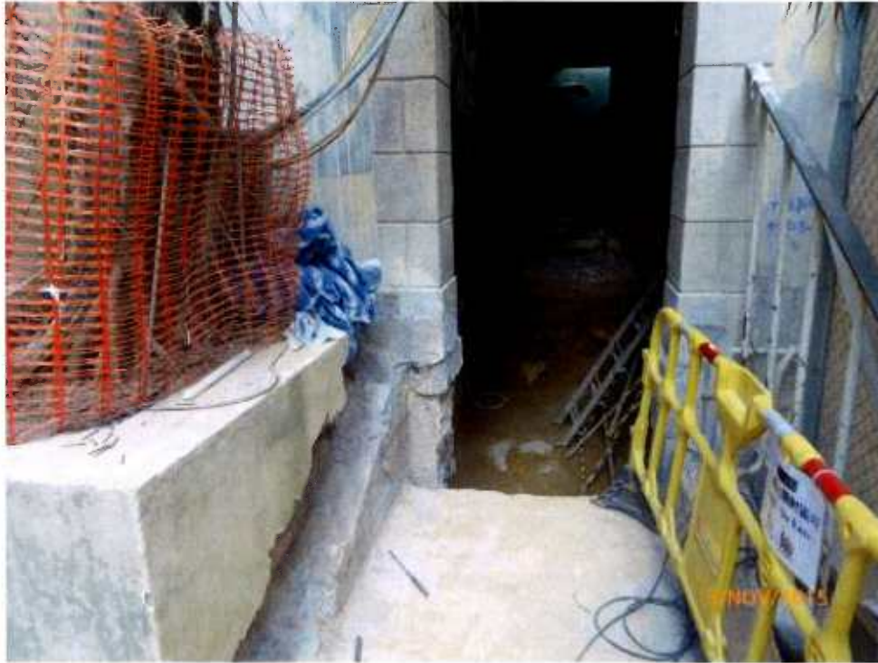
Fig. 8 Renovation work is in progress near the planter.
