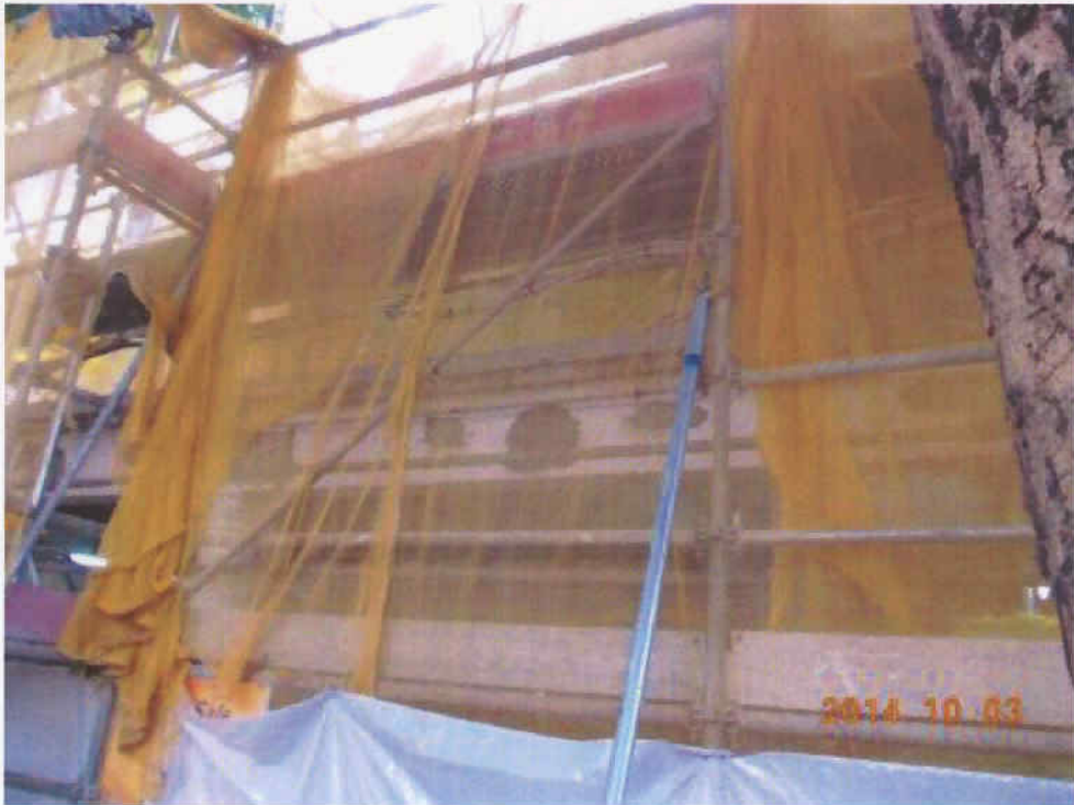
Fig. 7 Renovation work is in progress near the tree.
