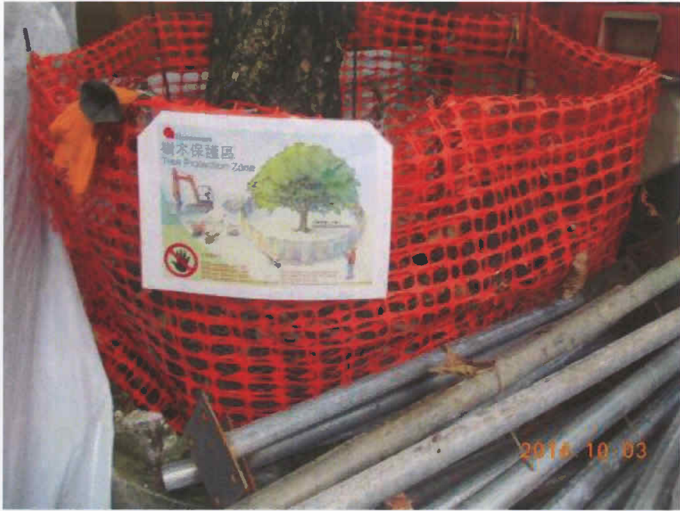
Fig. 6 The small cordon zone is in order.
