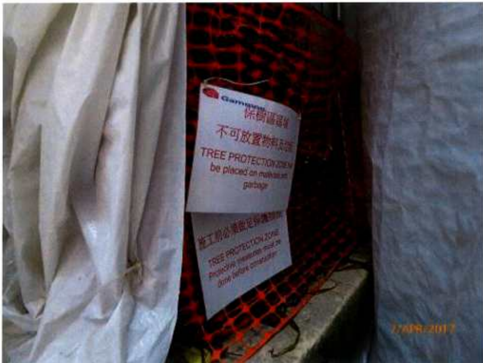
Fig. 9 Tree protection zone is in order at the time of inspection.
