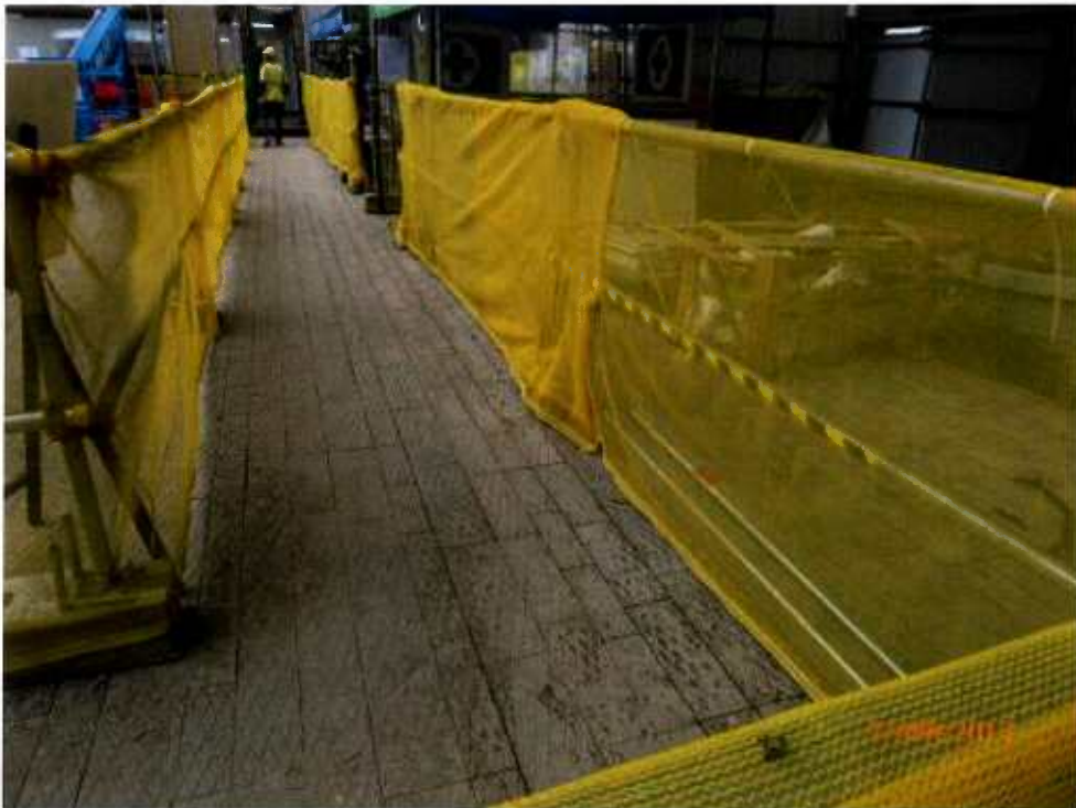
Fig. 11 The access near Tree-5 also is clean and tidy.
