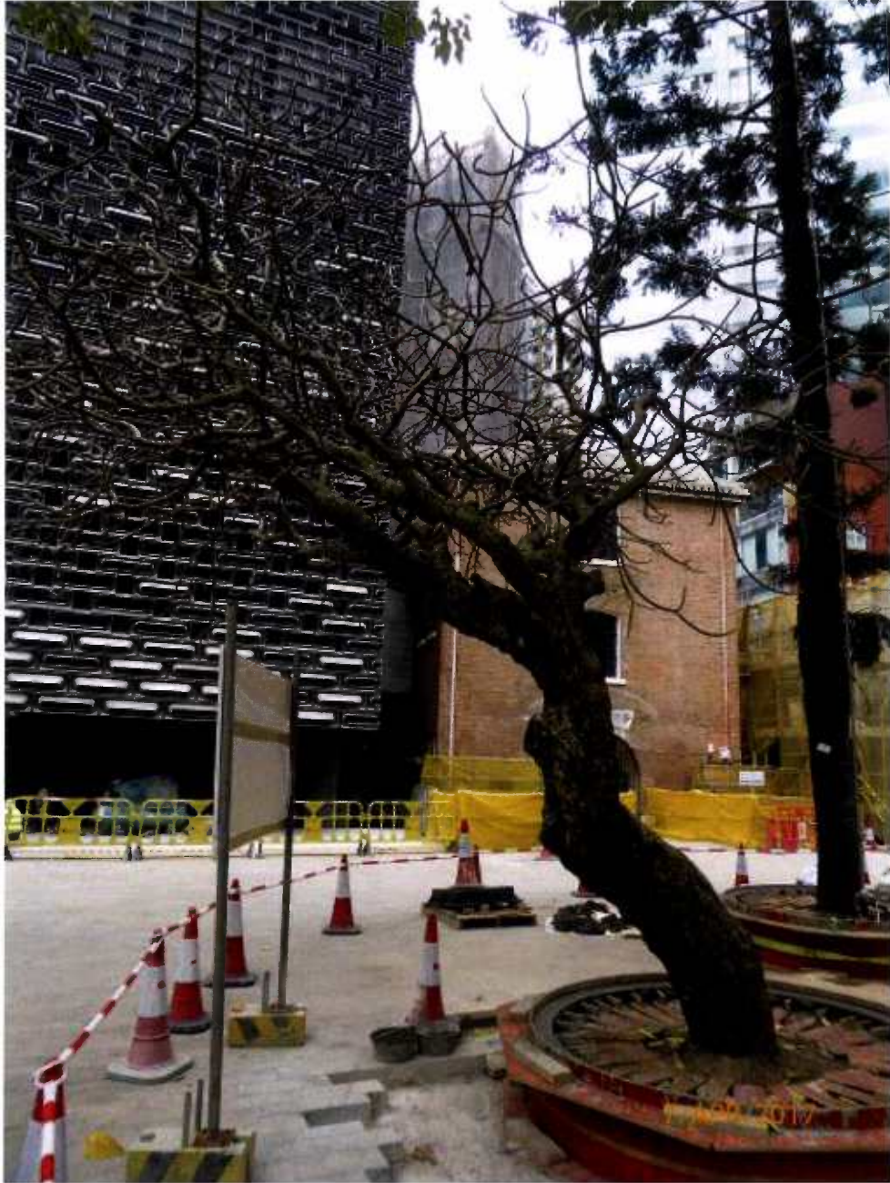
Fig. 10 Overall view of Tree-8 during inspection on 7 th April 2017.
