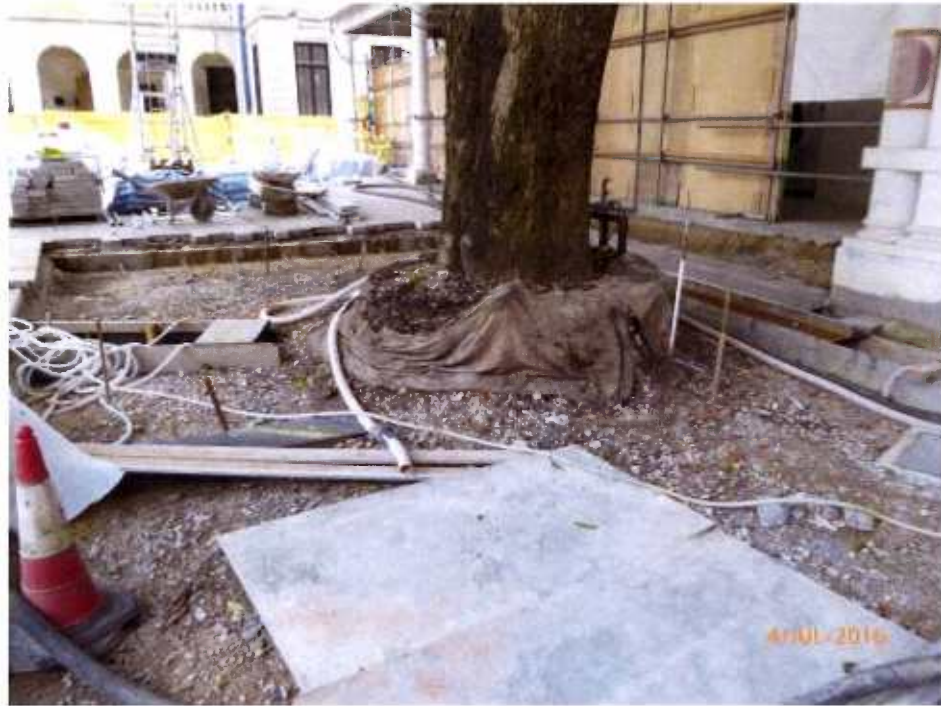
Fig. 10 Construction works are in progress near Tree-5.
