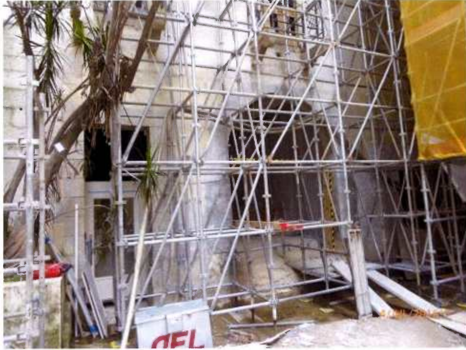
Fig. 10 Construction works are in progress near the tree.
