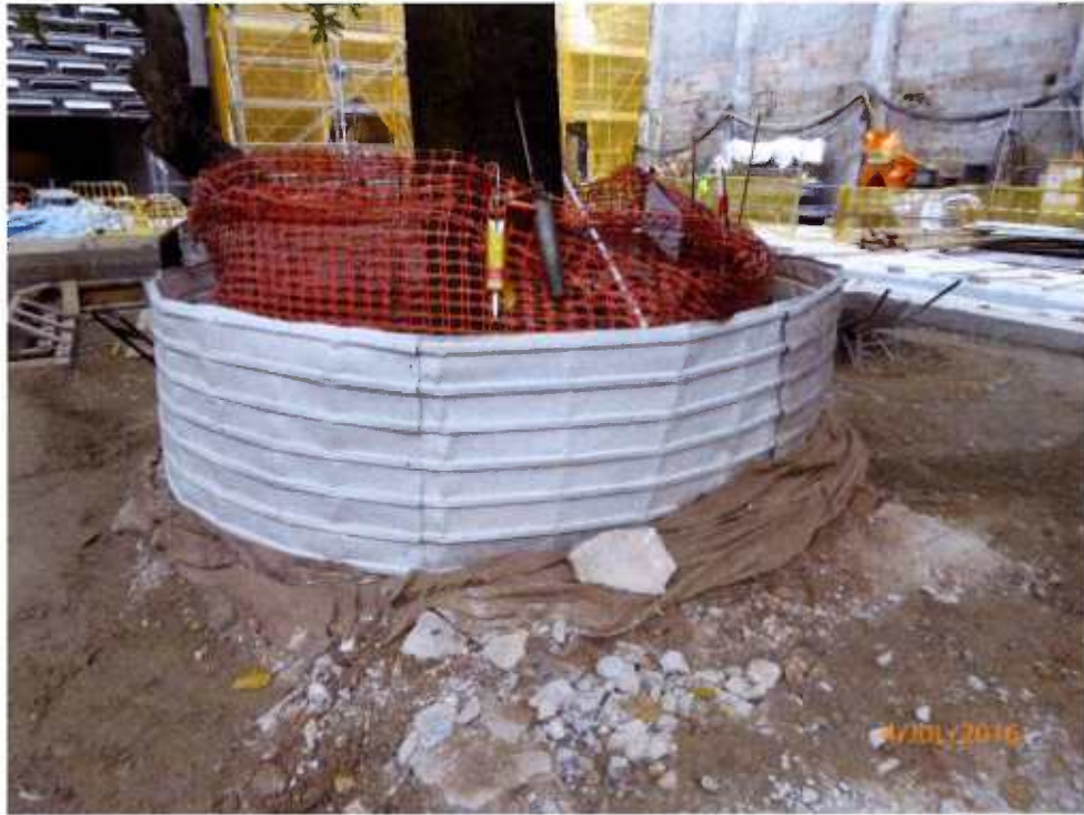
Fig. 10 The small cordon zone is in order.
