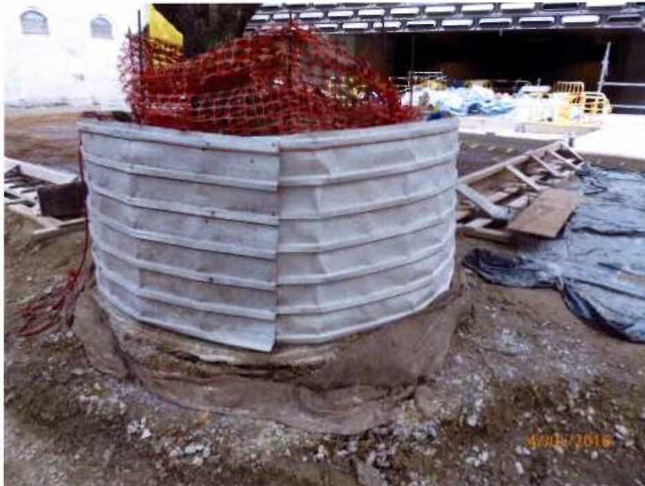
Fig. 9 Small cordon zone is in good order.
