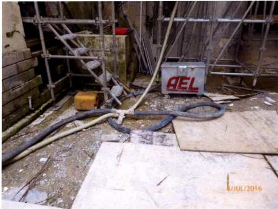
Fig. 11 Cleanliness of the site near Tree 11 is acceptable.
