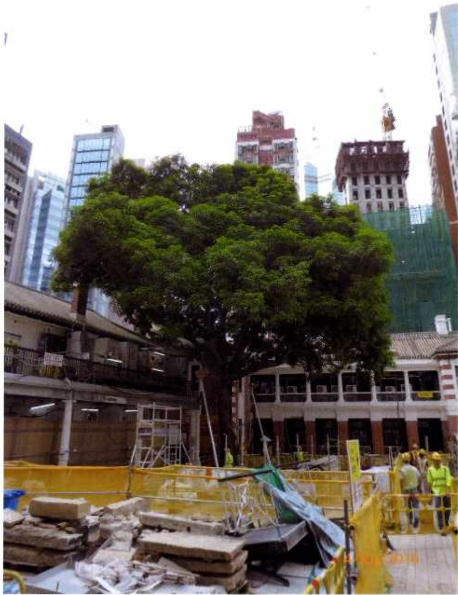
Fig. 12 Overall view of Tree-5 during inspection on 4 th July 2016.
