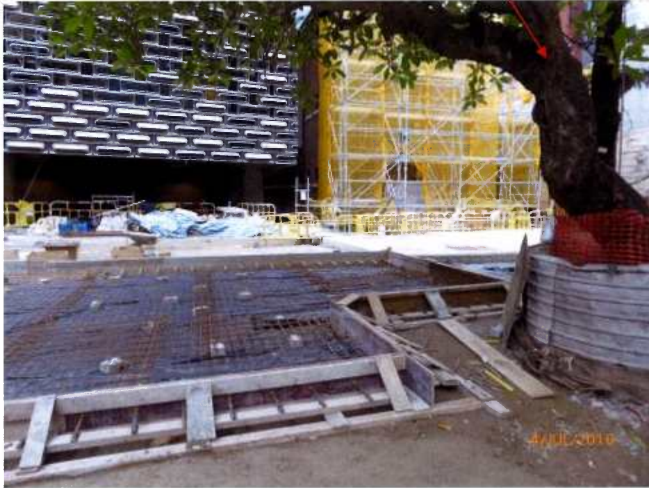
Fig. 10 Construction works are in progress near Tree-8 .
