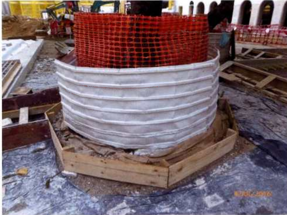
Fig. 8 Small cordon zone is in good order.
