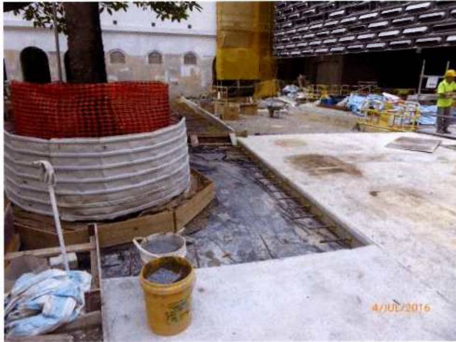
Fig. 10 Construction works are in progress near Tree-9.
