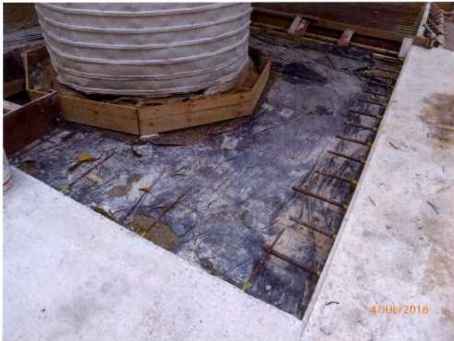
Fig. 9 The site near the planter is under renovation.
