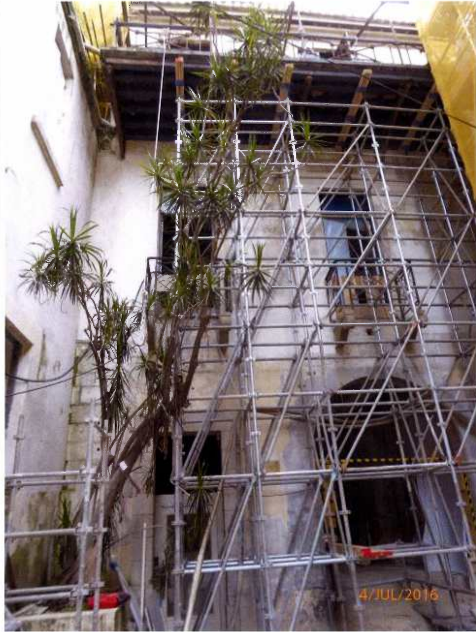
Fig. 12 Overall view of Tree 11 during inspection on 4 th July 2016.
