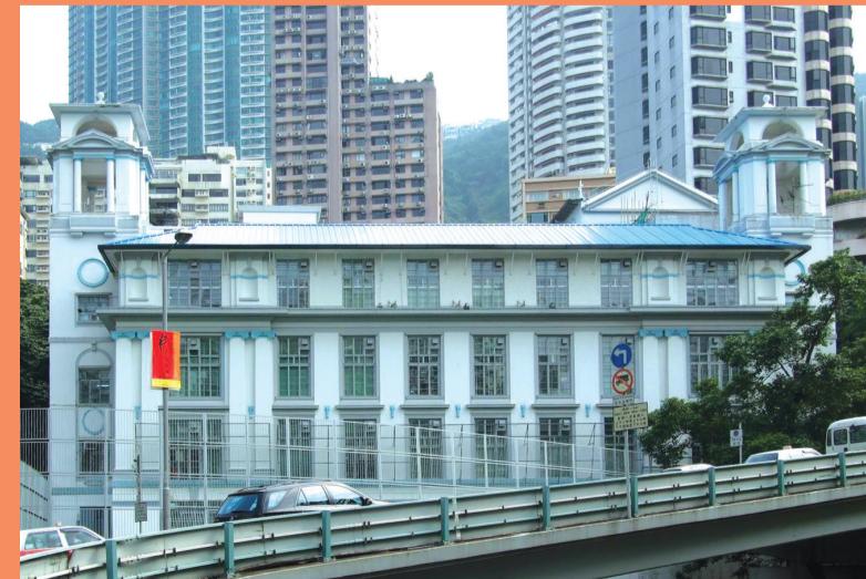
聖約瑟書院北座及西座 North and West Blocks, St. Joseph's College
