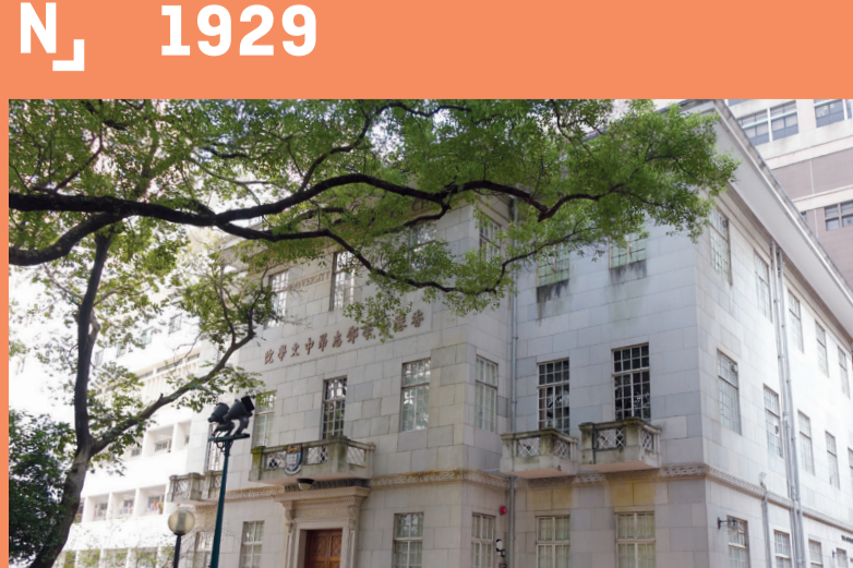
香港大學鄧志昂樓 Tang Chi Ngong Building, The University of Hong Kong
